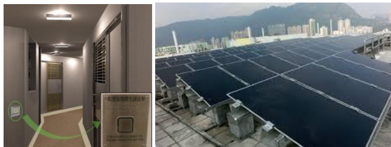
Figure 2: Two-level lighting control system (normal mode: 50 lux; triggered mode: 85 lux) (left); Roof photovoltaic system in a public housing development in 2010s (right)
