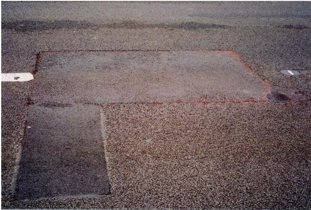
Figure 14.3 Breakdown of Sand Asphalt APL
