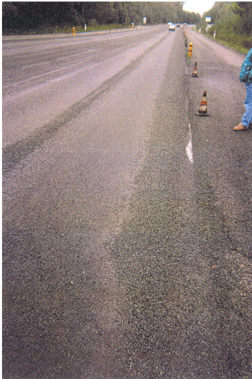
Figure 10.5 Wet Weather Failure - Slurry Surfacing with Insufficient Cohesive Strength before Thunderstorm, Damaged by Traffic
