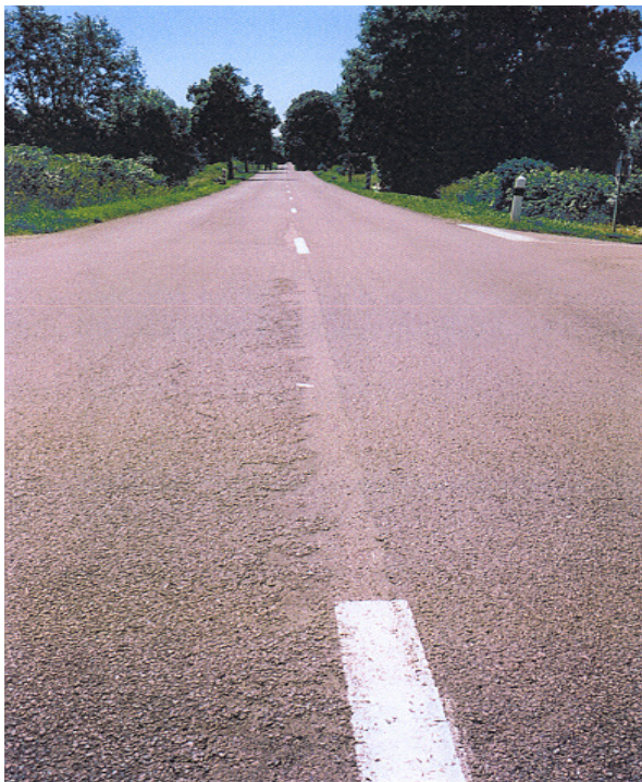
Figure 10.18 Fretting of Microsurfacing due to Mixture Problems – probably Low Binder Content
