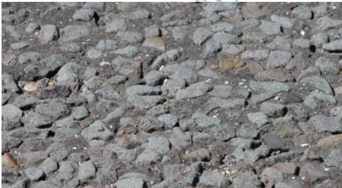
Figure 5.3 HRA after a Similar Period to Figure 5.2; however, These Chippings have not Polished, but are Worn (Lower Macro-texture) because they are a Different Stone Type (Pennant Sandstone) which Retains Micro-texture. (Photographs from a Report to the Office of the Deputy Prime Minister and the Mineral Industry Research Organisation – Capita Symonds Ltd 2004: 'The Sustainable Use of High Specification Aggregates for Skid Resistant Road Surfacing in England').
