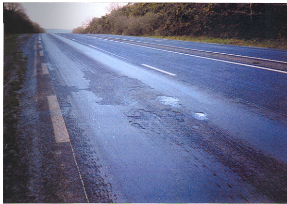
Figure 10.15 Slurry Surfacing – Mixture Problems: Fattening up and Delamination
