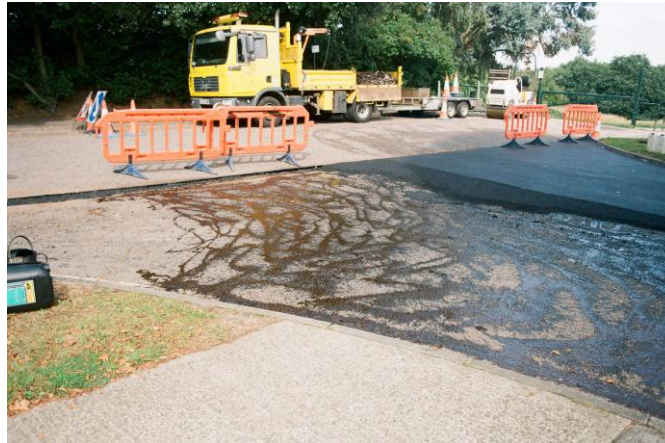
Figure 12.18 Poor Accuracy of Distribution of Tack Coat by Hand, using Watering Can
