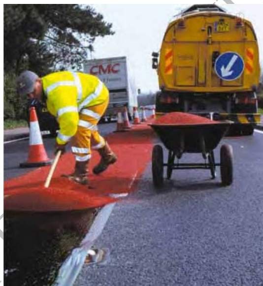
Figure 13.3 Pigment Coated Chippings Applied to Resin Binder
