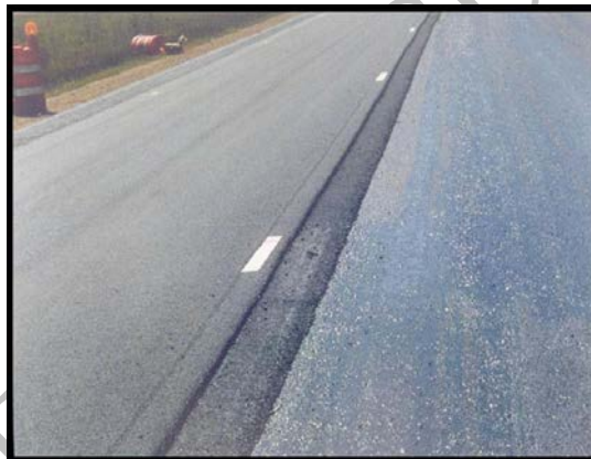
Figure 12.32 Edge Compaction to Provide an Overlap Type Joint
