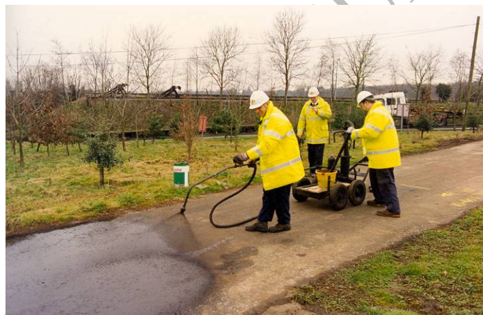
Figure 12.19 Hand Spraying Requires Expertise and after a Short Period Research has shown Rates of Spread Varying Markedly due to Tiring and Lapses in Concentration
