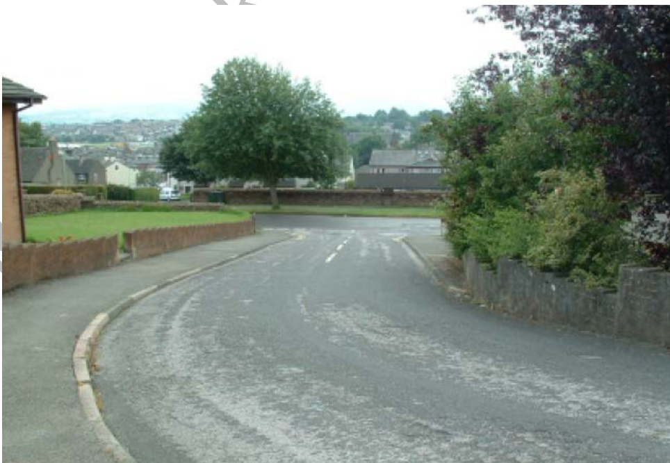
Figure 8.25 Fretting – Poor Specification – Chipping Size or Binder Rate of Spread or Adverse Conditions at the Time of Laying
