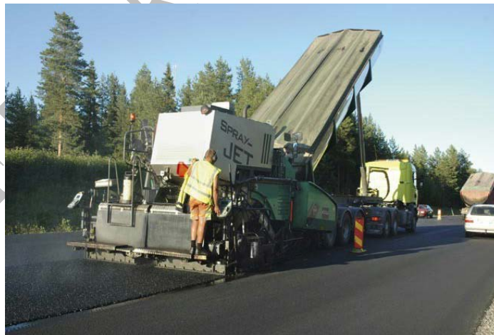
Figure 12.26 Combined Paver Bond Coat Sprayer laying TASC
