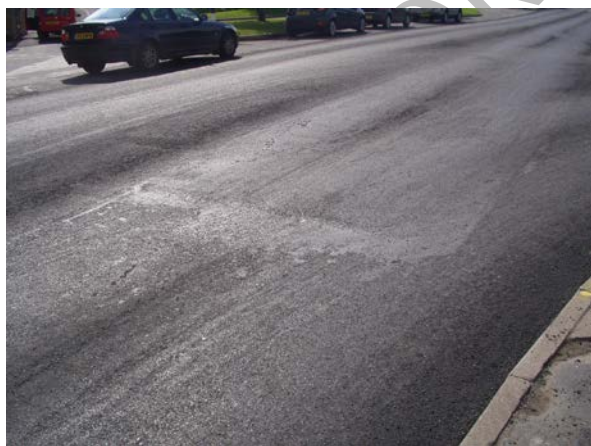
Figure 10.16 Poor Workmanship at a Joint – also Mixture Binder Rich and will Fat up
