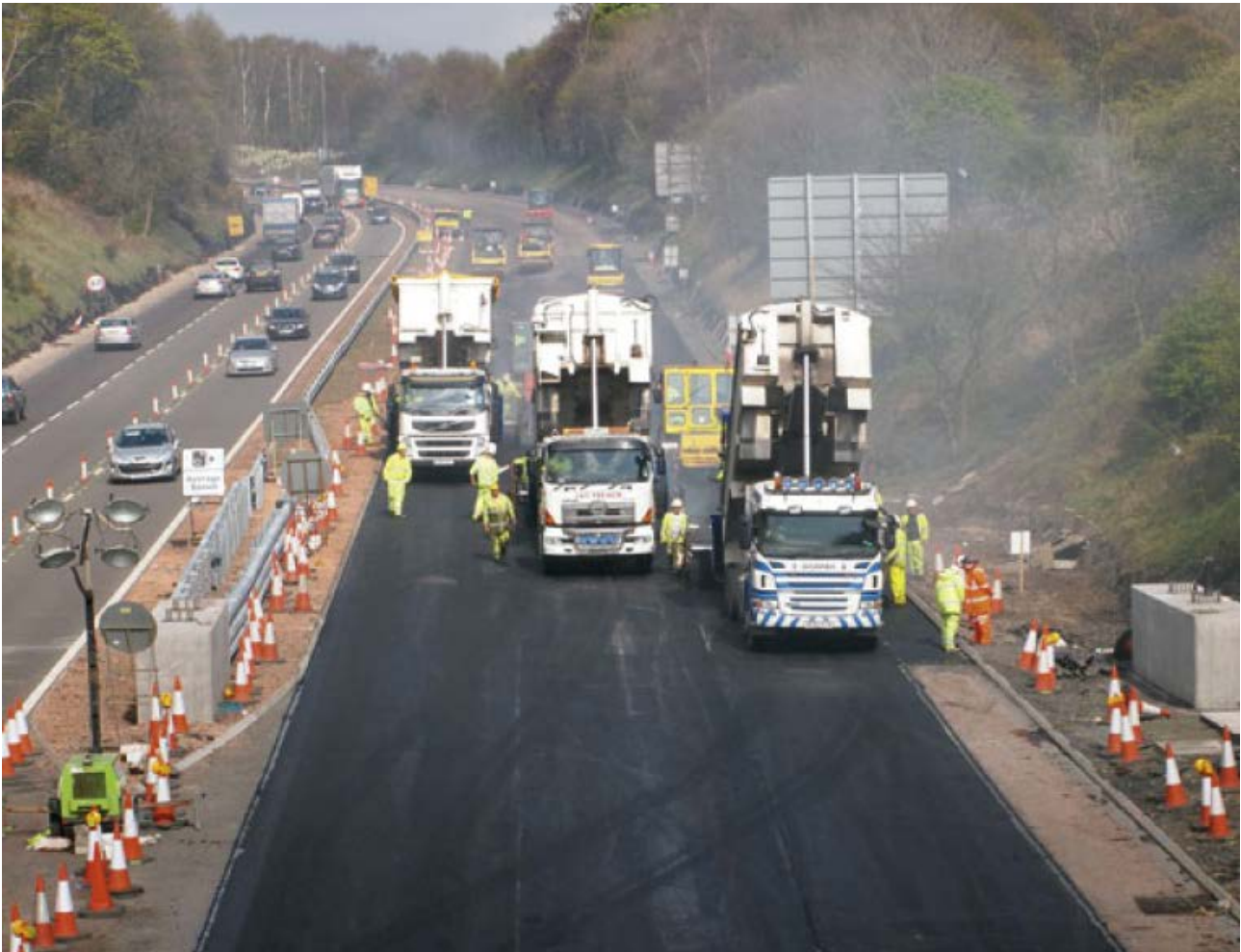
Figure 4.9 Paving Machines in Echelon
