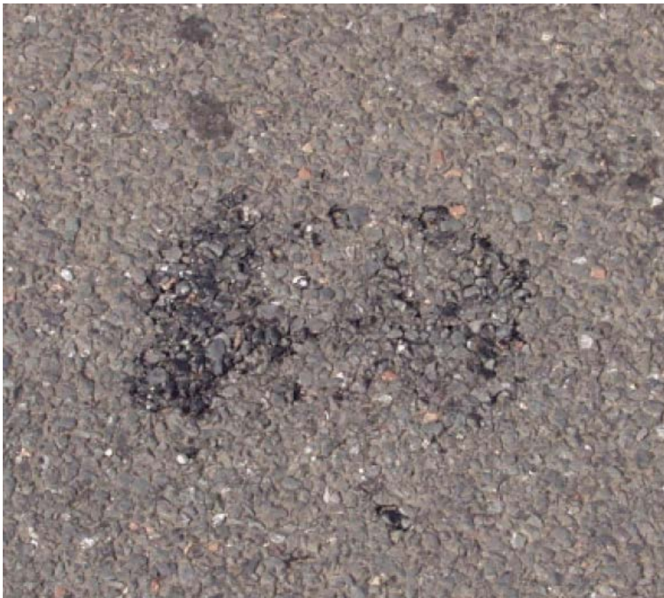
Figure 8.24 Tearing – Powered Steering – Urban Work – Alternative Design needed
