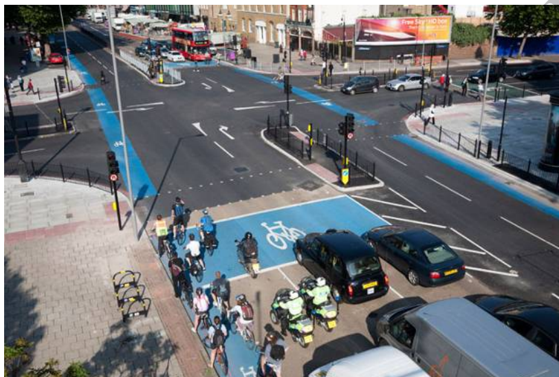
Figure 13.5 Coloured Cycle Lanes in Coloured Resin and Pigmented Chippings
