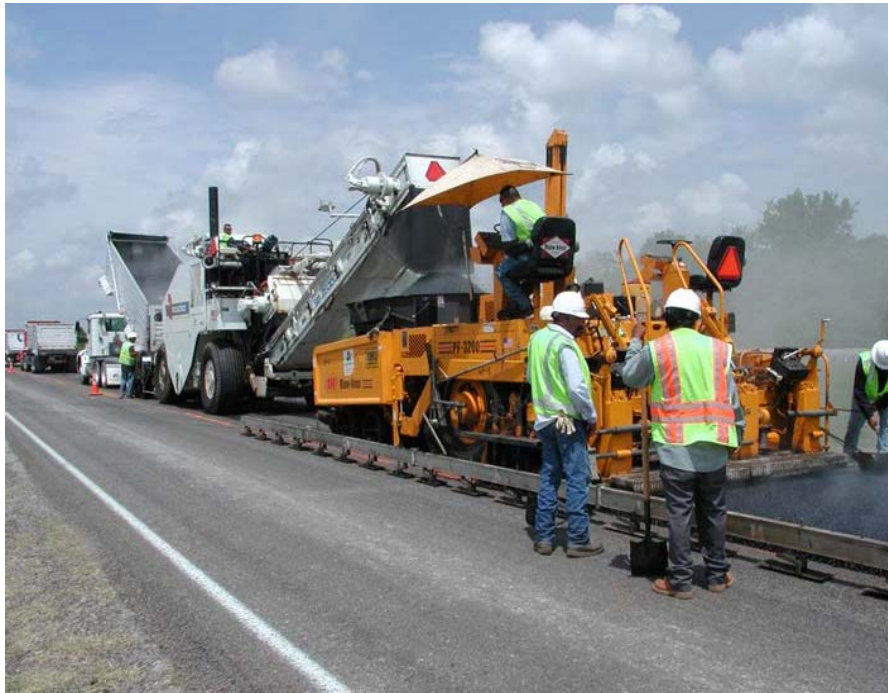
Figure 12.1 Shuttle Buggies Being Loaded without Interfering with Paving Operations
