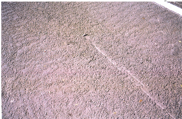
Figure 10.23 Score Mark caused by Aggregate Contaminant (May also be Lumps of Cured Material)
