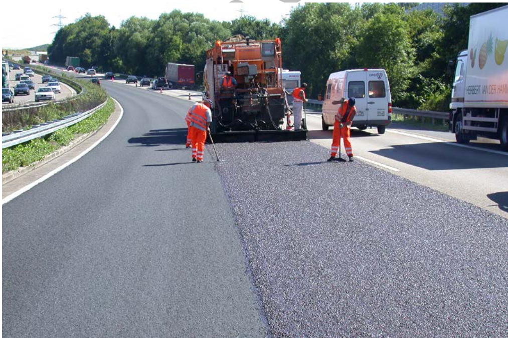
Figure 10.3 Microsurfacing Second Layer - Motorway Work in Europe
