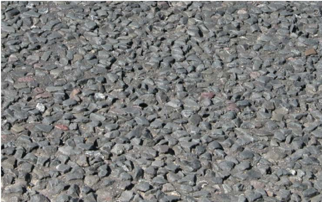
Figure 5.2 HRA after 15 years' Service – Note Polishing of the Chippings, but Good Macro-texture Retention
