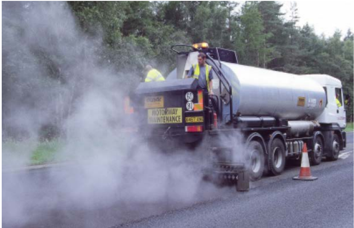
Figure 8.3 Computerised Sprayer – Steam from a Polymer Modified Emulsion Sprayed at 85 °C
