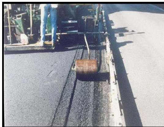
Figure 12.33 Edge Compactor Attached to the Paver
