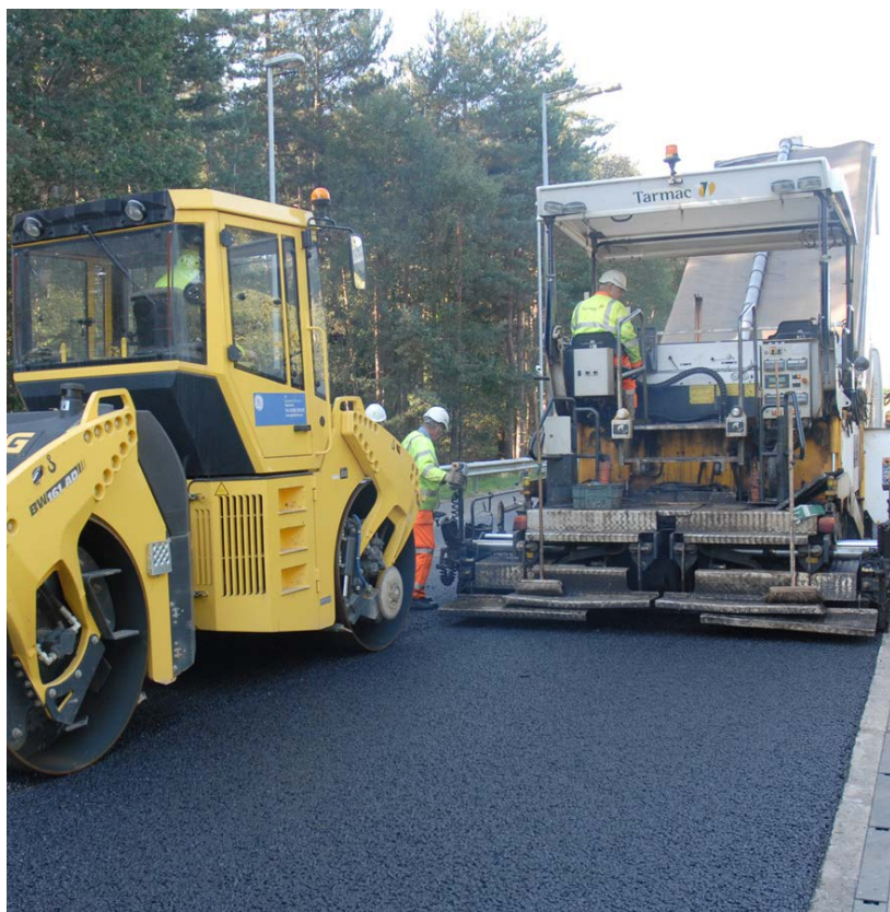
Figure 4.7 TASC being Laid on a Binder Course
