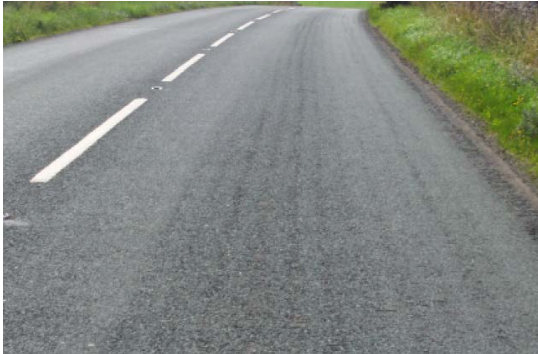
Figure 8.26 Streaking – Spraybar Problems – Binder Temperature or Pressure Too Low, Blocked Filter or Jets, Spraybar Height Variations, or Pump Problems.
