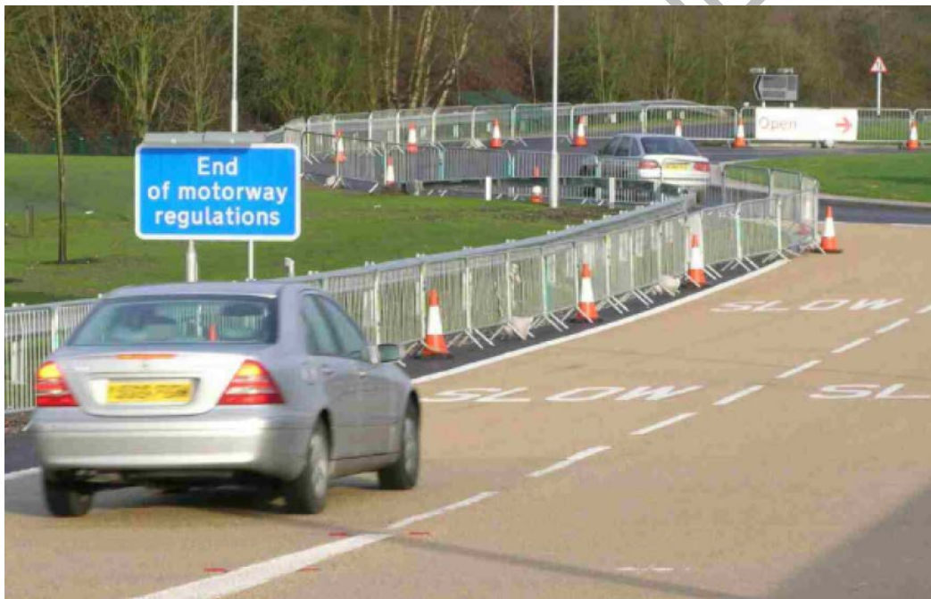
Figure 9.1 HFS – Sprayed Epoxy Resin System using Chinese Calcined Bauxite
