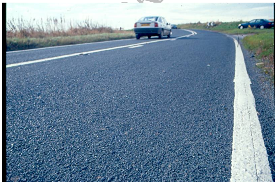
Figure 4.3 Innovative Ultra-thin Treatment (IUT) Low Tyre/Noise Generation Surface Course, with Three Chipping Layers (14, 10 and 6mm) and Two Polymer Modified Binder Layers (One as a Grout)
