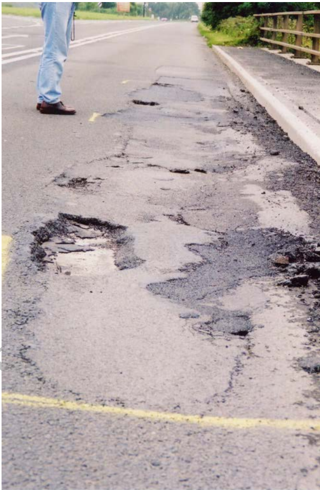
Figure 14.1 Premature Failure of sub-120mm Thick Bridge Deck Surfacing
