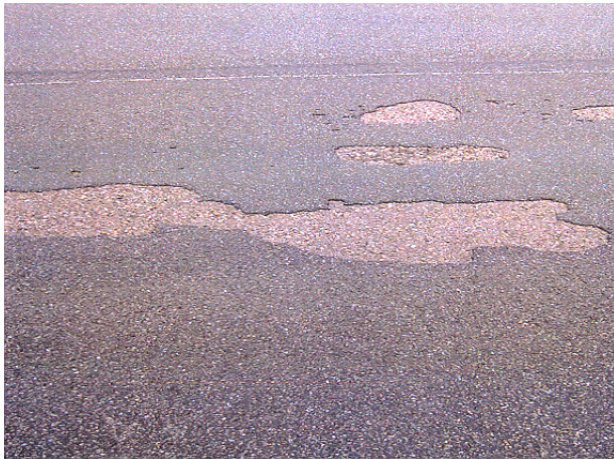
Figure 10.17 Delamination – no Bond Coat
