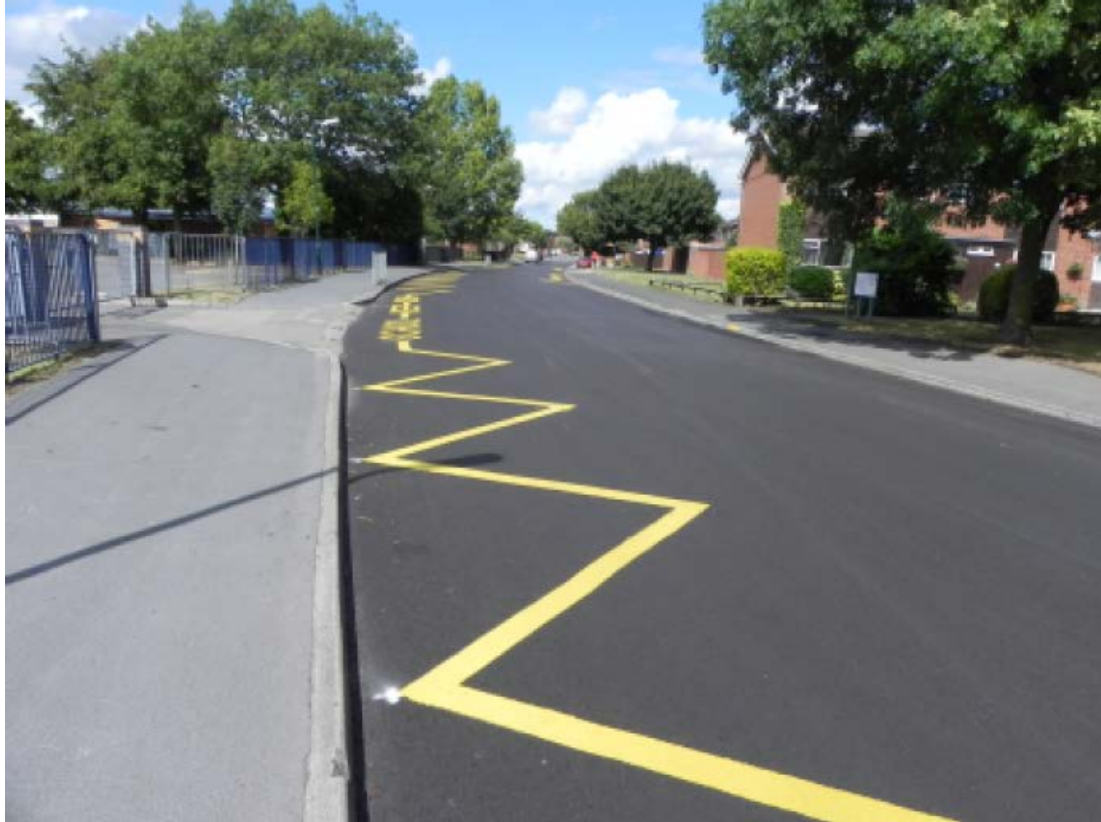
Figure 5.4 55/10 HRA – Sufficient Macro-texture for Low Speed Roads
