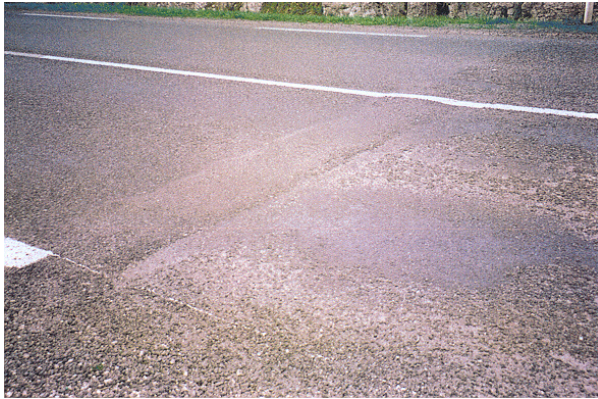
Figure 10.22 Transverse Bump and Some Localised Loss of Aggregate
