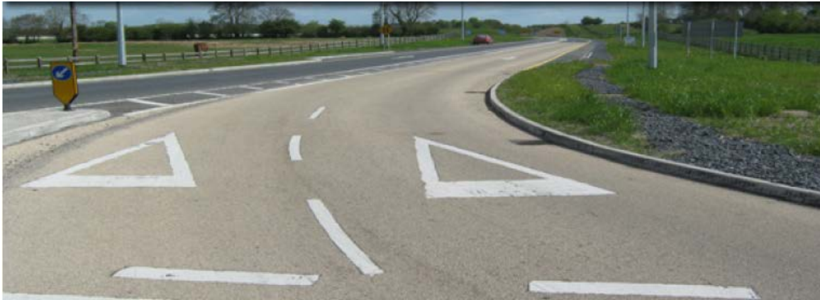
Figure 9.2 HFS Cold Applied Resin System
