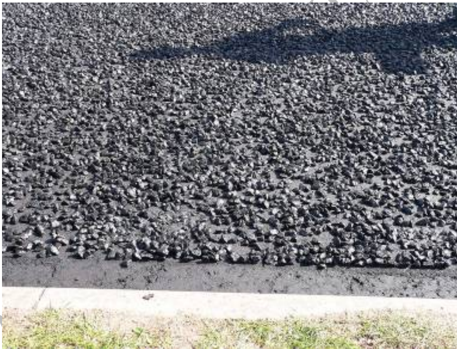
Figure 12.4 HRA Surface Course Application of Pre-coated Chippings Prior to Rolling
