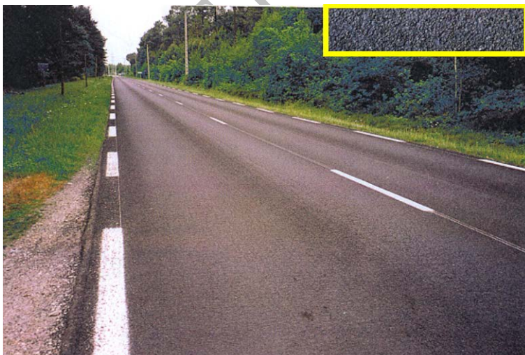
Figure 10.26 Microsurfacing on a Rural Road with Adequate Macro-texture – see Insert
