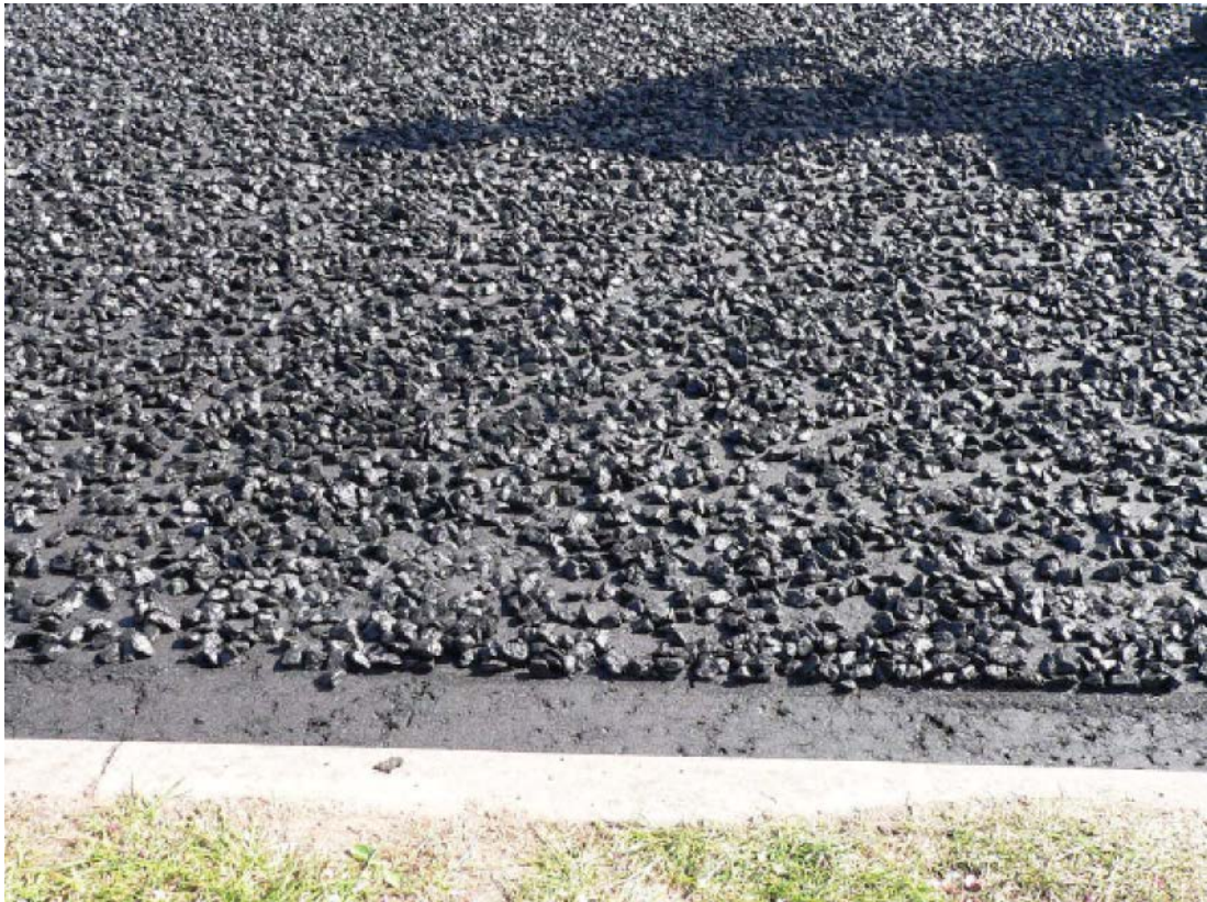
Figure 5.6 Applied Chippings before Rolling – Note Chippings not Laid at the Kerb Edge
