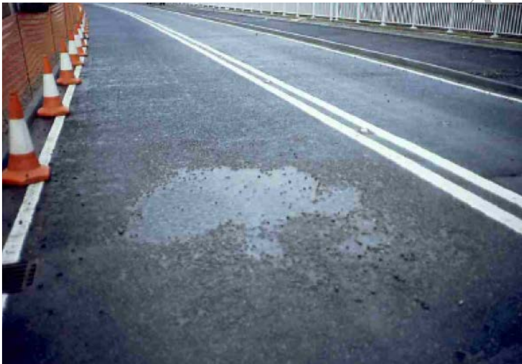
Figure 12.5 Loss of Pre-Coated Chippings due to Poor Weather Conditions
