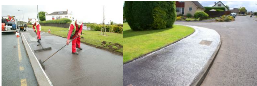
Figure 10.13 Footway Maintenance Slurry Surfacing – Street Furniture and Kerbs are Protected with Tape
