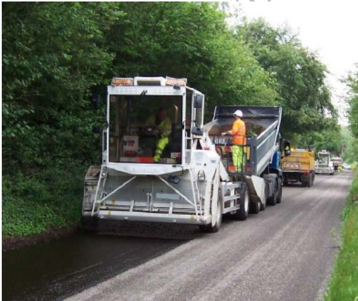
Figure 8.1 Rural Road 10 mm Racked-in with 6 mm Surface Dressing Intermediate Polymer Modified Binder
