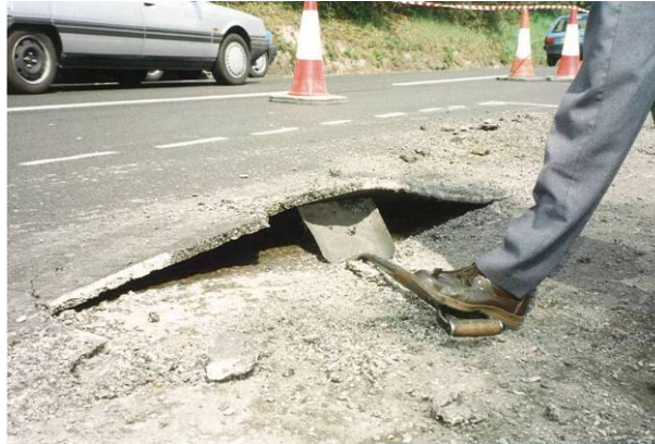
Figure 12.14 Lack of Bond to Substrate can have Catastrophic Results
