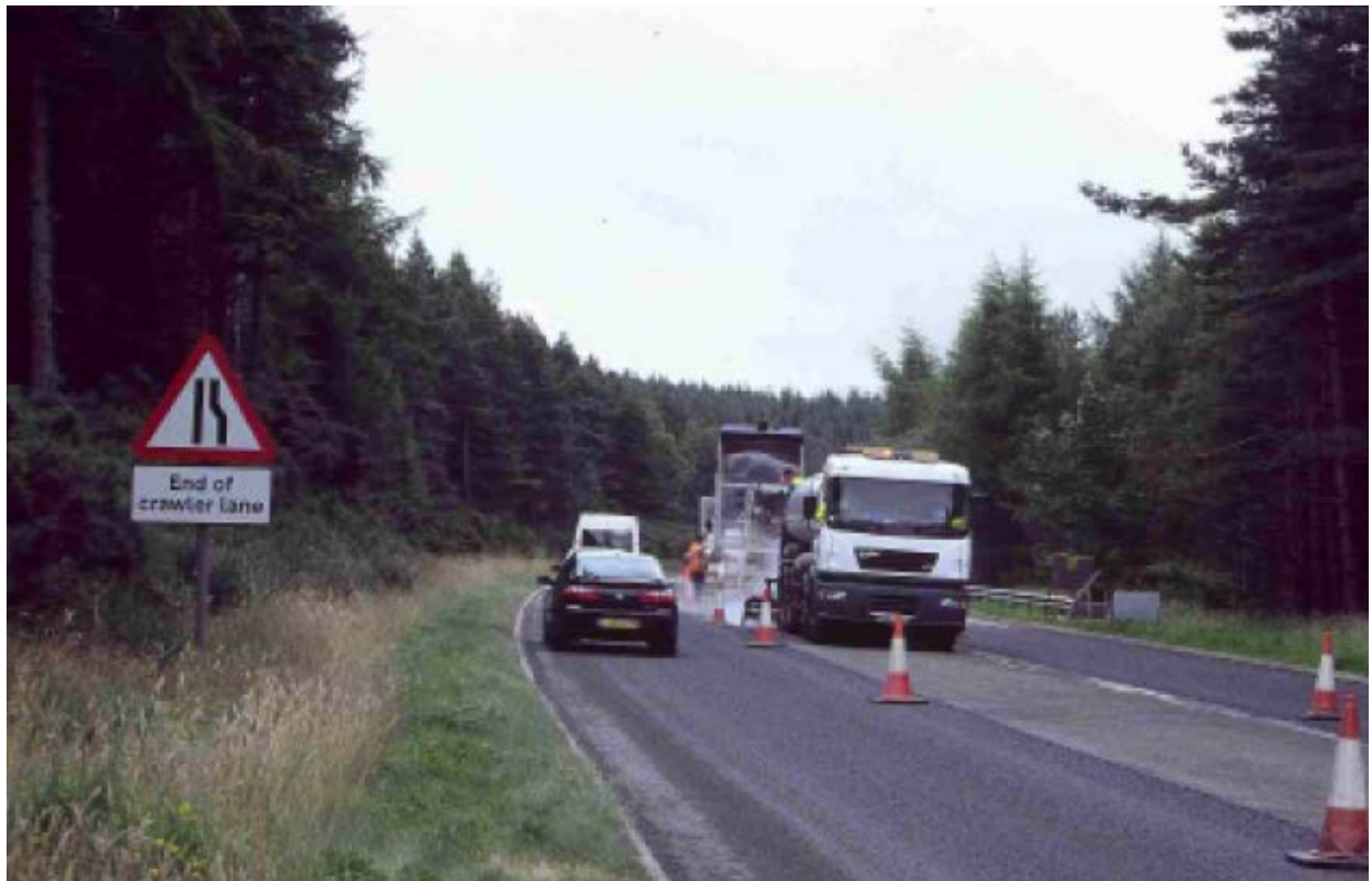
Figure 8.4 14mm Racked-in with 6mm Surface Dressing using Premium Polymer Modified Emulsion
