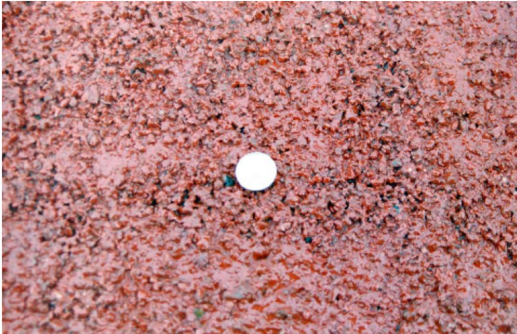
Figure 9.7 Red Pigmented Resin Screeded System with Grey Guayanan Calcined Bauxite
