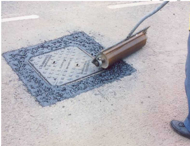
Figure 13.12 Final Application of Pre-coated Chippings
