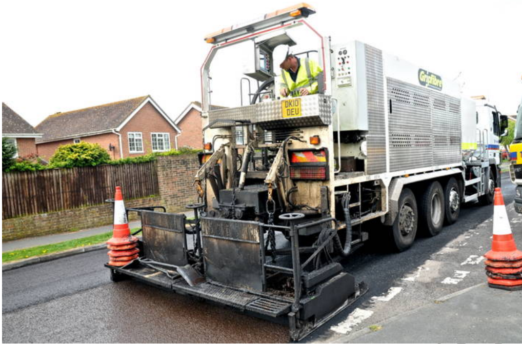
Figure 10.4 Microsurfacing Surface Layer over Previously Laid Coarser Base Layer – Urban Road
