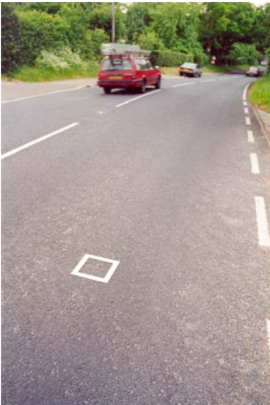
Evidence of Fretting - Low Percentage Loss Measured (2%) after Five Years, therefore Satisfactory
