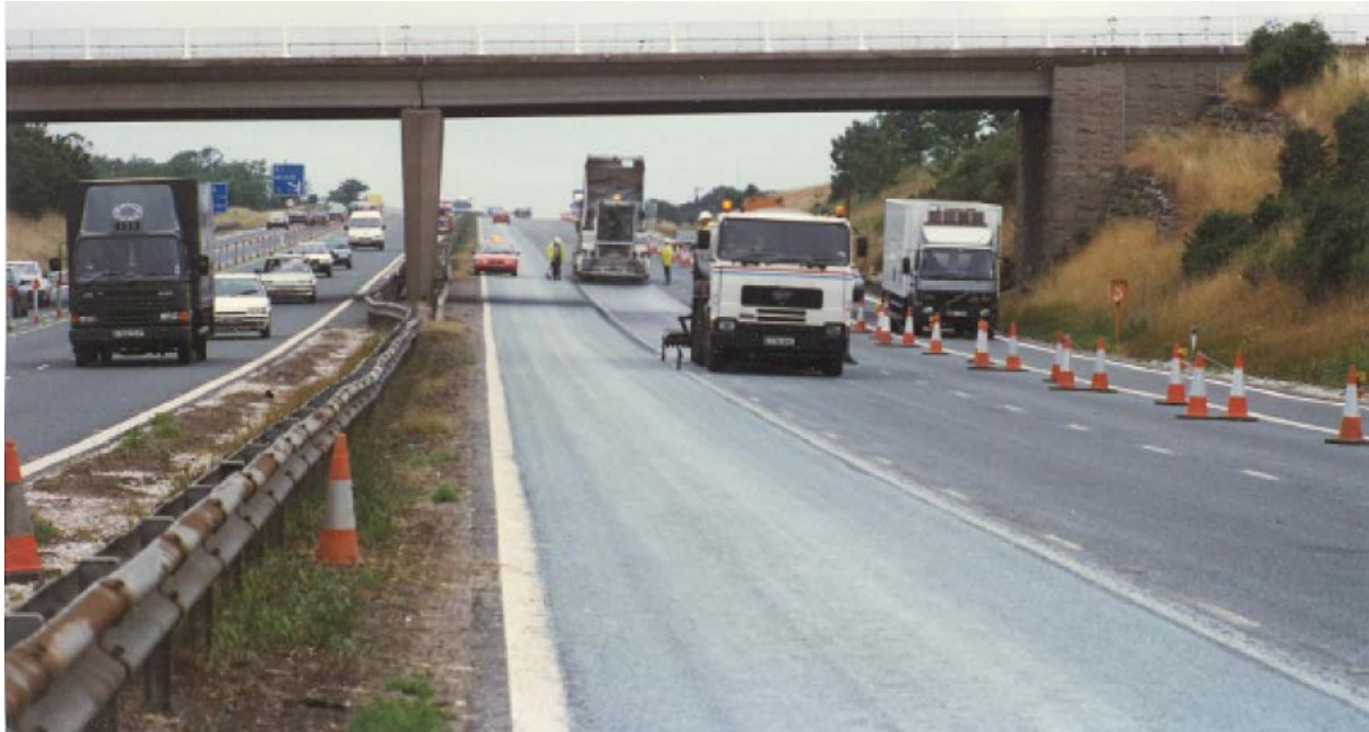
Figure 8.2 High-Speed Heavily Trafficked Road: Proprietary Surface Dressing (IUT) Comprising 14mm Primary Followed by 6mm Chipping Layer using Two Layers of a Premium Polymer Modified Bituminous Emulsion Binder
