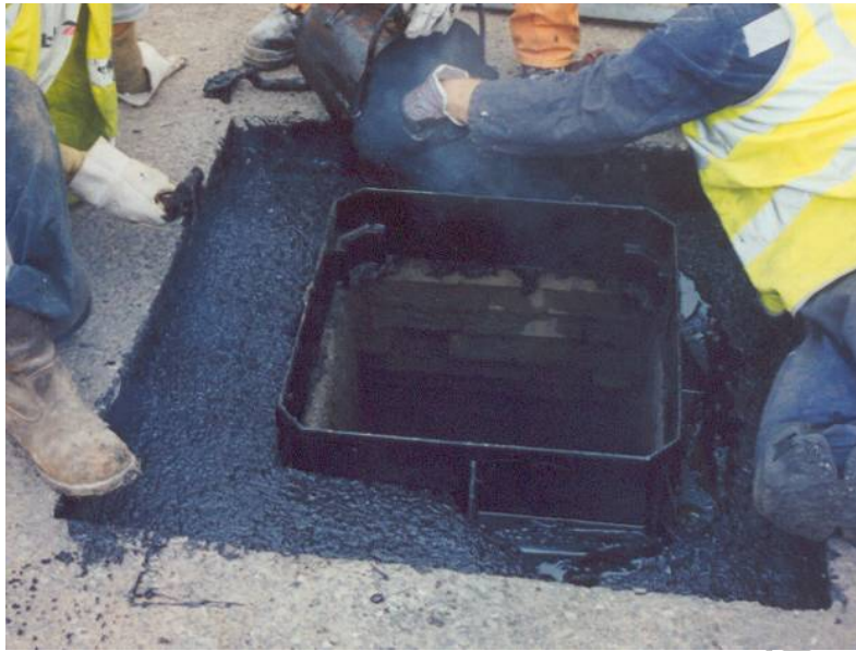
Figure 13.11 Seating the Frame and Sealing
