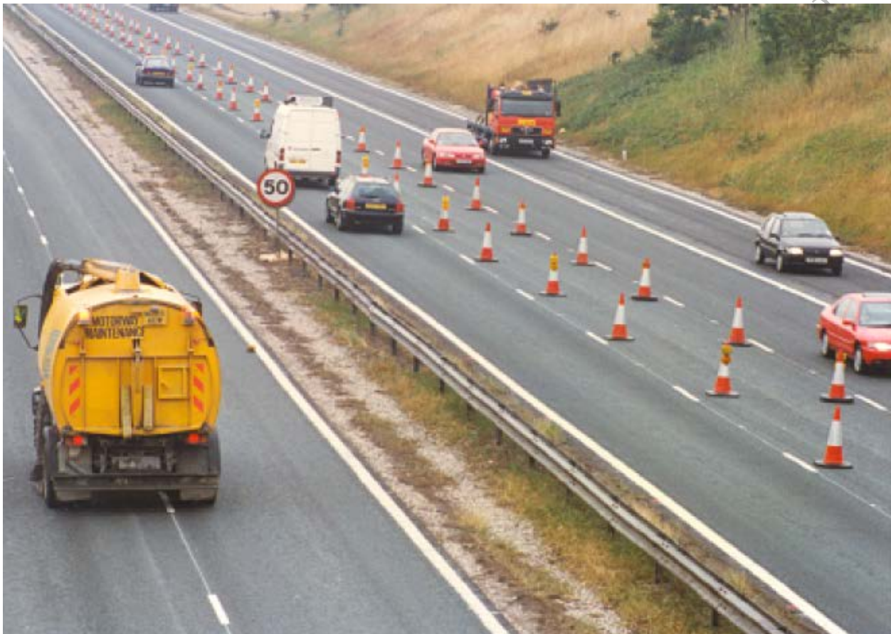
Figure 8.6 Suction Sweepers are Used for IUTs to Remove any Loose Chippings from the Primary Layer during the Installation and then from the Final Surface Dressing Layer
