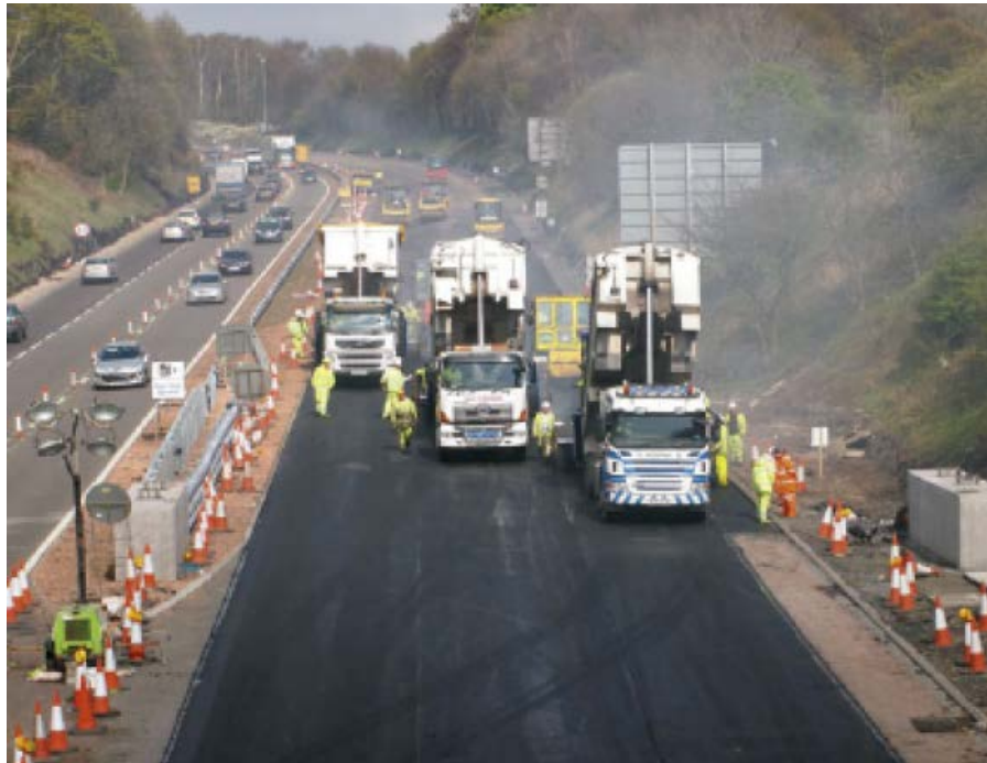
Figure 12.12 Three Paving Teams in Echelon Laying Stone Mastic Asphalt
