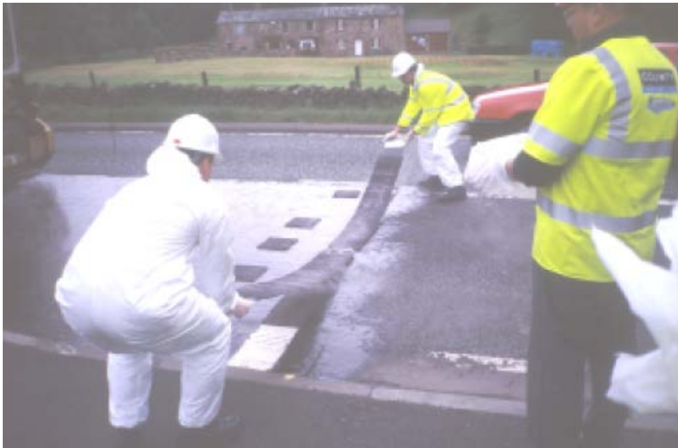
Figure 8.15 Transverse Distribution of Binder Test
