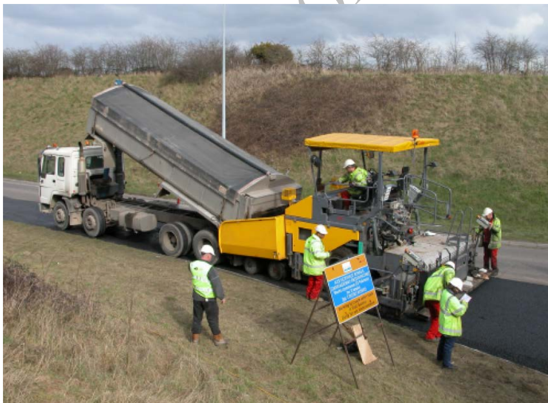
Figure 4.8 TASC Polymer Modified 25mm Overlay over Bond Coat
