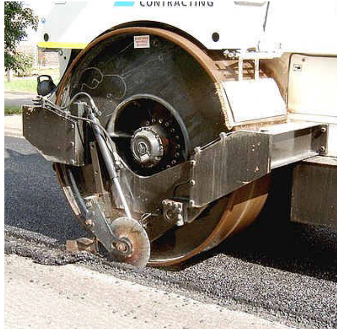
Figure 12.28 Cutting Back Thin Asphalt Overlay Preparing a Vertical Joint
