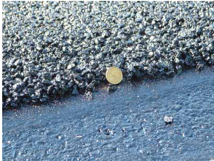
Figure 12.22 Asphalt Ultra-thin Layer (AUTL) Being Laid on Class 5 Bond Coat that has Broken
