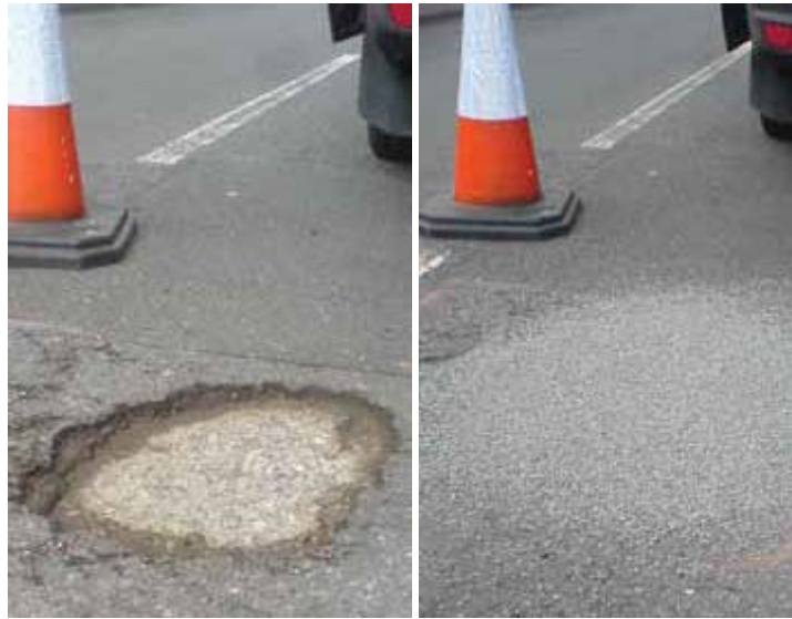
Figure 13.6 Emergency Patching Materials; note Application of Chippings on the Resin System
