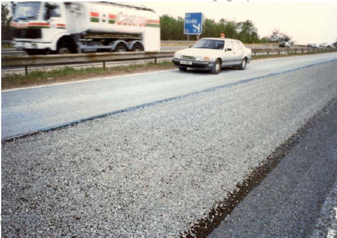
Figure 8.9 Primary 14mm layer; Note Two Wet Edges and Binder Visible through the Chippings (Windows)
