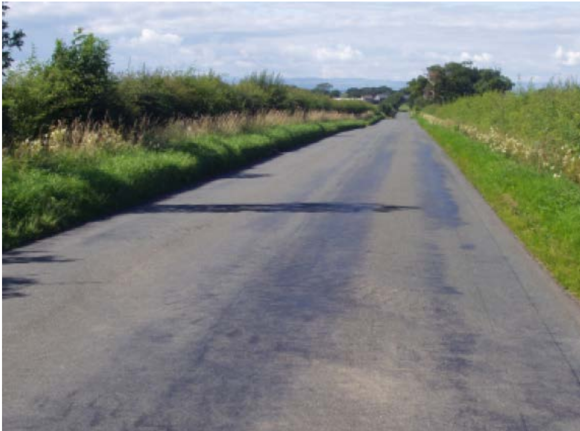
Figure 8.20 Bleeding and Tracking
