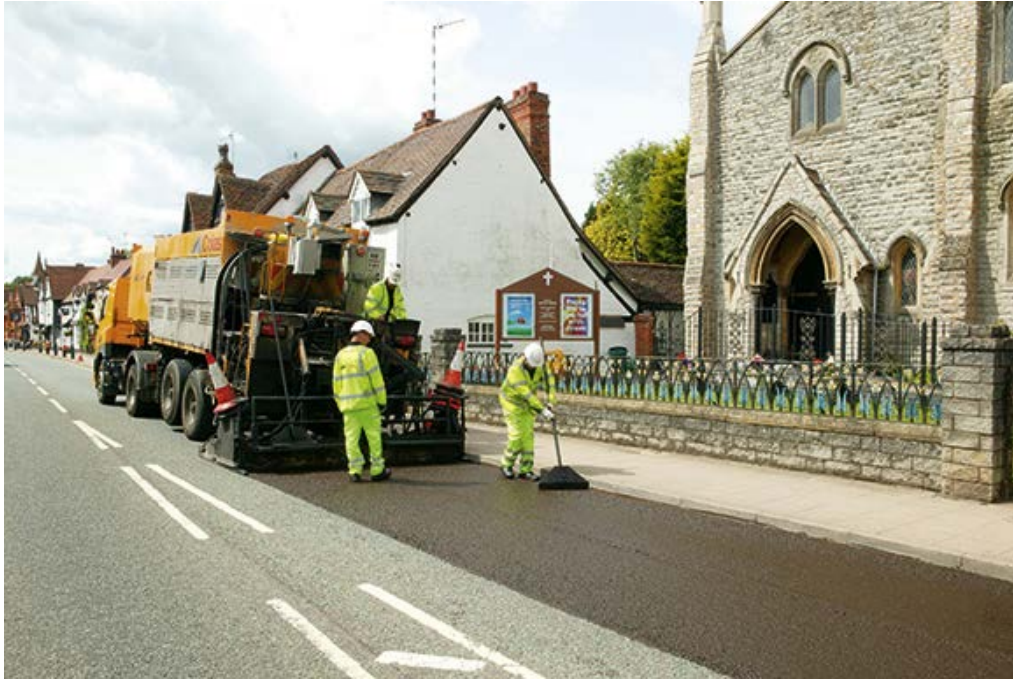
Figure 10.2 Slurry Surfacing - Urban Road
