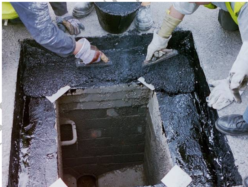
Figure 13.10 Polymer Modified Mastic for Manhole Repair, note the Hot Bond Coat
