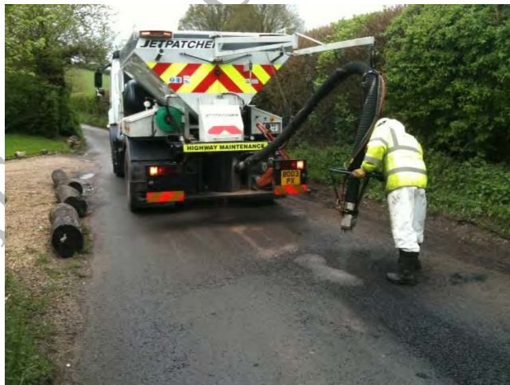
Figure 13.7 Spray Injection Patching
