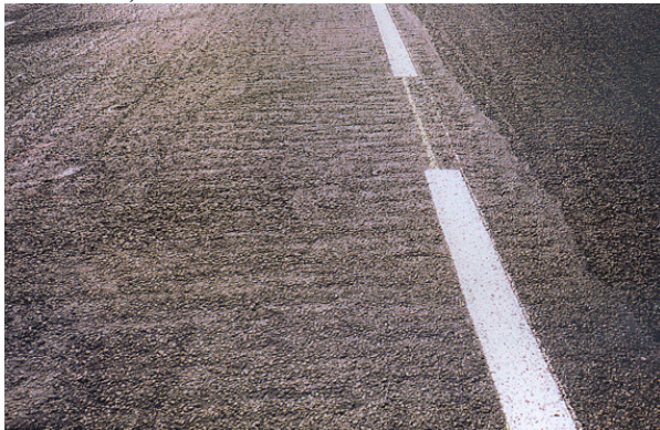
Figure 10.20 Unacceptable Corrugation of Laid Material
