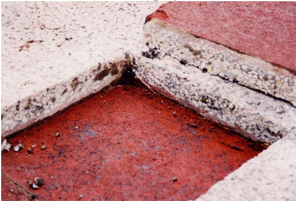
Figure 14.2 Moisture Trapped in Thin Surfacing
