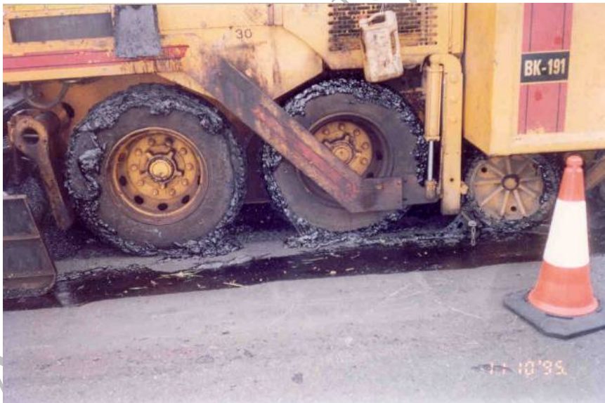
Figure 12.23 Bond Coat Being Picked up by Warm Paver Tyres.
