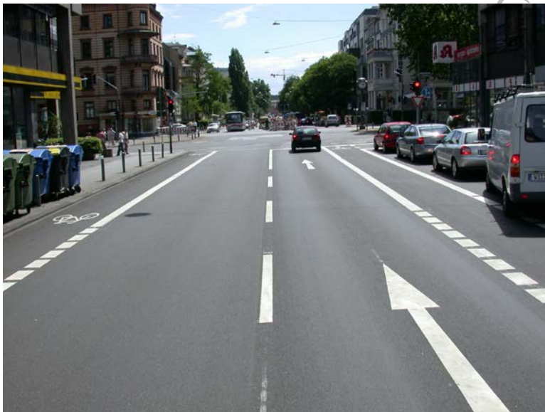
Figure 10.9 Microsurfacing Used for an Urban Braking Area
