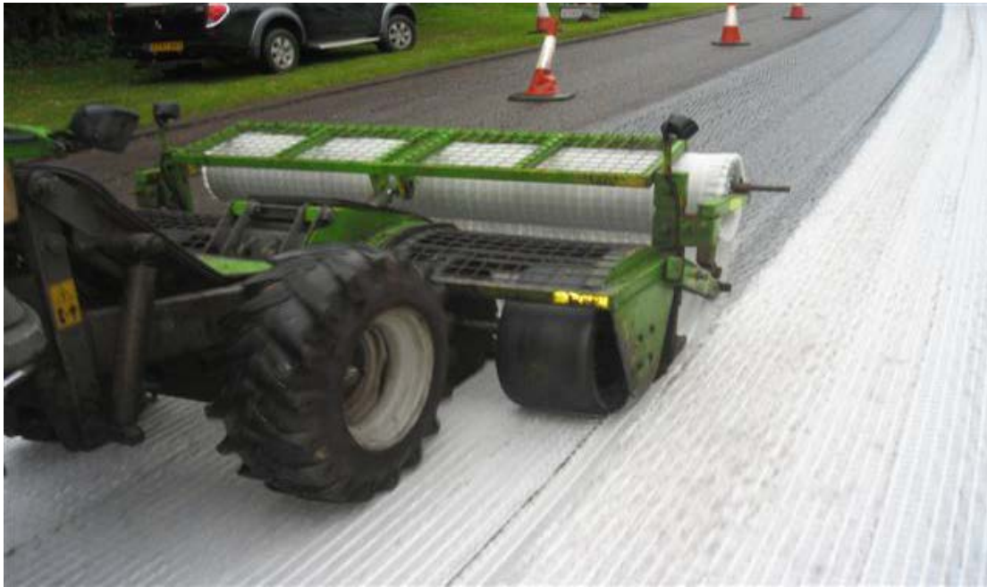
Figure 11.7 Purpose Built Applicator for Installing Geosynthetics
