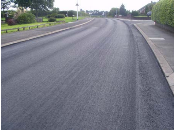
Figure 10.24 Slight Mixture and Segregation Problems and Spreader Box needs Maintenance. This Appearance is not Regarded as a Defect; the Skid Resistance will be Good and the Surfacing is Complete. Traffic Wear will Improve the Appearance with Time.
