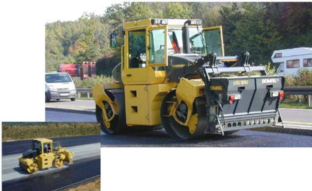
Figure 6.3 Gritting Application on SMA Surface Course (Source: Gartner, 2012)
