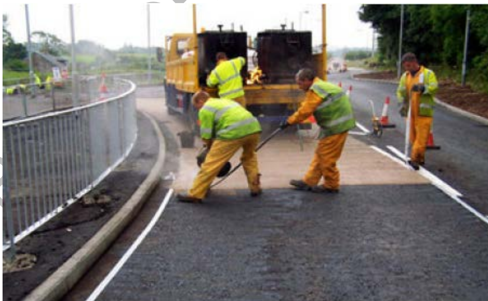
Figure 9.3 Hot Applied Screeded Mixed Resin System
