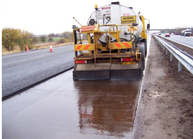
Figure 12.20 Example of Even Application of Bond Coat
