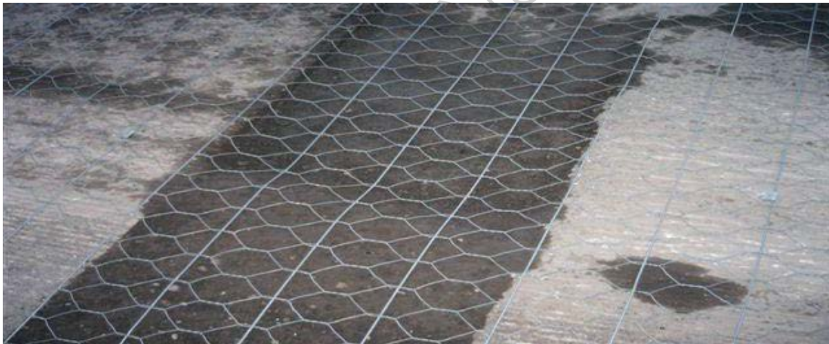
Figure 11.1: Steel Mesh (typically Galvanised Steel Wire, Double Twisted to form a Mesh with Reinforcing Bars at Intervals).
