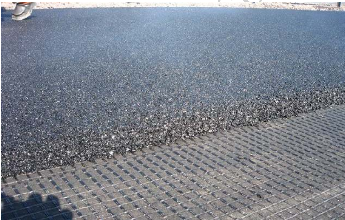
Figure 11.8 Combination Grid with Asphalt Overlay
