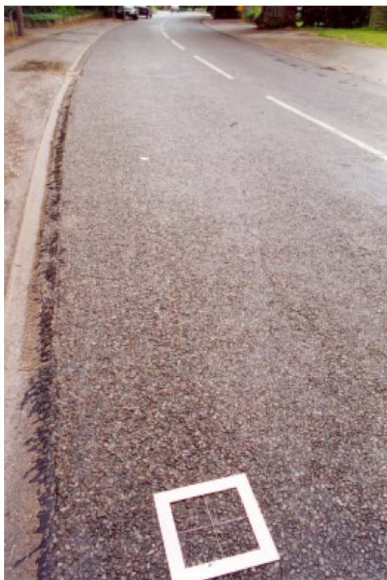
Inverted Double Dressing Age 15 years, Surface Comprising 14mm Chippings (No Loss)
