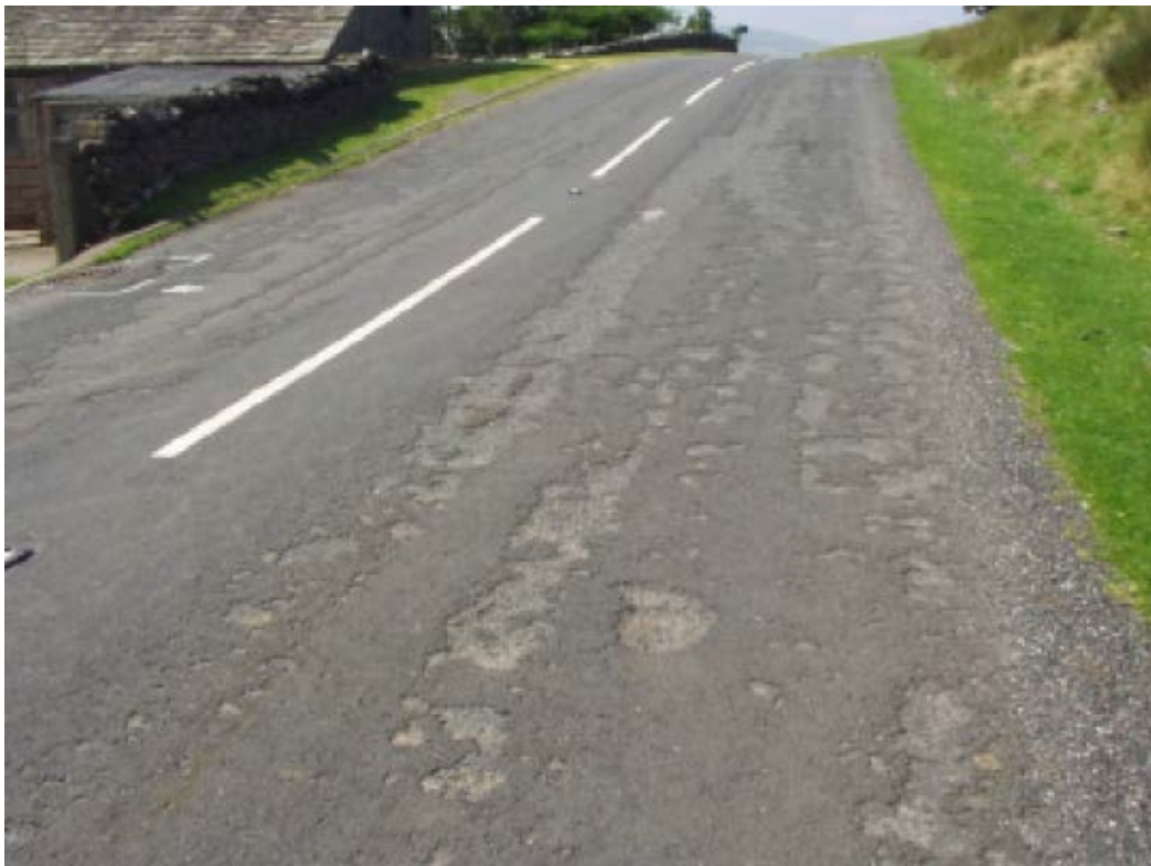
Figure 8.22 Scabbing – Poor Site Preparation – Surface Contaminants not Removed
