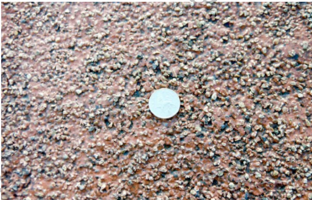
Figure 9.8 Red Pigmented Resin Screeded System with Grey Guayanan Calcined Bauxite after a Few Years Wear at a Pedestrian Crossing – Note Loss of Pigmentation
