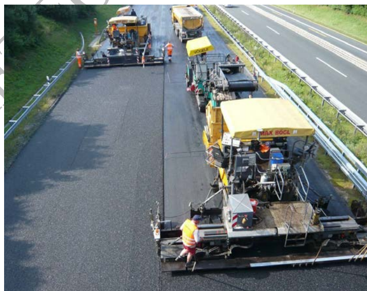
Figure 12.11 The Second of Two Paving Machines, in Echelon, Laying the Second Rip of a TASC so that Both Rips can be Compacted Simultaneously Whilst Hot
