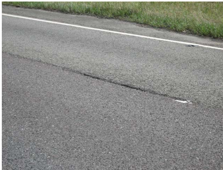
Figure 12.15 Road Markings may Encourage Fretting Beneath more Open-textured Materials
