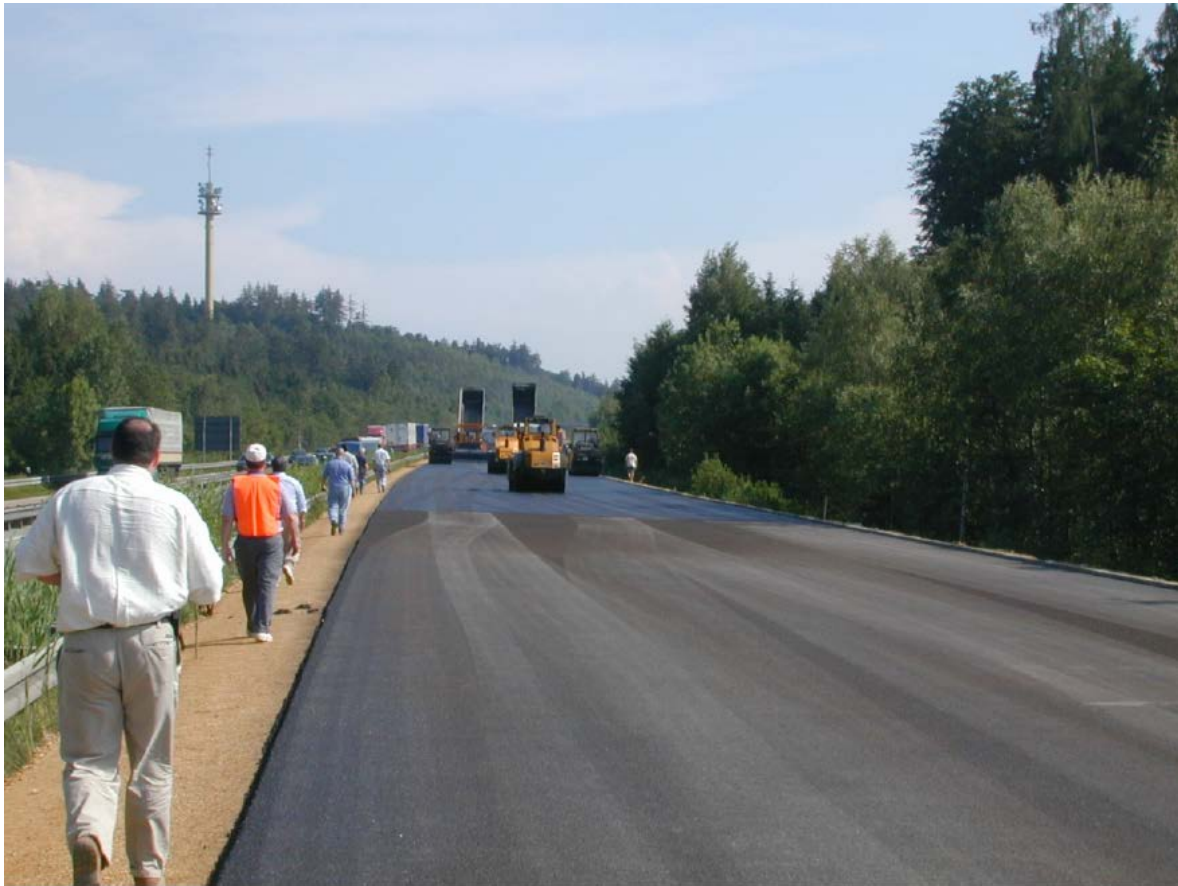
Figure 6.4 Appearance of SMA Surface Course Before and After Gritting (Source: Prowell, 2009)
