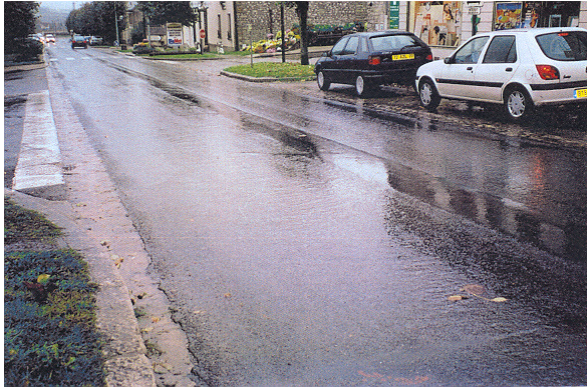
Figure 10.19 Poor Overlap at Joint – More Pronounced when Road is Wet
