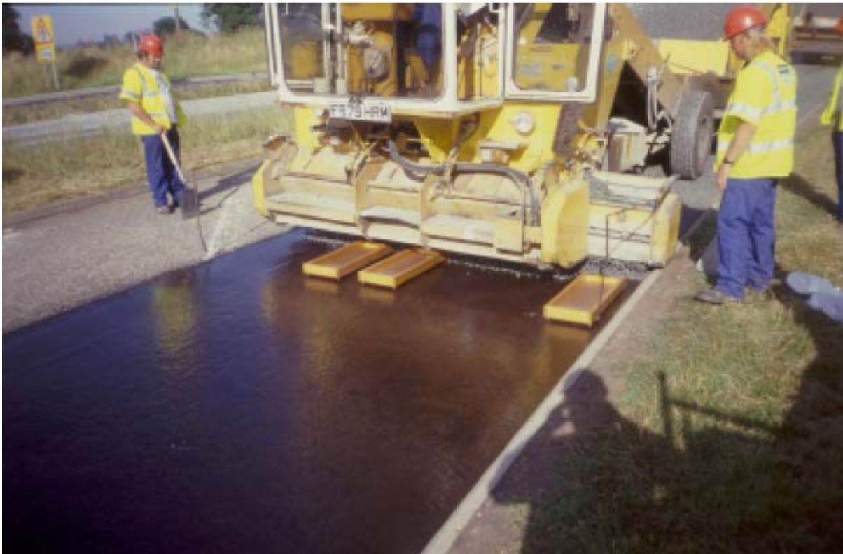
Figure 8.17 Checking Rate of Spread of Chippings BS EN 12272-1
