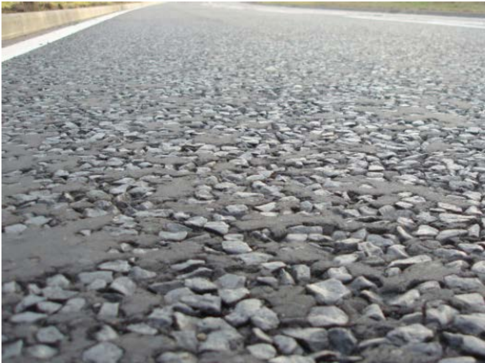
Figure 5.1 Newly Laid Chipped HRA Surface Course
