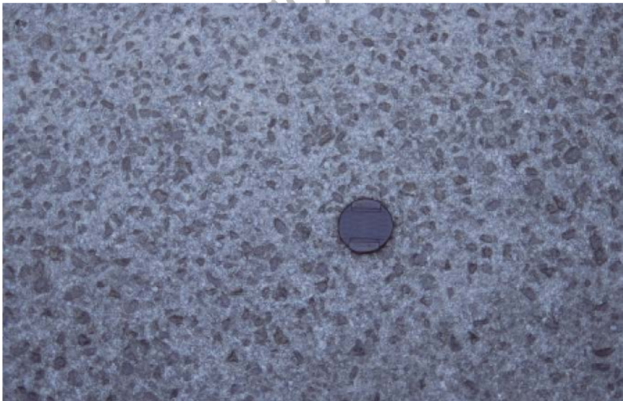
Figure 8.11 Excess 6mm Chippings Removed, Suction Swept – Carriageway Open to Traffic, 14mm Chippings Locked in by the 6mm Final Layer. No Loose Chippings to Damage Vehicles even at High Speed.
