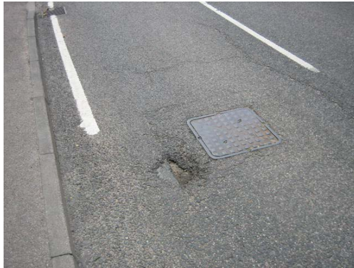
Figure 12.16 Defects around Ironwork
