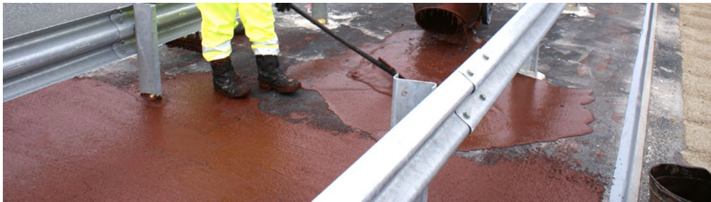
Figure 10.10 Coloured Slurry Surfacing Used for a Central Reserve
