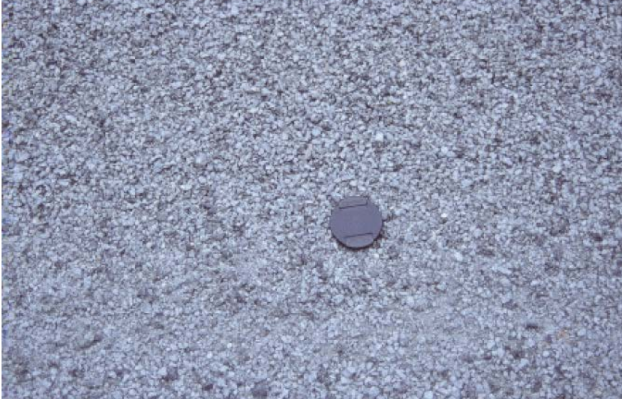
Figure 8.10 Initial Excess of 6mm Chippings from the Final Layer in a Double Surface Dressing
