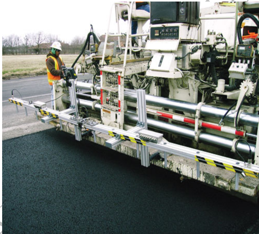
Figure 12.35 Infra-red Detectors Attached to Paver with Monitor Mounted Above
