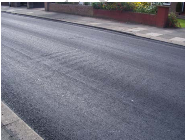
Figure 10.21 Slight Corrugation Visible is not a Defect – Appearance will Improve with Traffic Wear
