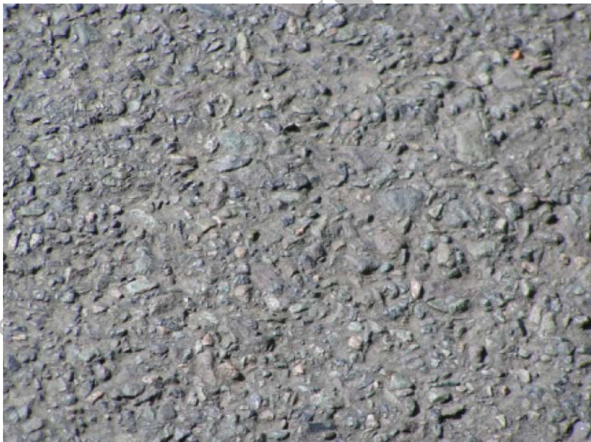
Figure 8.13 Long Life Example: 24 years A 452 - Premium Emulsion 14mm and 6mm Chippings
