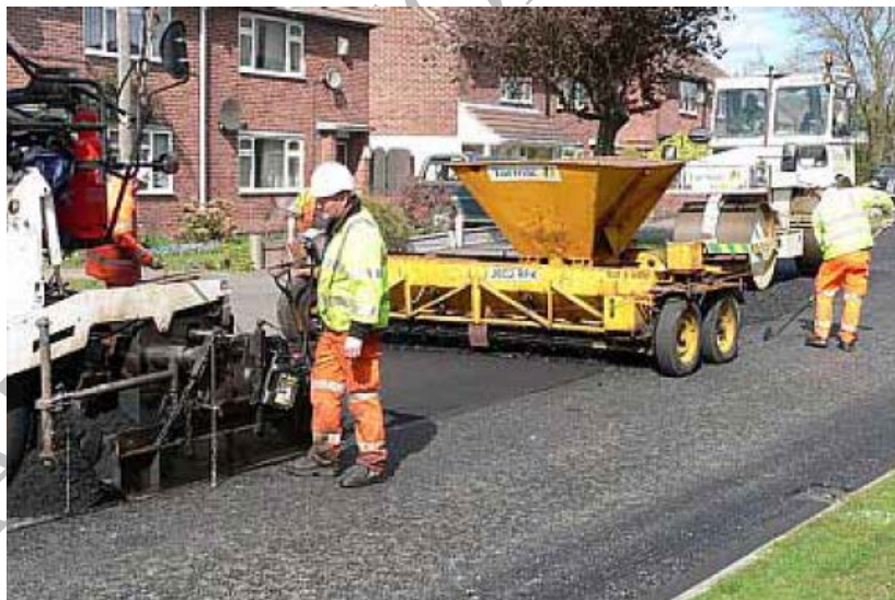
Figure 12.7 Chipping Machine Straddling the Paved HRA Surface Course
