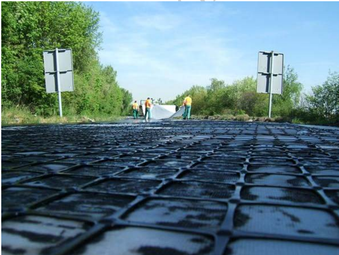
Figure 11.3: Polymer Grids (typically Punched and Stretched Polypropylene or Knitted/woven Polyester).
