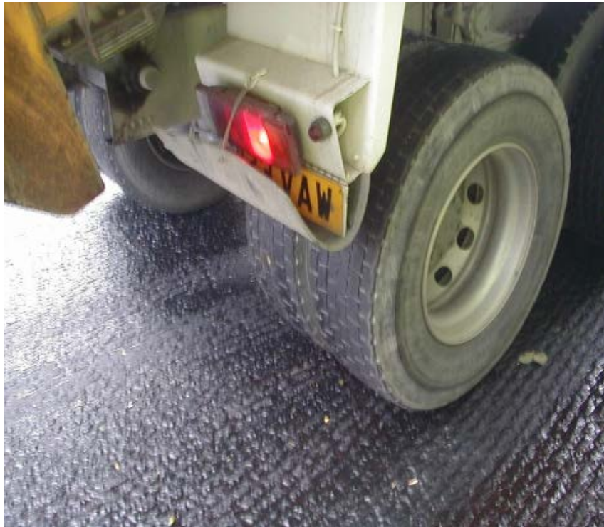
Figure 12.24 Non-sticky Bond Coat, not Being Picked up on the Asphalt Delivery Tyres
