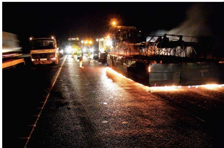
Figure 12.9 Pre-heating Cold and Wet Asphalt Substrate before Overlaying with a Thin Asphalt Layer.
