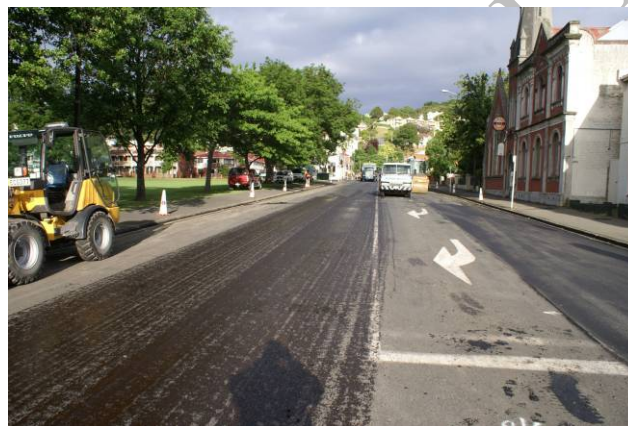
Figure 12.21 Example of Poor Transverse Distribution of Bond Coat
