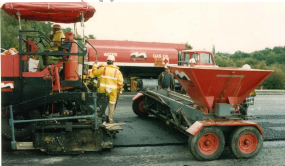
Figure 5.5 Application of Pre-Coated Chippings
