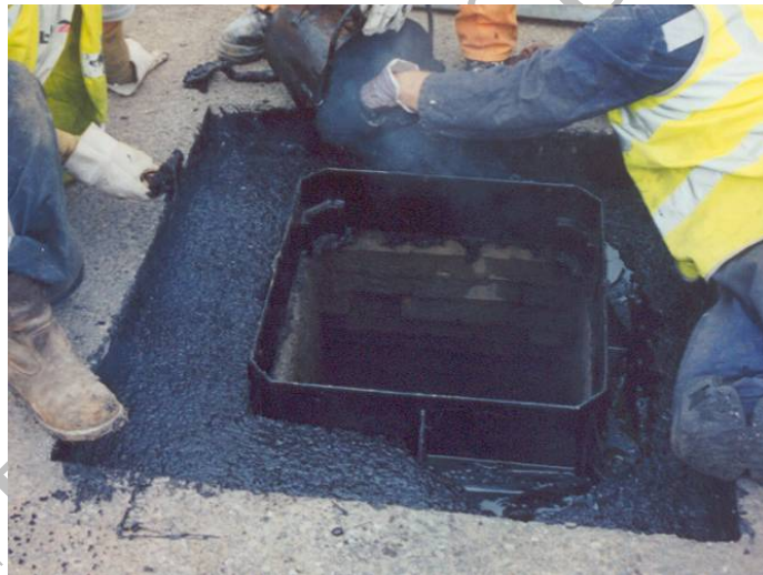
Figure 12.17 Polymer Modified Mastic Asphalt used for Bedding and Sealing Round Ironwork
