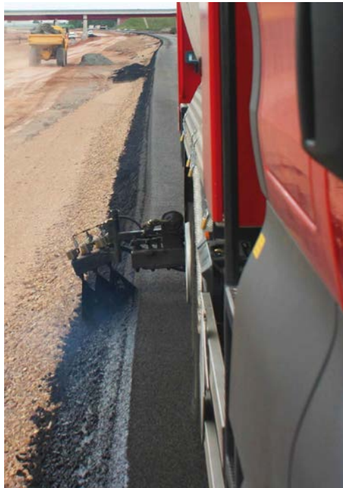
Figure 12.31 Side Jet Spray on Modified Bond Coat Sprayer to Seal Vertical Joints and Edges
