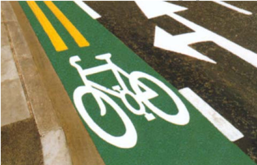
Figure 9.4 Cycle Lane – Green Resin System
