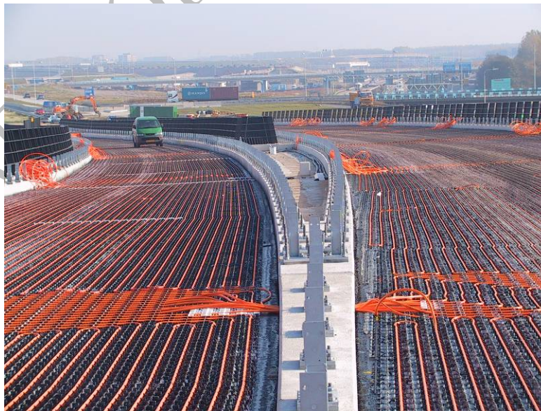
Figure 13.8 Pipes Embedded in Road Structure to Recover Heat, to Keep Fly-over Clear of Ice in Winter (Source: Ooms, the Netherlands)
