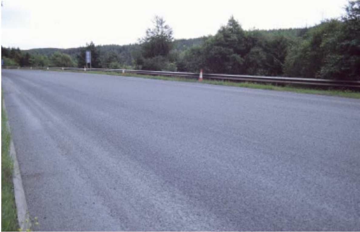
Figure 8.12 Double Surface Dressing Open to Traffic.
