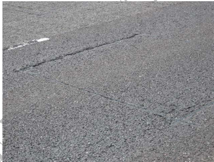
Figure 12.13 Detector Loops may Cause Material Failure
