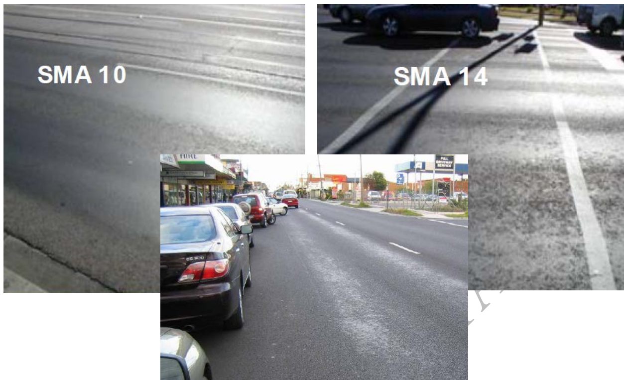
Figure 6.5 Variable Appearance of SMA Surface Course: Binder Rich (SMA 10) and Non-uniform Texture (SMA 14), (Source: Mangan, 2007)
