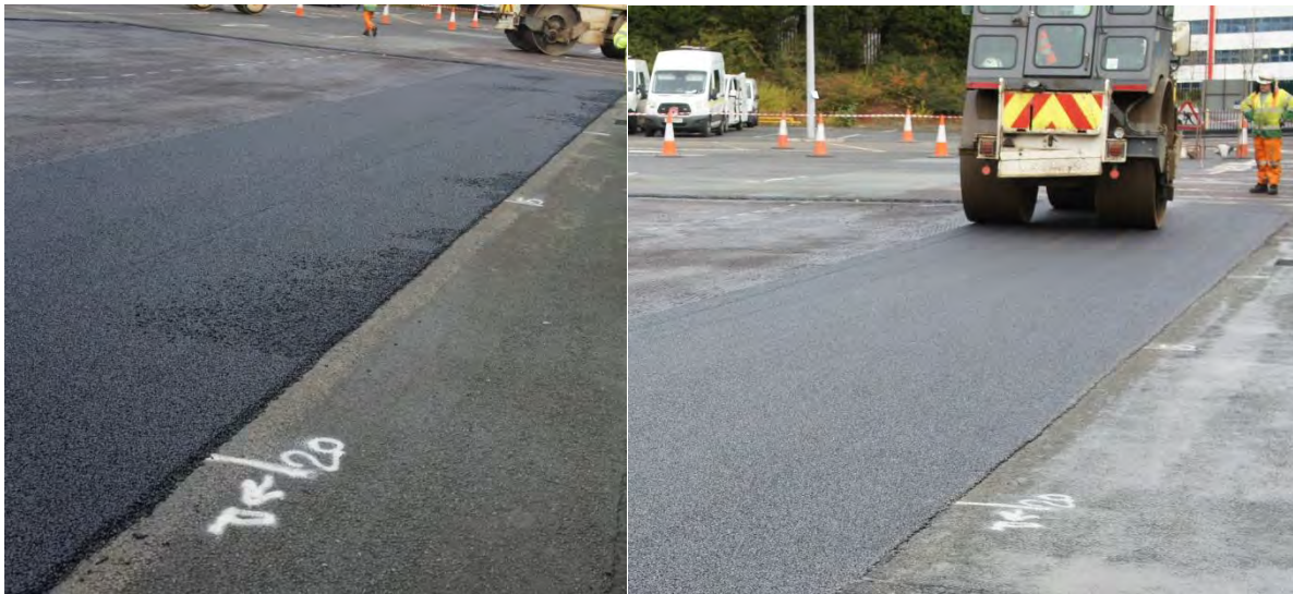
Figure 5: Heated Joint A i) before compaction ii) after compaction
