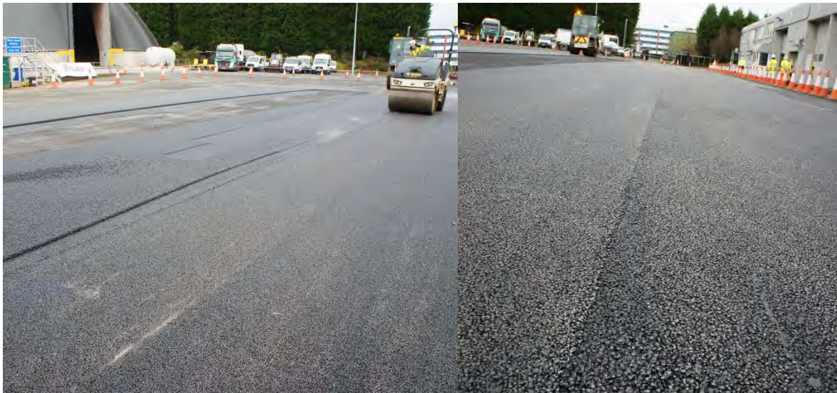
Figure 6: Heated joint B i) before compaction; ii) after compaction
