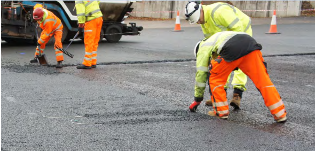
Figure 17: Installation of thermocouples at Rip 1 joint (chainage 34 m)
