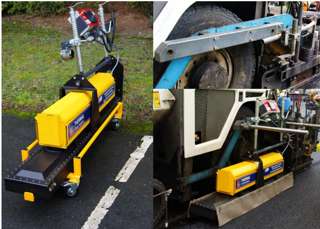
Figure 3: Photographs of the equipment; (clockwise) i) Joint heater equipment, ii) Paver side bar mount, iii) Joint heater technology fitted on the paving machine
