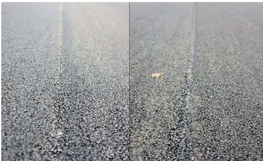
Figure 8: i) Heated Joint C (between Rips 3 and 4); ii) Painted joint D (between Rips 4 and 2)
