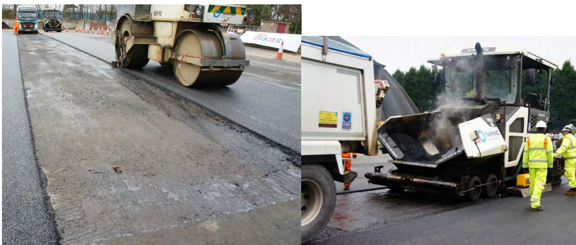
Figure 7: i) Cutting back Rip 2 unconfined edge prior to painting and installing Rip 4; ii) Installing Rip 4
