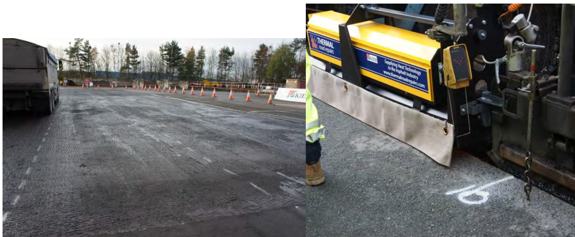
Figure 4: i) Planed surface prior to installation, ii) Joint heater in operation
