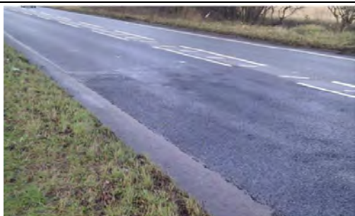
2014 Boundary between WMA (right) and HMA (left)
