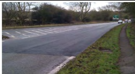
2014 Boundary between HMA & existing surface (looking in Eastbound direction)
