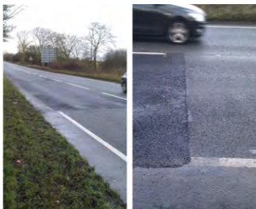
2014 Boundary between WMA and existing surface
