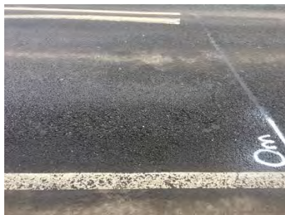
2017 Boundary between WMA and existing surface
