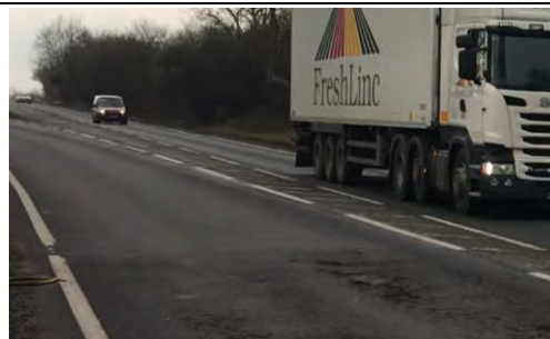
2017 Boundary between WMA (bottom) and HMA (top)
