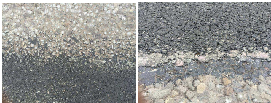
Figure 4: Joint Treated with Paver Mounted Heater (left) and Joint Untreated (right) - Area 9 Paver Mounted Heater Trials, 2016
