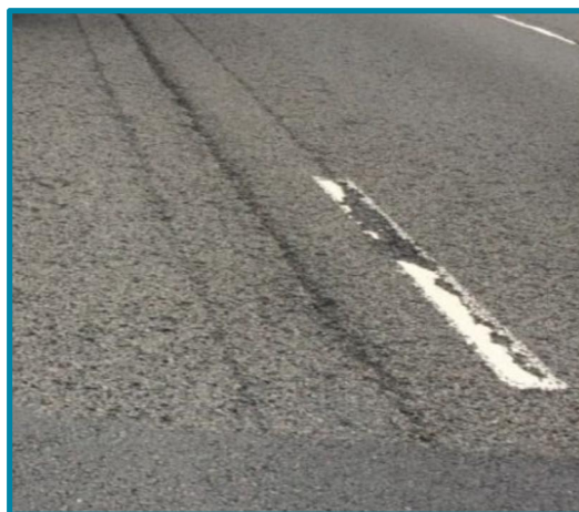
Figure 11: Reflective Cracking from Underlying Joints
