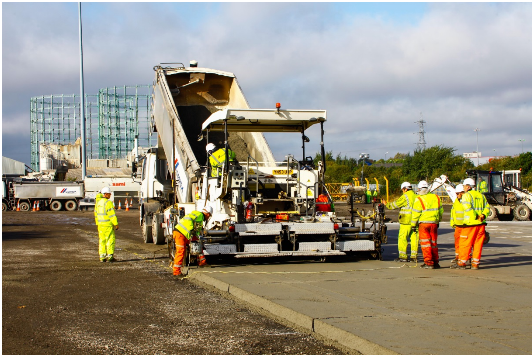
Figure 6 Paver laying RCC with grooving and groove filling taking place behind it
