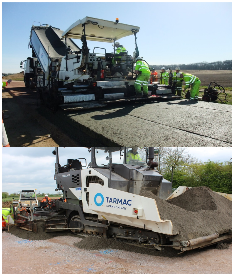
Figure 5 Rigid body truck tipping directly into paver hopper and discharged material in paver hopper
