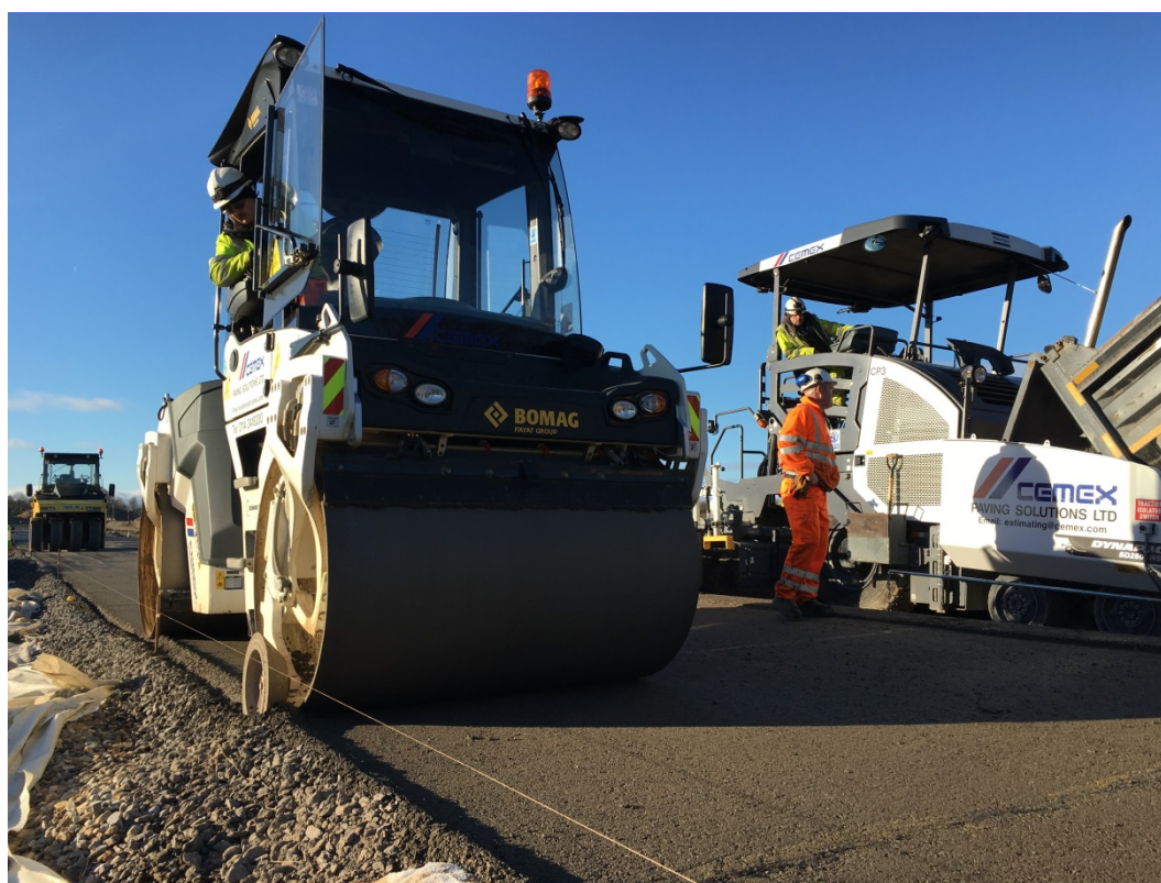
Figure 7 Twin drum roller followed by PTR compacting freshly laid RCC
