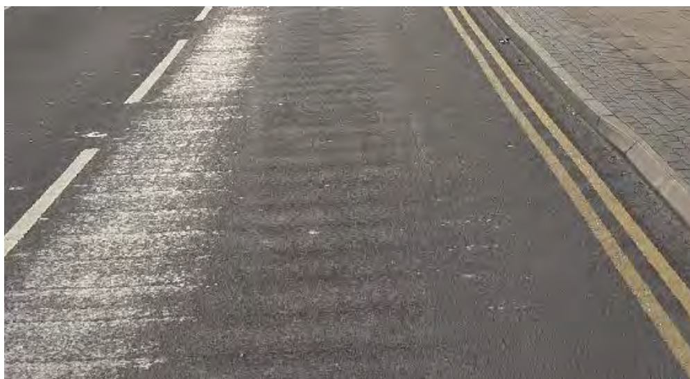
Figure 14: Loss of Texture and Ripples on the High Friction Surface (other)
