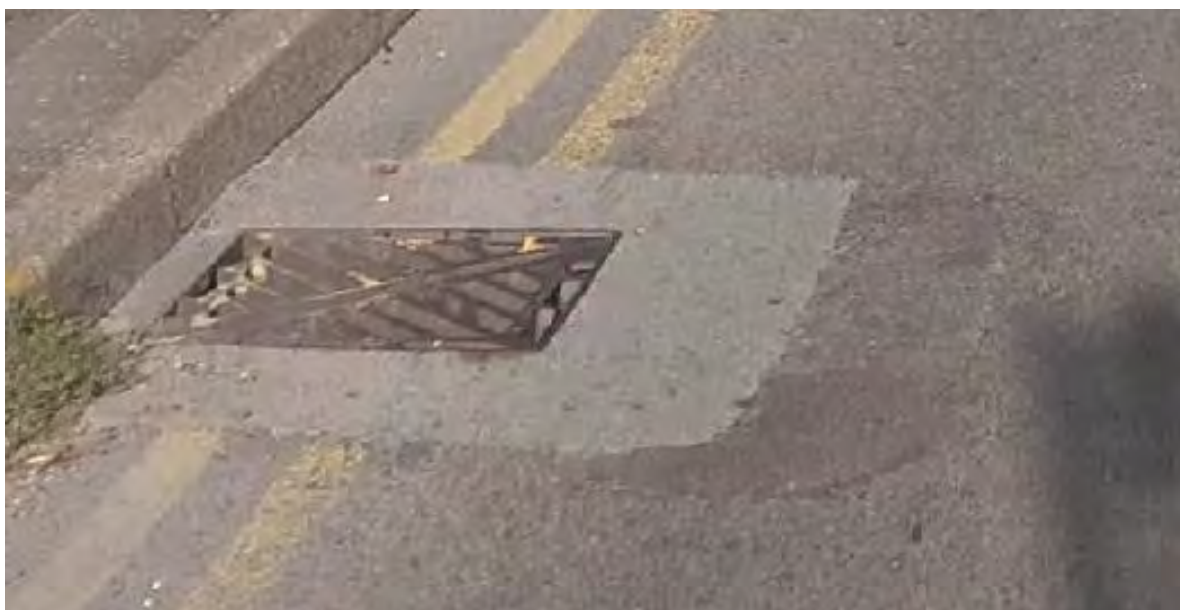
Figure 15: Repairs to Gully (other)
