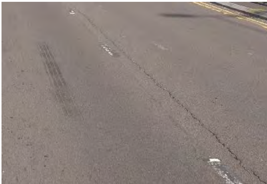
Figure 11: (c) and Open Joints (oj)
