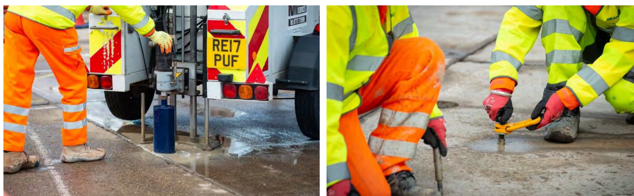
Figure 5.15 Cutting cores at slab corners (left) and placing lifting lugs (right)
