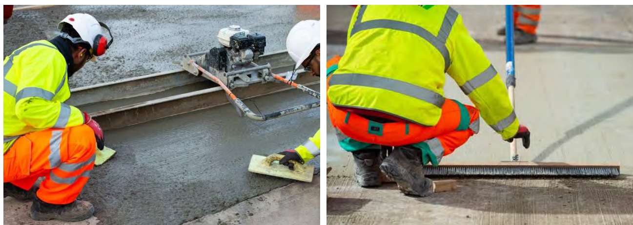
Figure 5.21 Finishing with paddles and a vibrating screed (left) and brushing to give surface texture (right)
