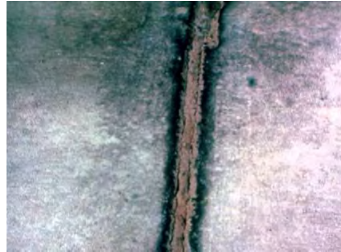
Reference: Pumping - Concrete Surfaced Airfields, Paver Distress Identification Manual [1]
