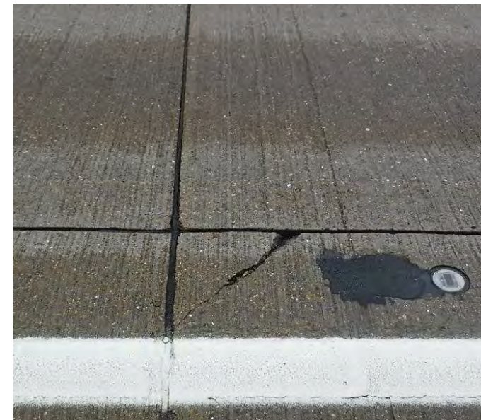
Reference: Corner cracking – Highways England
