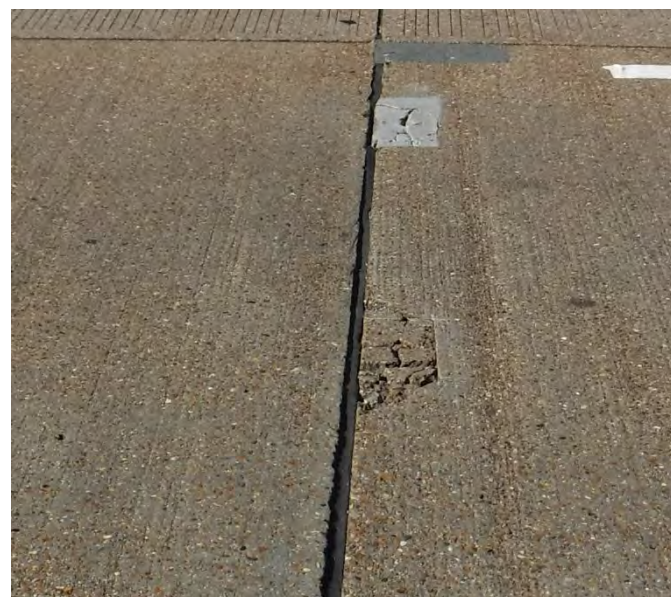
Reference: Joint spall – Highways England
