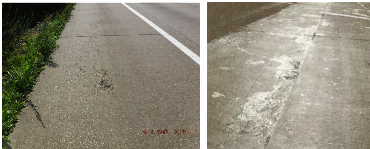
Figure 3.2 Surface scaling
