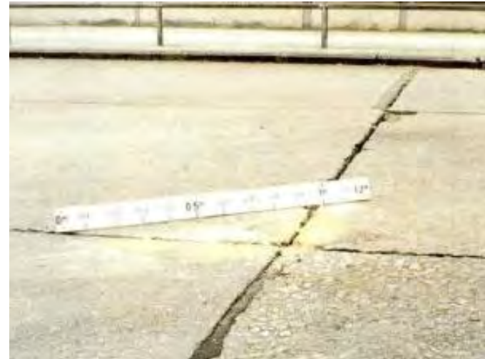
Reference: Slab rocking - CORD [6]
