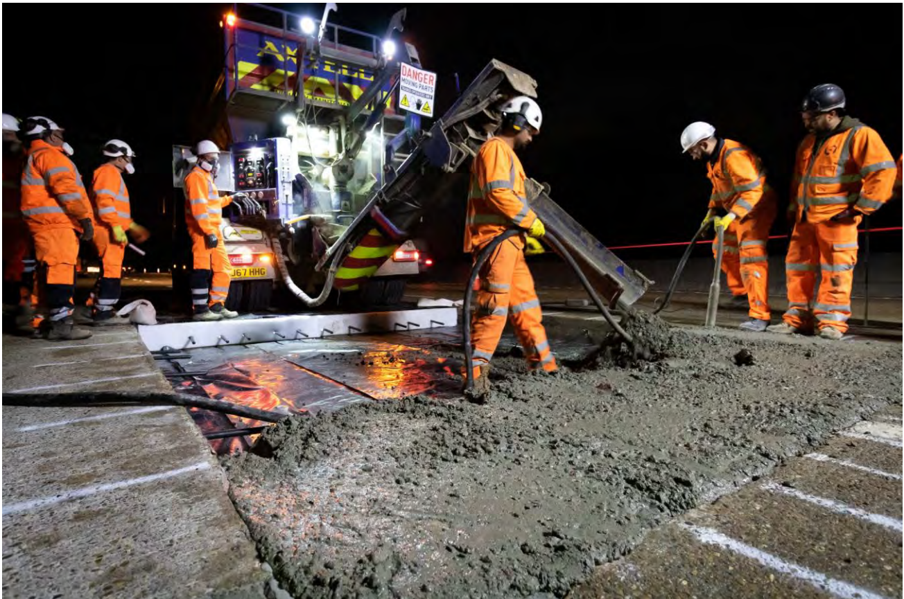
Figure 6.1 Placement of early strength concrete for bay replacements
