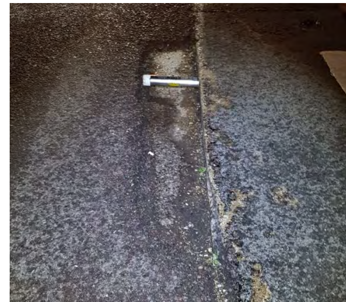
Reference: Asphalt delamination - Highways England
