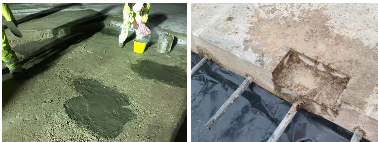
Figure 5.16 Foundation being levelled with rapid setting grout prior to bay replacement (left) and additional breakout of spalled area (right)
