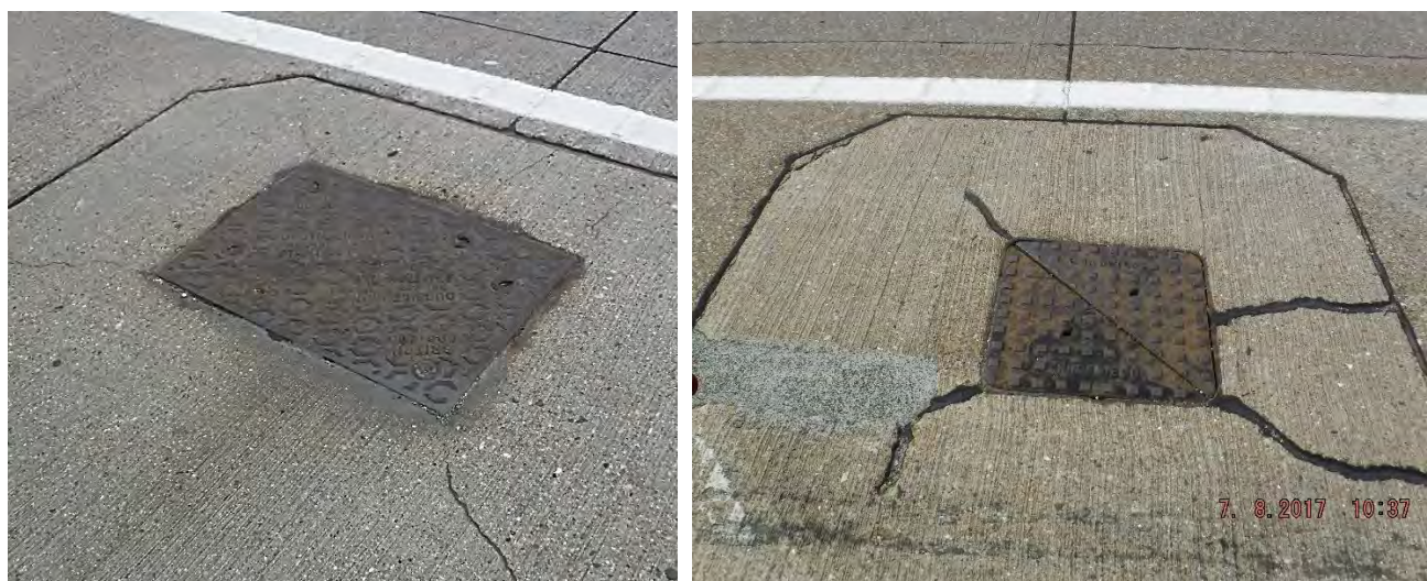
Figure 3.13 Cracks around ironwork
