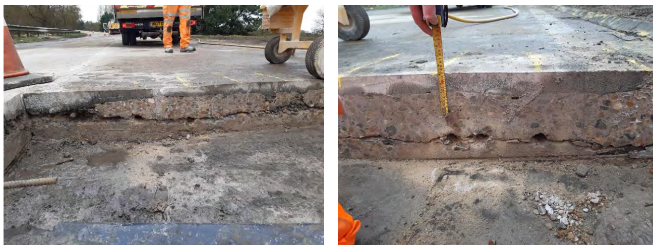
Figure 2.9 Deterioration of concrete extending into the adjacent bay not identified by the pavement investigation prior to repair works
