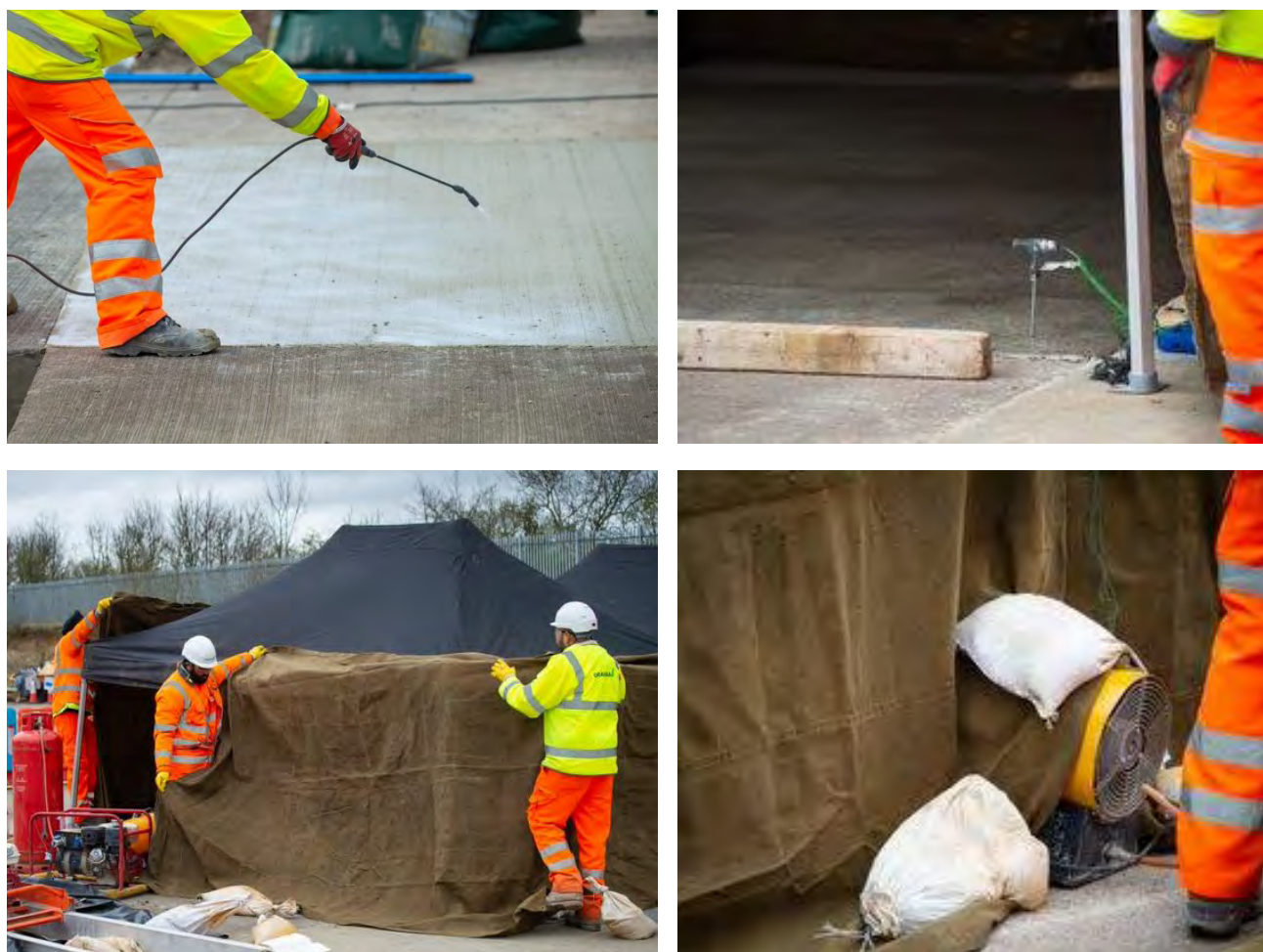
Figure 5.22 Aluminised curing compound being applied (top left), probe insertion to monitor curing rate by temperature-matched curing (TMC) (top right), tents being set up over bay (bottom left), propane heater being used to increase ambient temperature and curing rate (bottom right).
