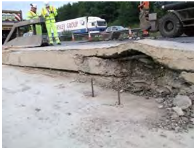
Reference: Compression failure - Highways England
