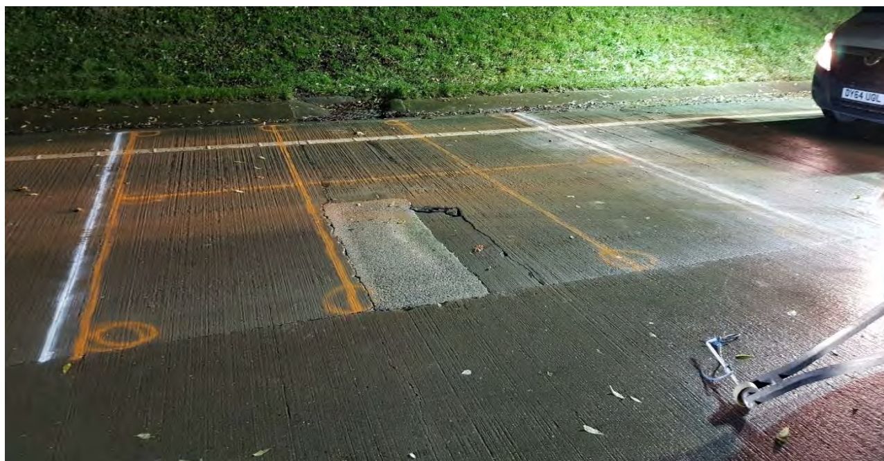
Figure 5.28 Typical CRCP full depth repair dimensions. Full depth saw-cuts in orange and shallow saw-cuts to expose reinforcement for mechanical coupling in white.
