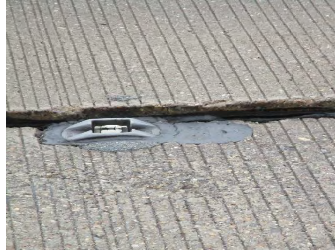
Reference: Joint stepping - Highways England
