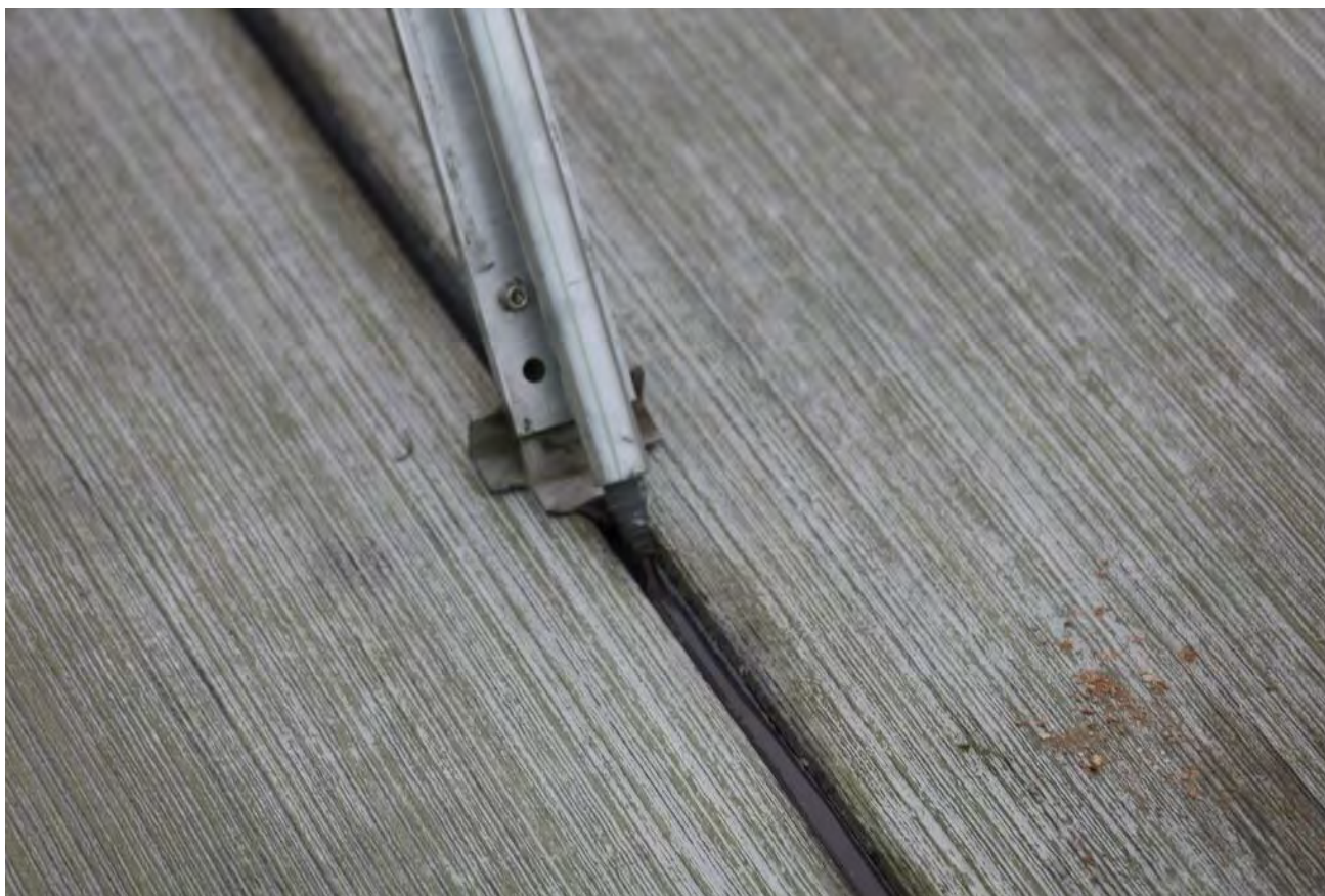
Figure 5.3 Self levelling joint sealant being applied through a nozzle to achieve a uniform recess below the pavement surface
