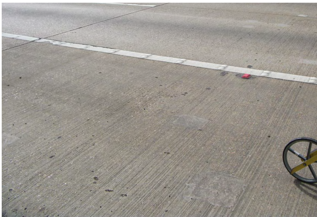
Figure 3.4 Pop-outs and thin bonded repairs to pop-outs
