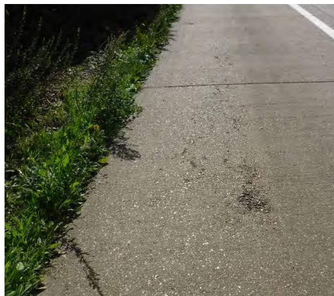
Reference: Surface scaling – Highways England
