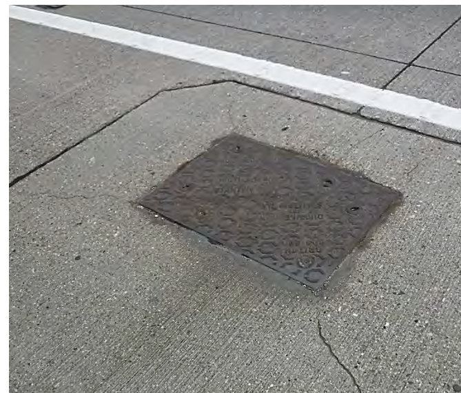
Reference: Cracks Around Manhole - Highways England
