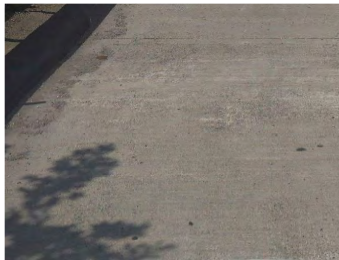
Reference: Surface scaling – Highways England
