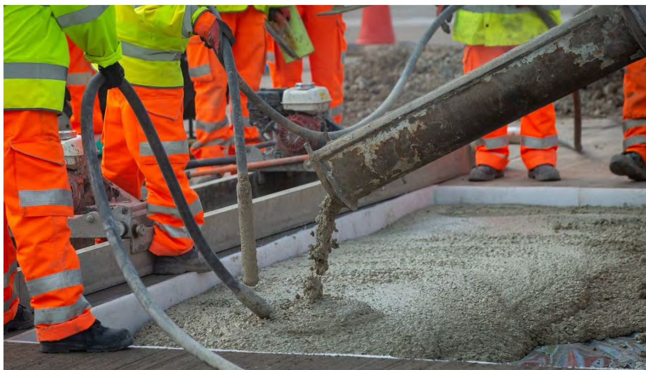
Figure 5.20 Compaction with vibratory poker
