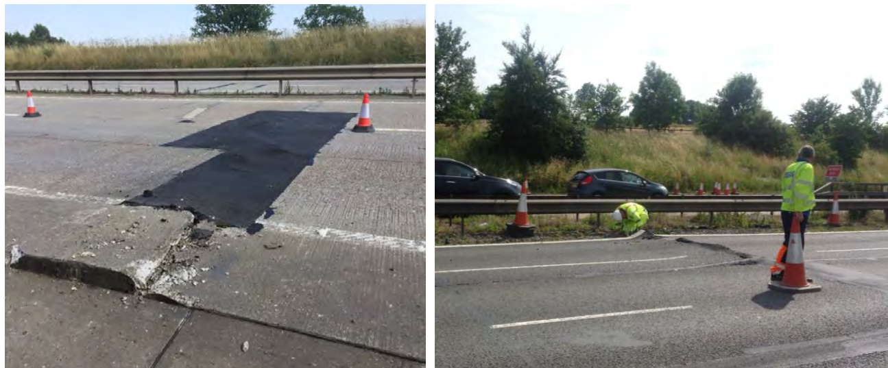
Figure 3.20 Compression failures
