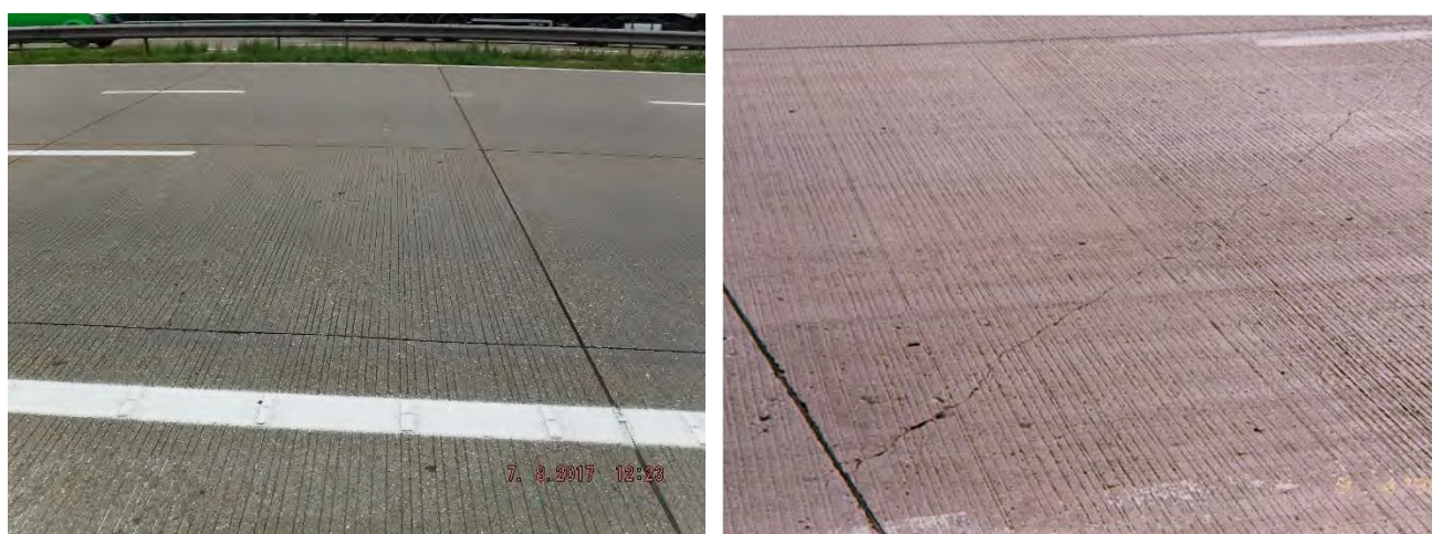
Figure 3.14 Diagonal cracks
