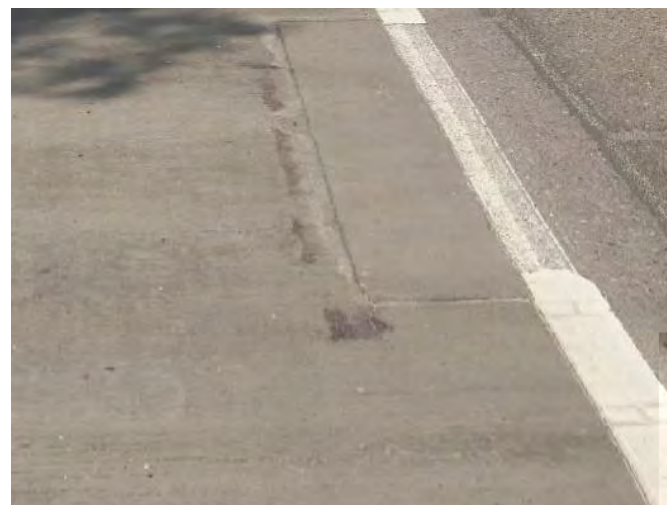
Reference: Rust staining and patching
