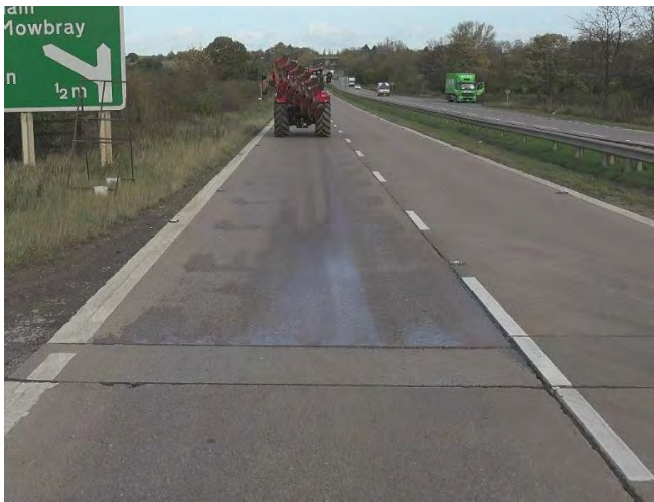
Figure 3.19 Slab rocking (evidenced by pumping)
