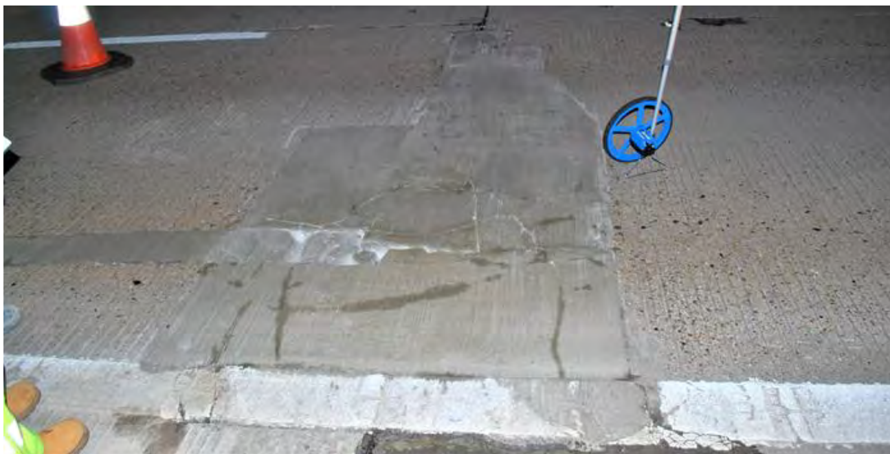
Figure 5.9 Failure of a shallow repair undertaken with a rigid repair material using an irregular shape and spanning a joint without re-establishing the joint
