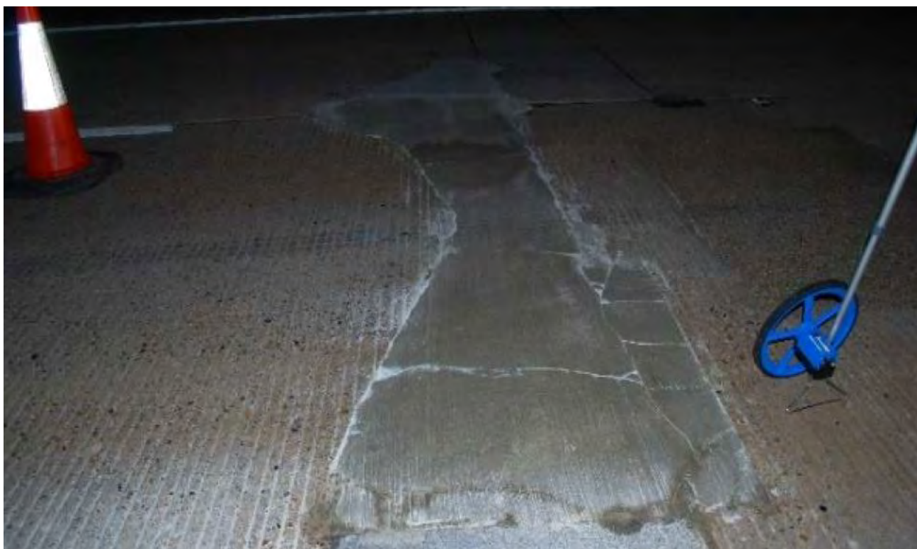
Figure 5.10 Failure of an irregular shaped shallow repair spanning a joint without re-establishing the joint
