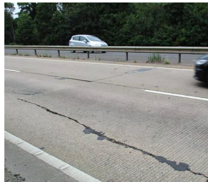
Reference: Longitudinal crack - Highways England
