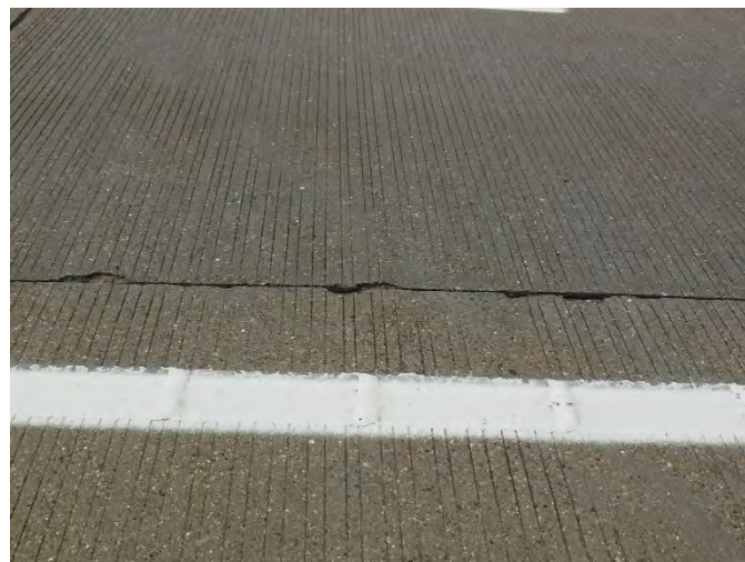
Reference: Joint spall - Highways England
