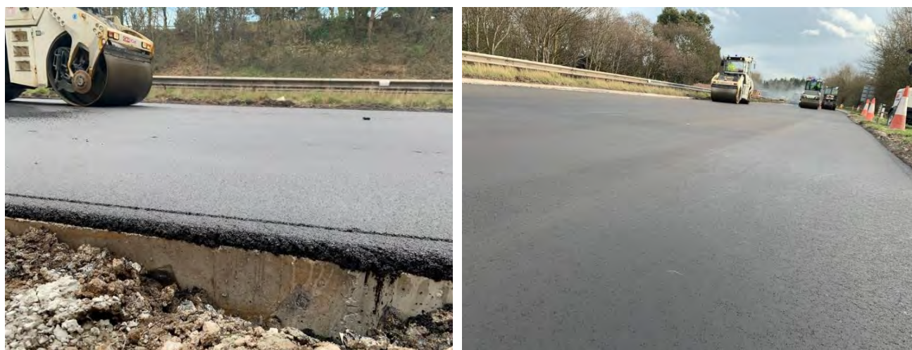
Figure 7.6 Asphalt SAMI over URC
