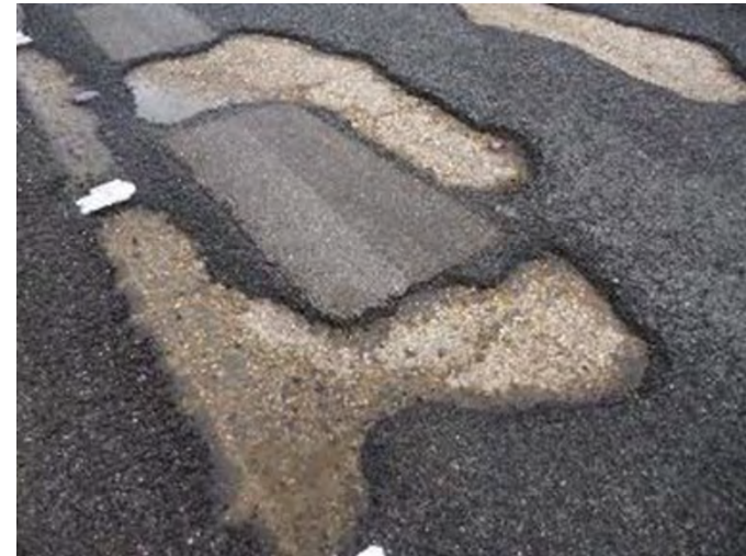
Reference: Asphalt delamination - Highways England
