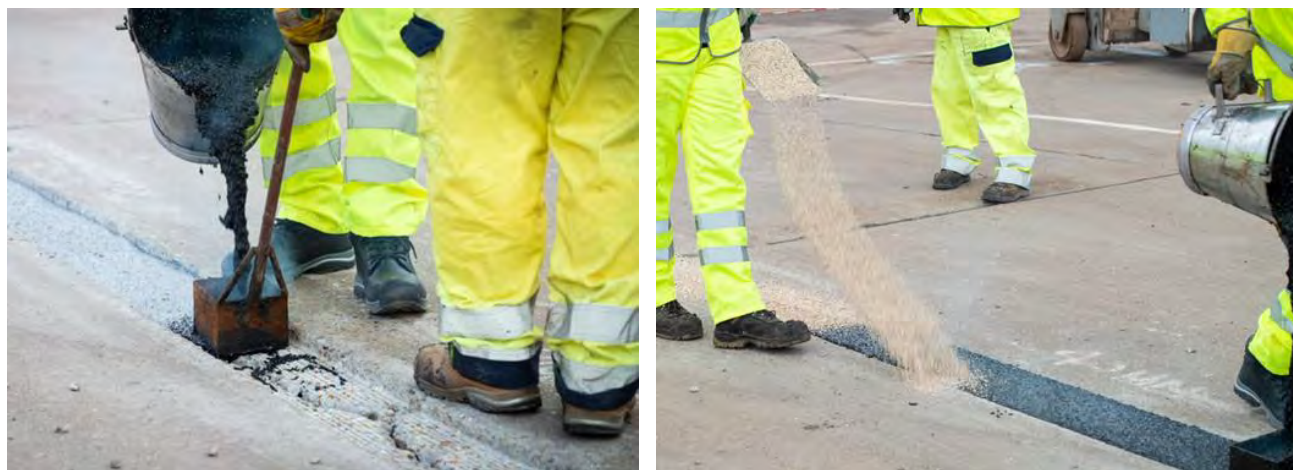
Figure 6.4 Inlaid crack repair using polymeric material
