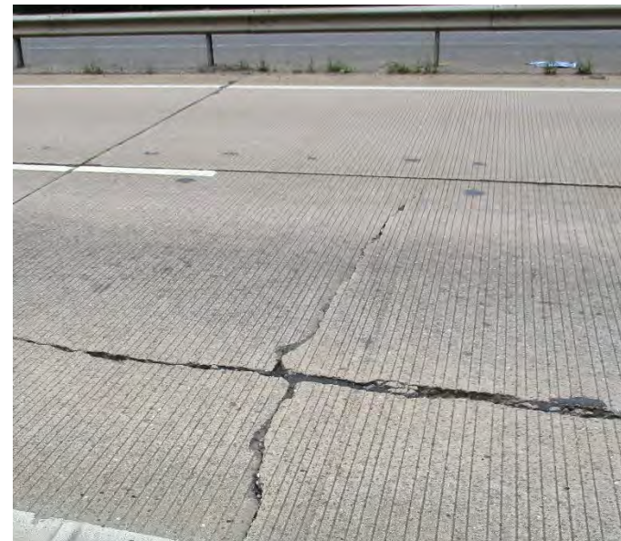
Reference: Shattered slab - Highways England
