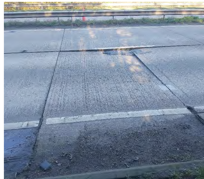
Reference: Slab rocking - Highways England
