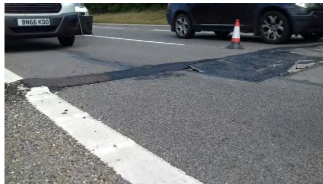
Reference: Surface irregularity - Highways England
