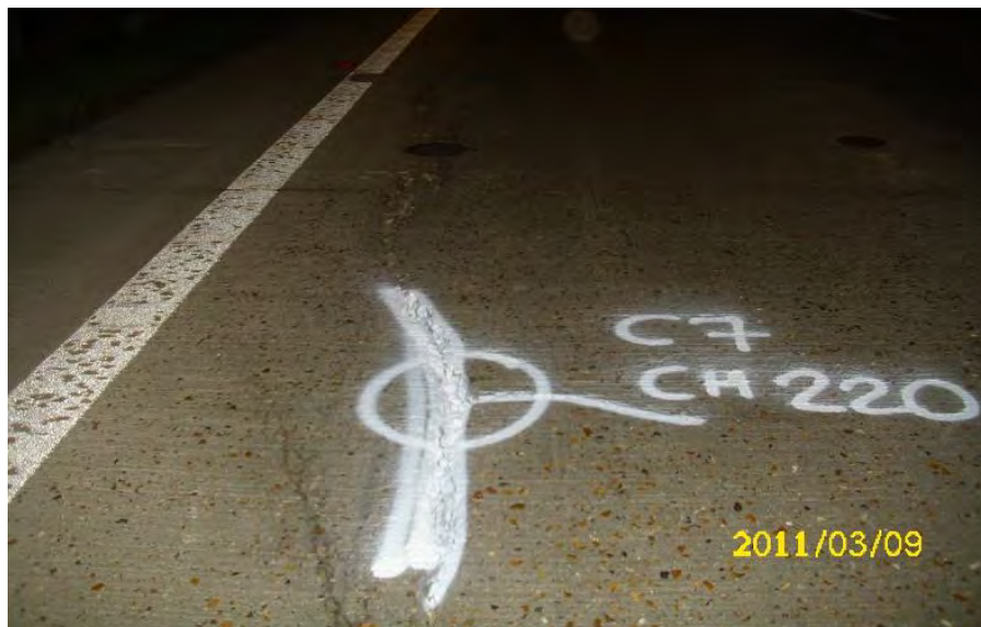
Figure 3.23 Longitudinal crack in CRCP
