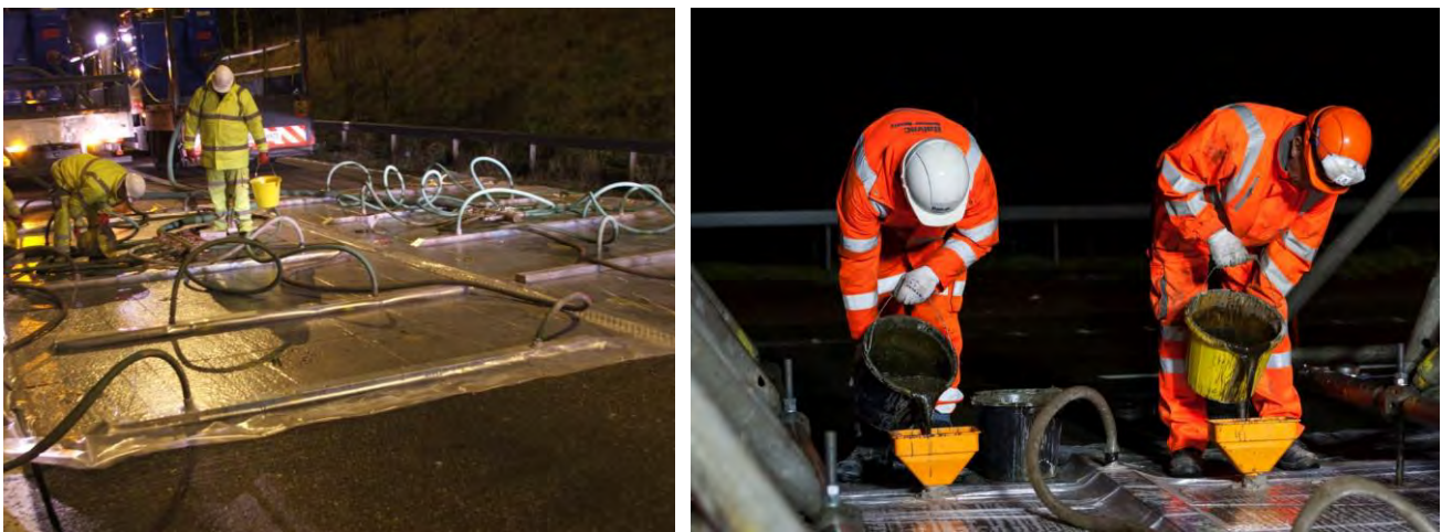
Figure 5.35 Vacuum grouting
