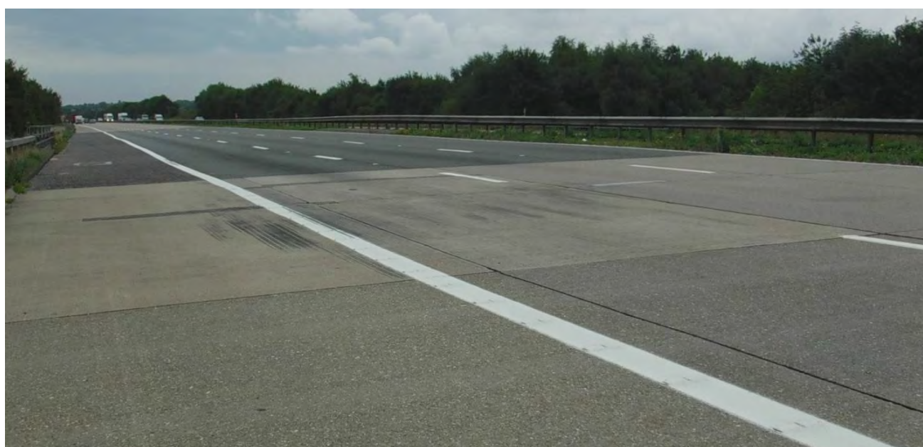
Figure 3.1 Surface irregularities evidenced by rubber deposits on road surface
