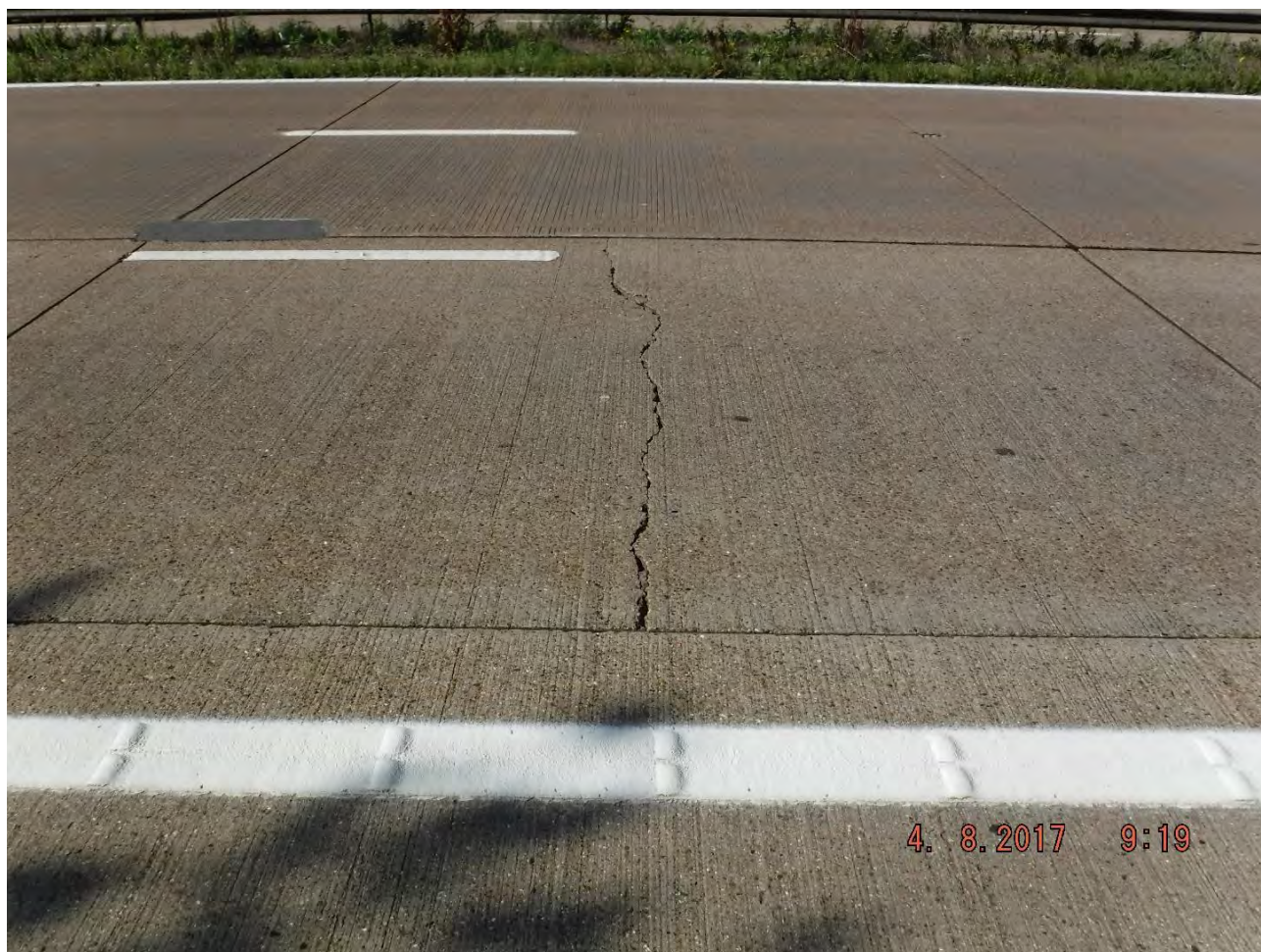
Figure 3.15 Transverse crack
