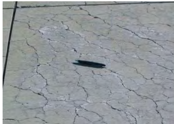
Reference: Alkali silica reaction - DIO Technical Standard - Airfield 05 -2019 [2]
