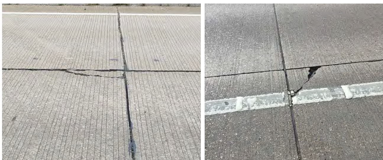
Figure 3.12 Corner cracks
