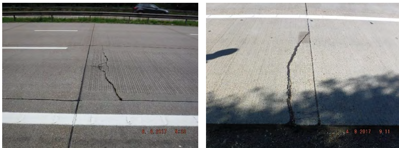
Figure 3.16 Transverse cracks in URC in proximity of a joint
