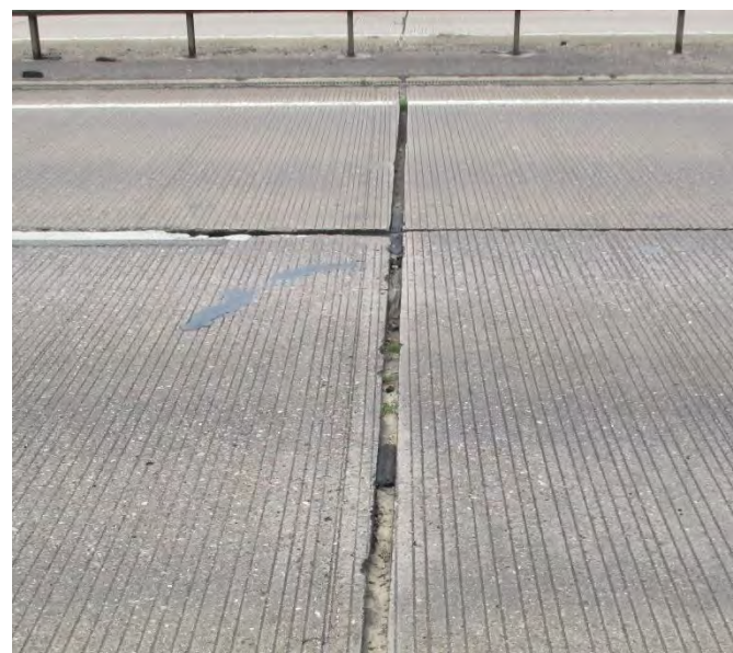
Reference: Joint seal damage - Highways England
