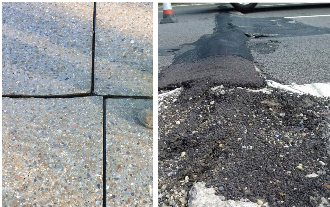
Figure 4.2 Shoving (left) and compression failure (right)
