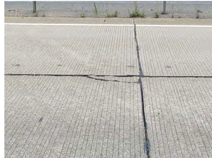
Reference: Corner cracking - Highways England
