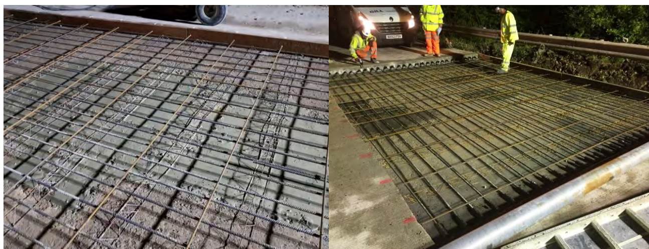
Figure 5.27 Prepared reinforcement and foundation
