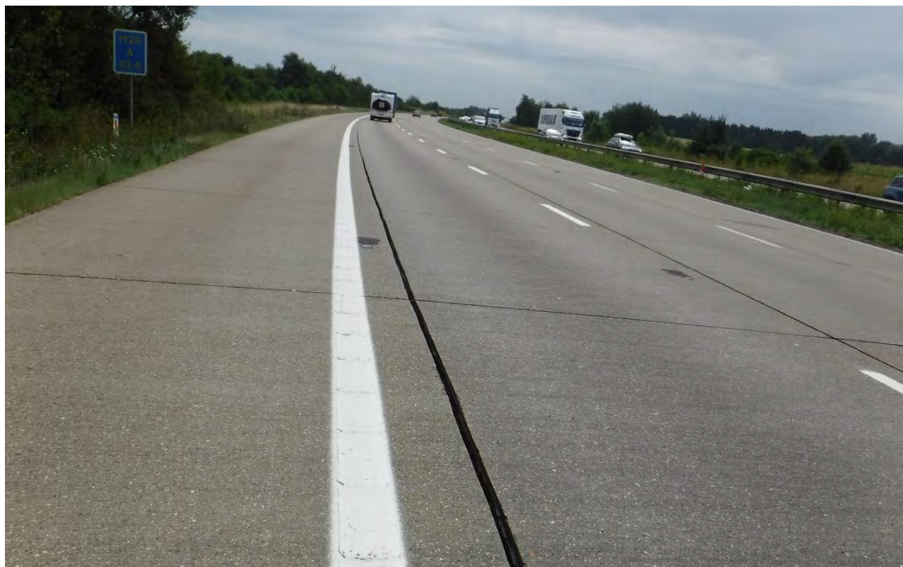
Figure 3.6 Adhesion failure of the joint seal in longitudinal joint as a result of the joint opening up
