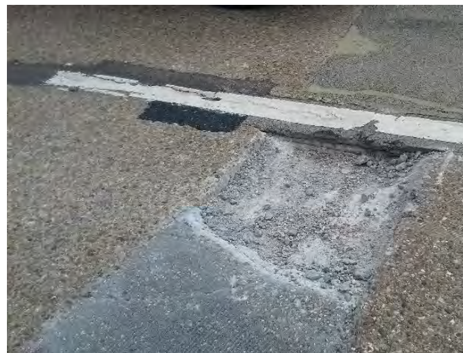
Reference: Patching failure - Highways England
