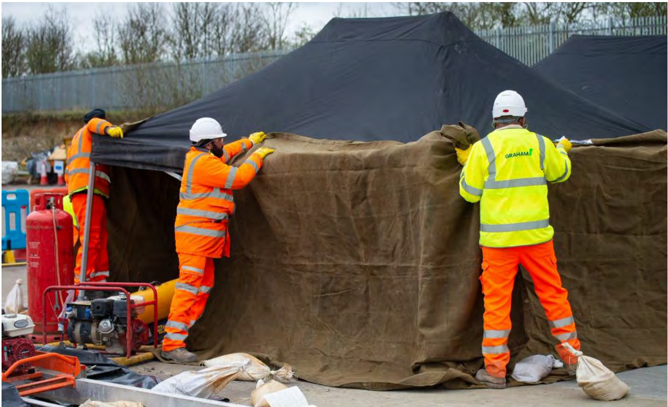
Figure 6.2 Tenting and heating of bay replacements with early strength concrete to increase strength development rate
