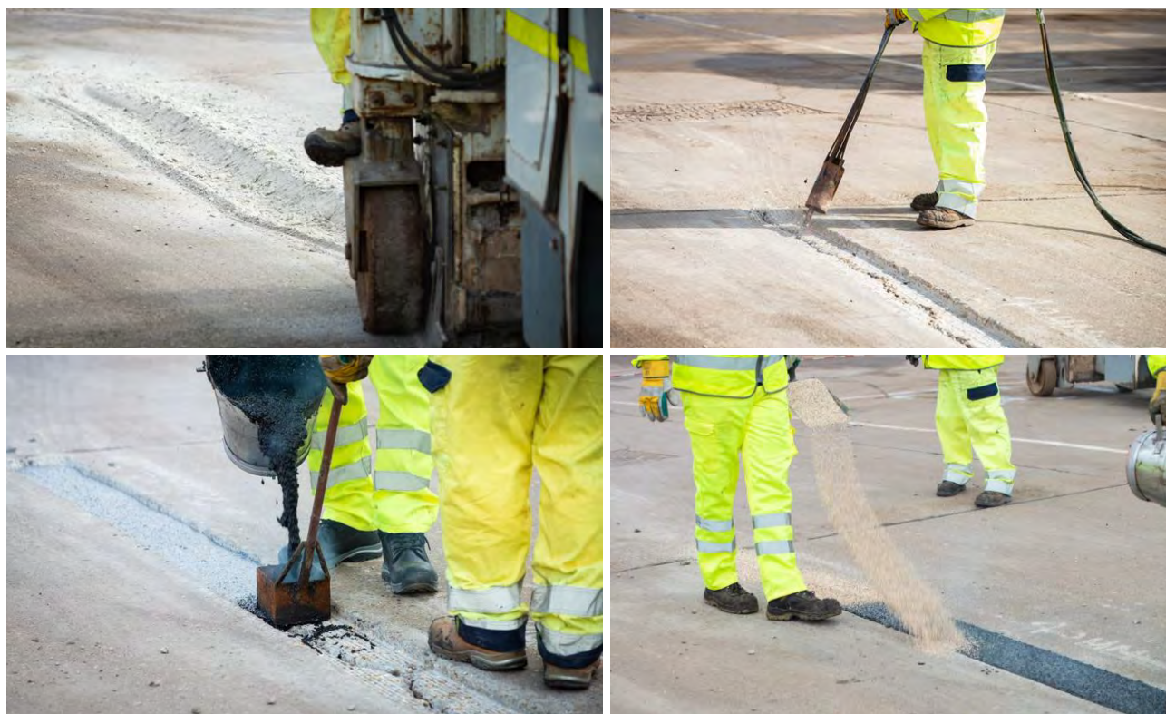
Figure 5.12 Inlaid crack repair process. Milling recess (top left), cleaning / drying recess (top right), filling recess (bottom left), applying chippings (bottom right).
