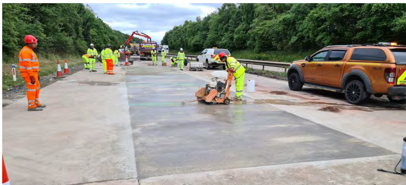
Figure 5.24 Sawing transverse joint grooves between bays
