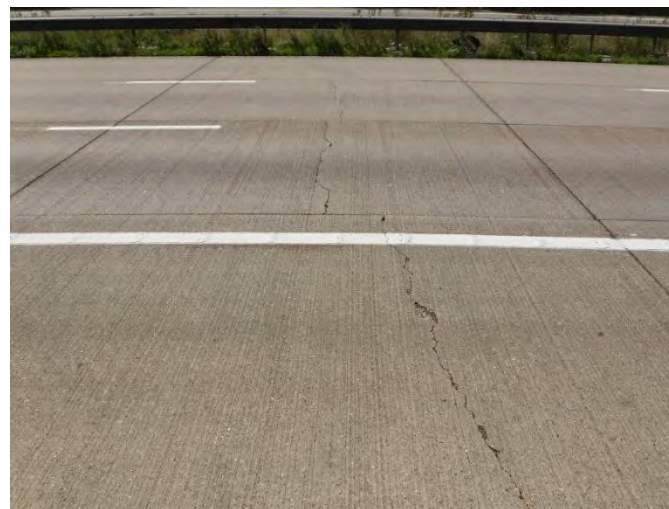
Reference: Transverse crack - Highways England
