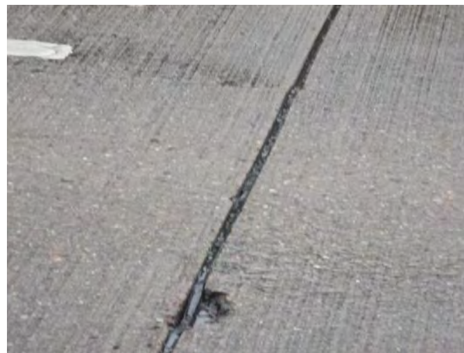
Reference: Joint seal damage and spalling - Highways England
