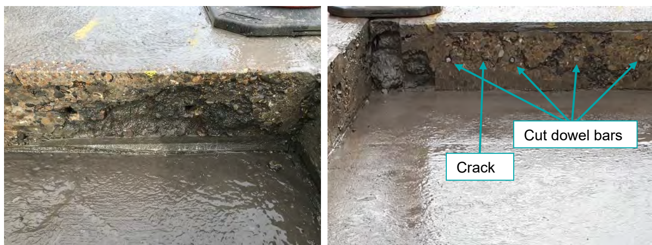
Figure 5.17 Unsuitable joint faces to receive load transfer devices
