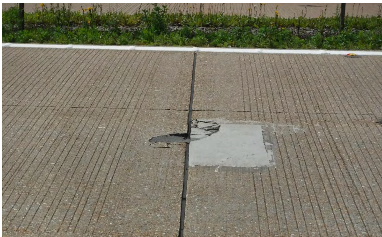
Figure 3.11 Deep joint spalls
