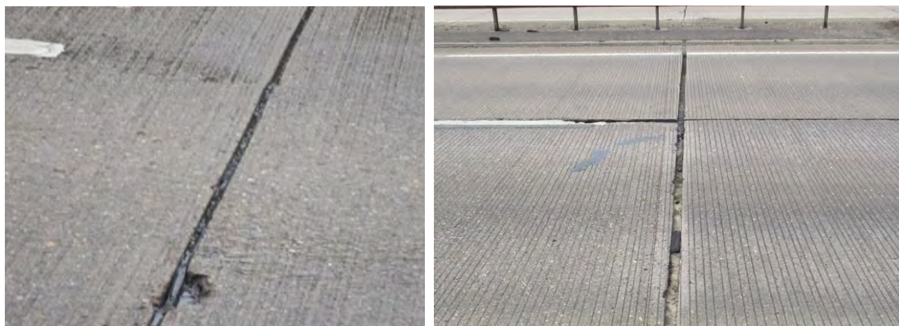
Figure 3.5 Defective joint seals
