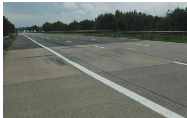
Reference: Surface irregularity - Highways England
