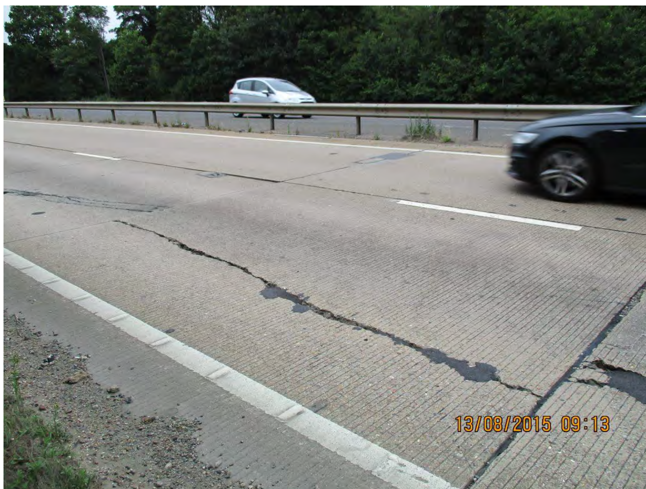
Figure 3.17 Longitudinal crack
