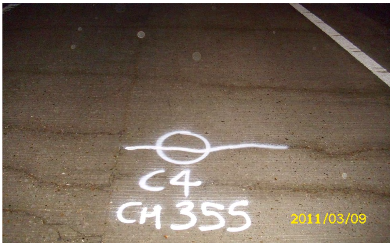
Figure 3.22 Significant transverse cracks in CRCP
