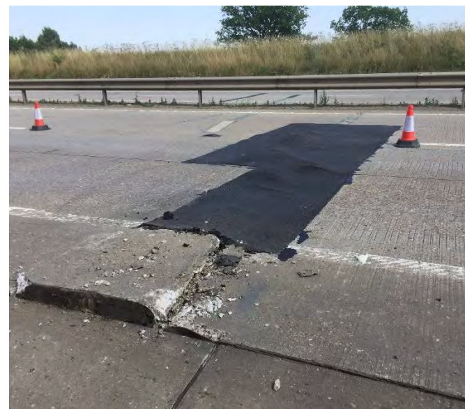
Reference: Compression failures and patching - Highways England
