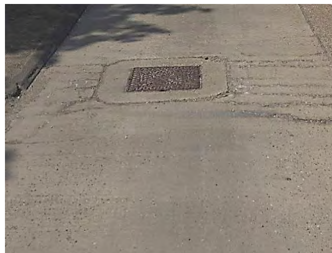
Reference: Cracks Around Manhole - Highways England
