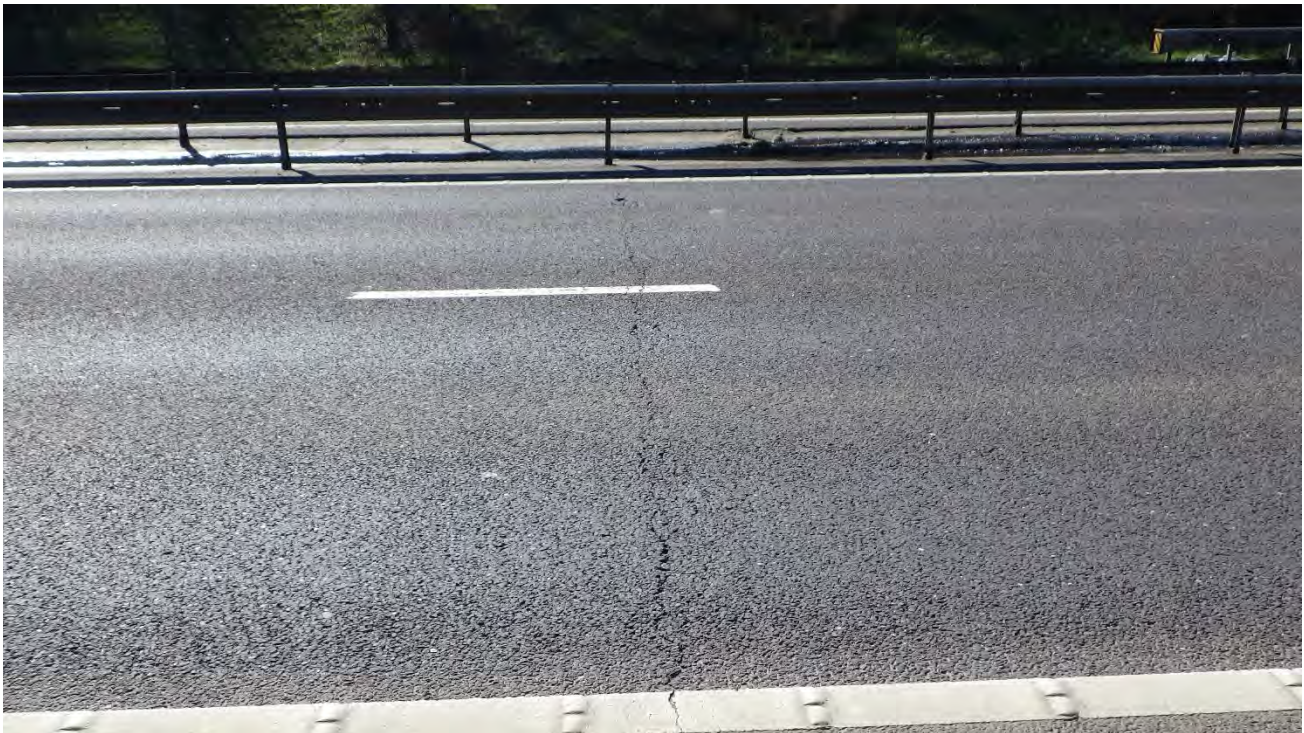
Figure 7.1 Reflective cracking in an asphalt overlay caused by an underlying joint / crack
