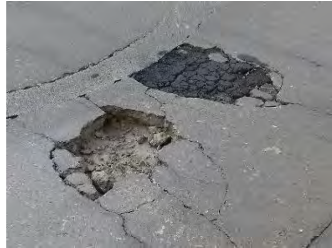
Reference: CRCP punchout and patching failure - Highways England
