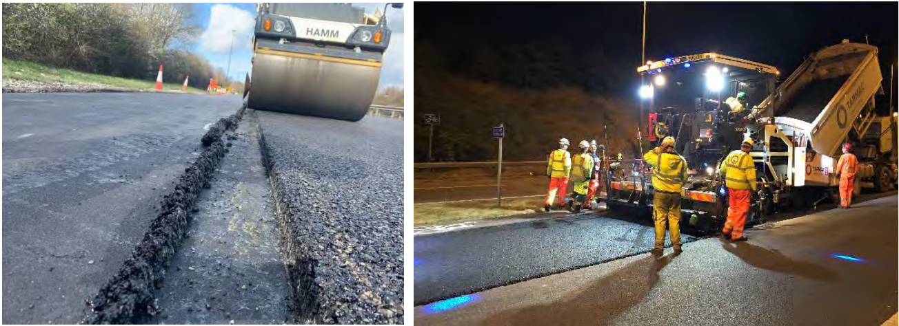
Figure 7.7 TSCS installation
