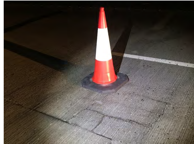
Reference: Shattered slab - Highways England
