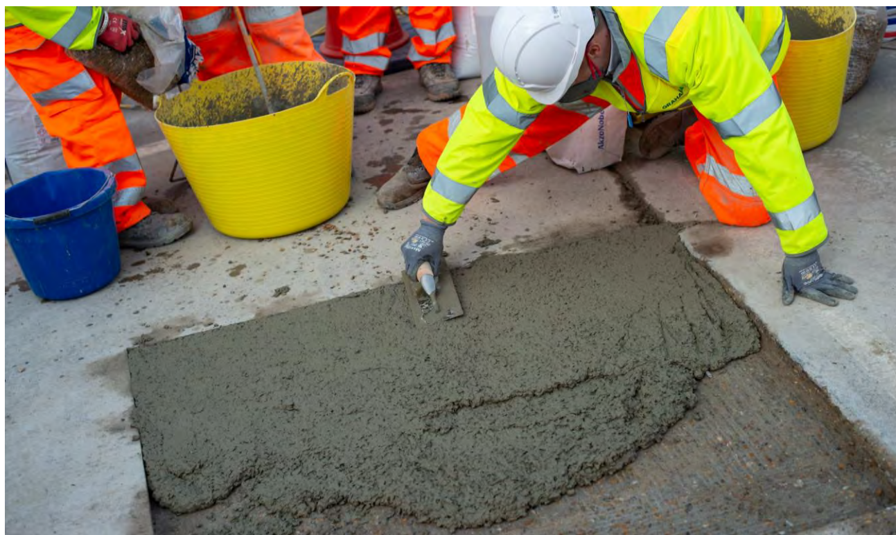
Figure 5.7 Installation of a shallow repair
