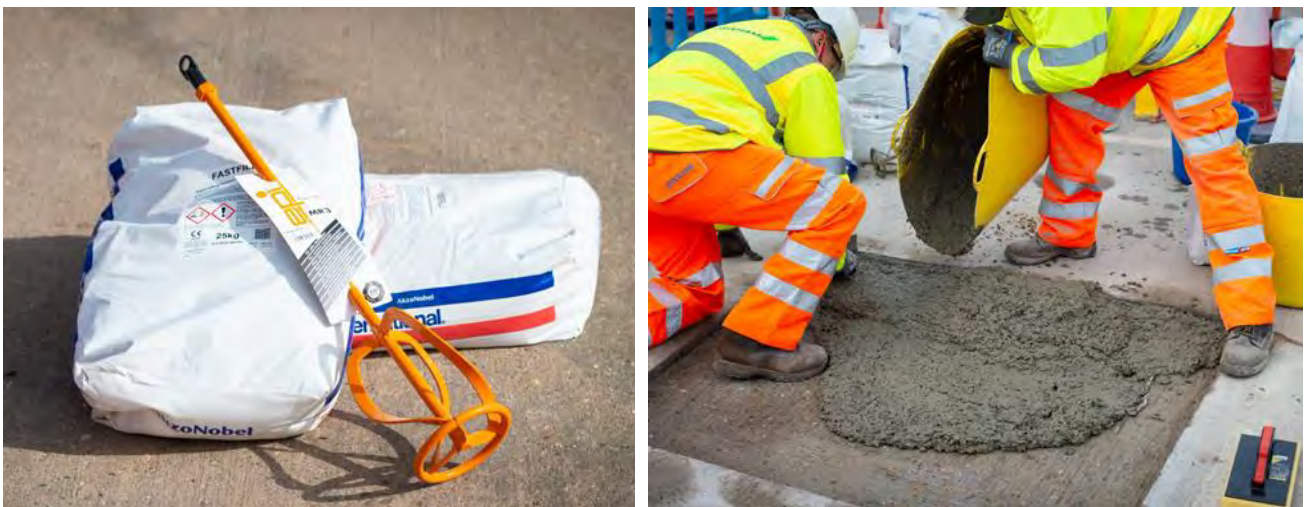
Figure 6.3 Polymer modified cement mortar
