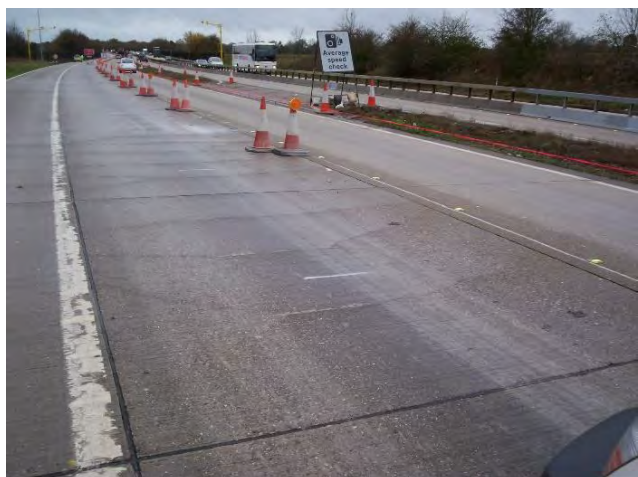
Figure 7.8 Crack and seat of URC pavement after slab cracking at 1 m intervals prior to asphalt overlay
