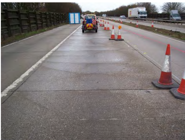
Figure 7.8 Crack and seat of URC pavement after slab cracking at 1 m intervals prior to asphalt overlay
