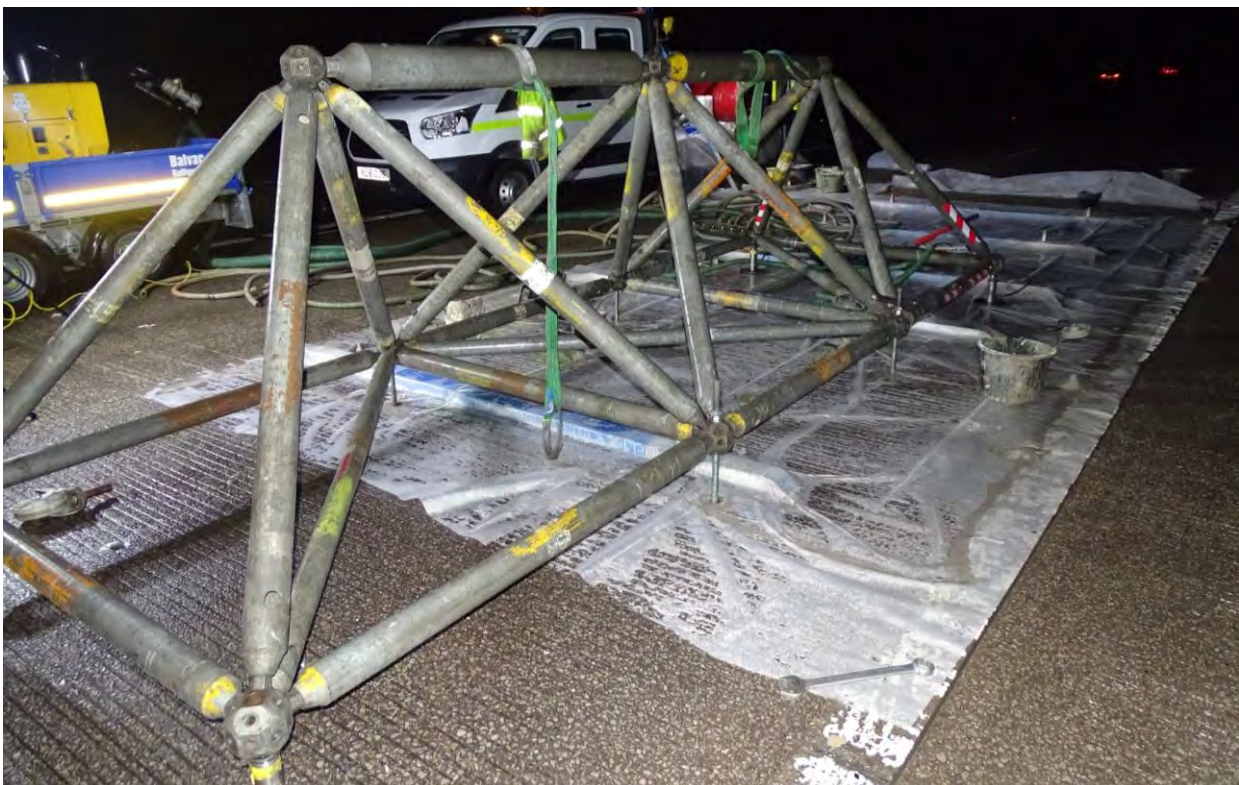
Figure 5.36 Slab lifting apparatus used in conjunction with vacuum grouting
