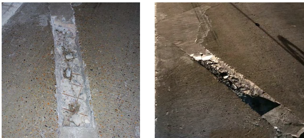
Figure 5.11 Failure of an irregular shape, high aspect ratio shallow repair undertaken over a working crack
