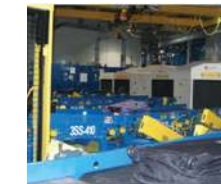
Orlando International Airport (MCO) Airport Security Improvement Program, Orlando, FL
