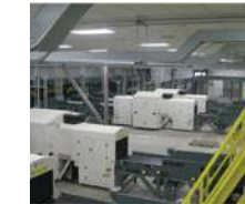
Orlando International Airport (MCO) Remote Baggage Screening Facility, Orlando, FL
