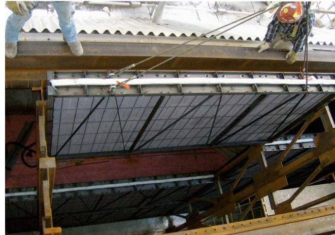
Mercury oxidation catalyst modules being installed for a full-scale demonstration.
