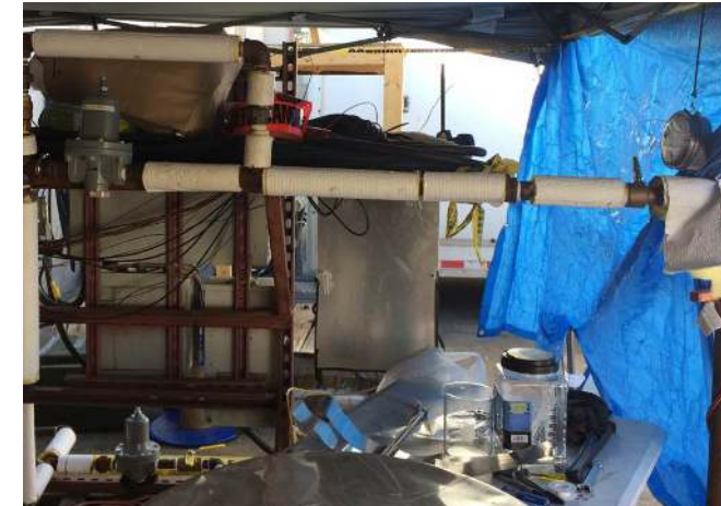
Molten salt thermal energy storage pilot-scale system.
