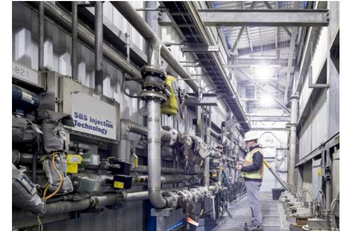
The distribution manifold and injection lances for a commercial SBS Injection™ System.
