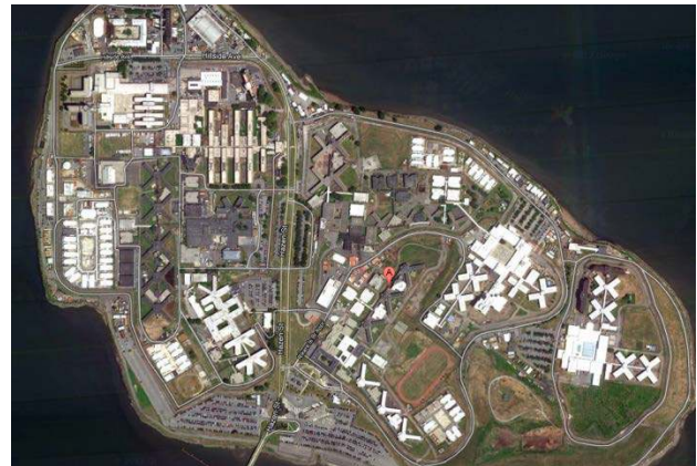
Figure 1. AECOM Designed and commissioned a 15MW microgrid in New York State.
