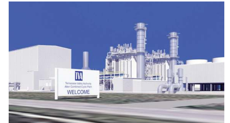
TVA, Allen Combined Cycle Project Memphis, Tennessee, U.S.A.
