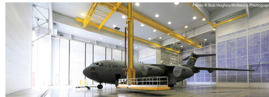
AECOM's design and construction services on a design-build 60,000-sf C-17 corrosion control hangar facility and a 20,000-sf maintenance facility at Hickam AFB in Hawaii earned a PACAF Design Award.
