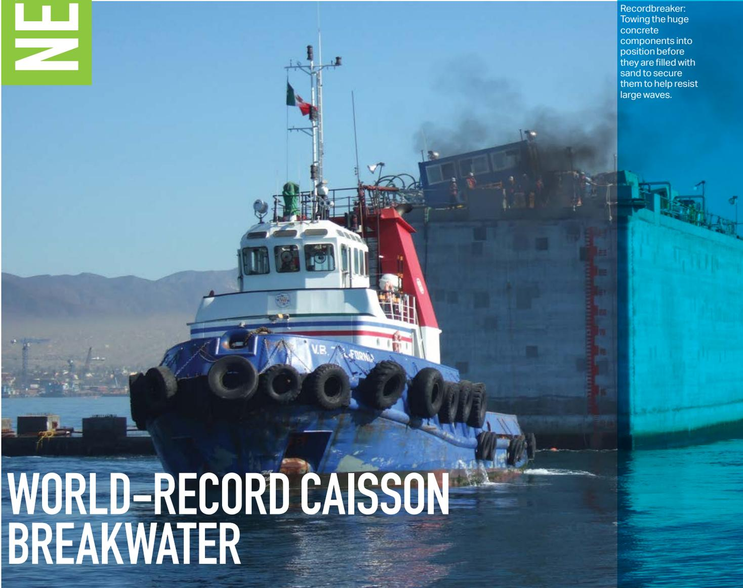
Recordbreaker: Towing the huge concrete components into position before they are filled with sand to help resist large waves.
