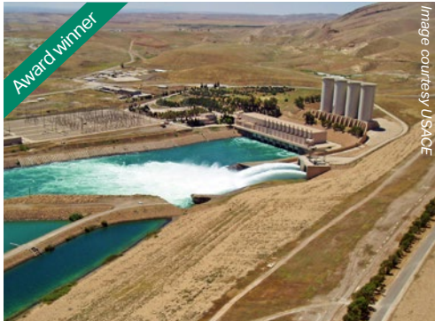
Mosul Dam Rehabilitation (Iraq) A/E services in support of USACE Engineer of Record during rehab focused on foundation grouting and repair of bottom outlets
