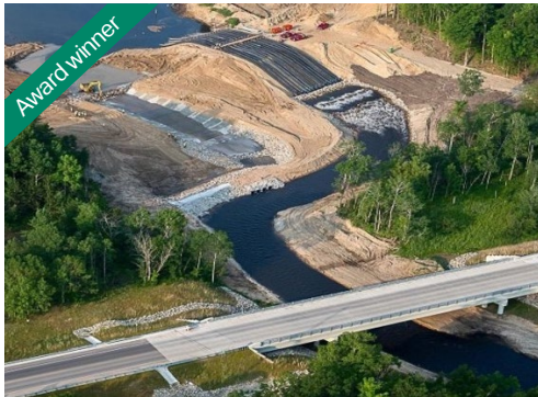
Boardman River Dam Removal (MI) On Michigan's largest river restoration project, supported USACE with work including natural channel design, structural and geotechnical analysis of dam breaching, and sediment management
