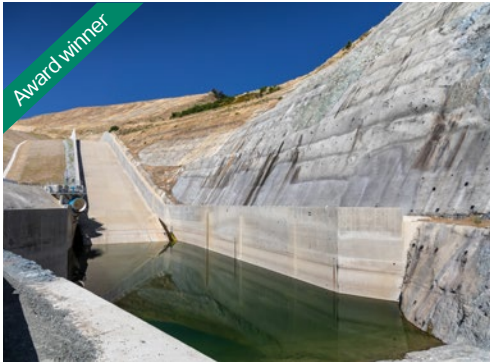
Calaveras Dam Replacement (CA) Planning, permitting, and conceptual and final engineering design services that met dam safety and strict environmental compliance requirements
