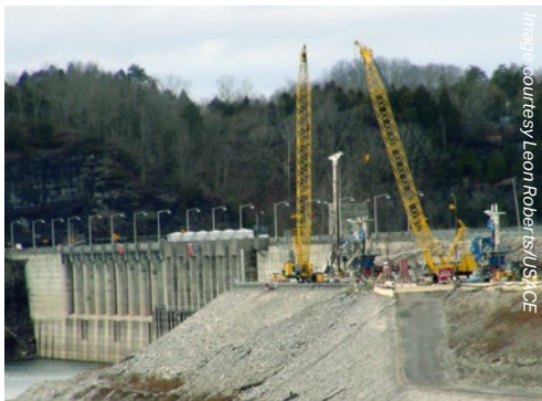
Wolf Creek Dam Instrumentation System Design, Installation & Operation (KY) Provided some of the most critical dams with safety performance monitoring/early warning systems
