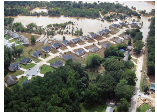
Hurricane Florence Sheltering & Temporary Essential Power Program (NC) Provided case management for 14,000+ applicants to repair critical damage and restore power for residents to safely shelter at home
