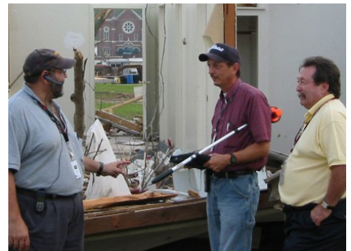
Hurricane Katrina Neighborhood Home Program Prepared 5,700+ damage assessments and 13,000+ environmental review records for a $5.4B recovery program
