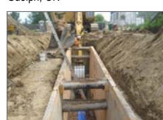
Light-Rail Transit (LRT) – Water; Wastewater; Stormwater Operational Impact Study , Hamilton, ON
