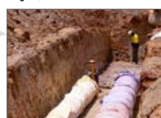
Asset Management Plans Development , Australia
