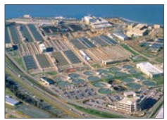
Asset Management Strategy to Improve O&M Efficiency , Washington, DC
