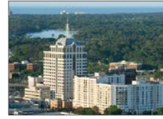
Condition Assessment of Force Main Infrastructure, Virginia Beach, VA
