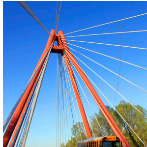
East Fork White River Bridge
