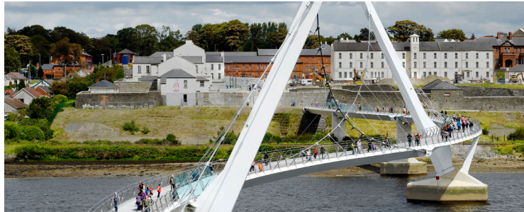
Peace Bridge over River Foyle Derry/Londonderry, Northern Ireland Feasibility, conceptual and final design; construction support 2011
