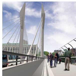
East 153rd Street Bridge
