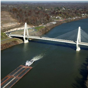
Bridge of Honor over the Ohio River Pomeroy, Ohio, United States Conceptual, preliminary and final design; construction support 2008
