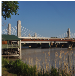
Interstate-35 Bridges over the Brazos River Waco, Texas, United States Conceptual, preliminary and final design; construction support 2014
