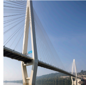
Ironton-Russell Bridge over the Ohio River
