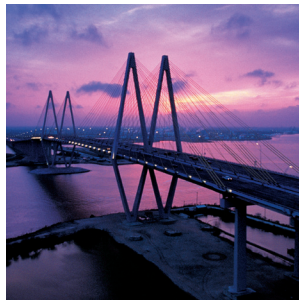
Fred Hartman Bridge
