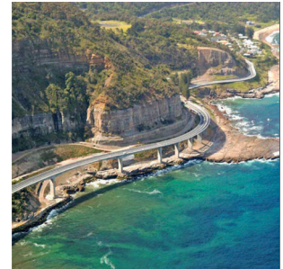
Sea Cliff Bridge and Lawrence Hargrave Drive Upgrade Illawarra, New South Wales, Australia Concept and preliminary design; detailed design and documentation; construction stage services 2005
