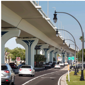
Selmon West Extension Design-Build Tampa, Florida, United States Final design; construction support 2021
