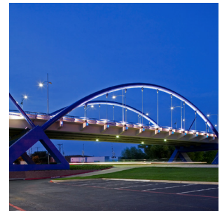
Arapaho Road Bridge
