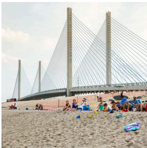
Charles W. Cullen Bridge at the Indian River Inlet
