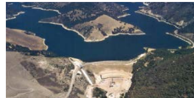
Lopez Dam Seismic Remediation Project San Luis Obispo County, CA
