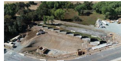
Argonaut Dam Remediation Jackson, CA
