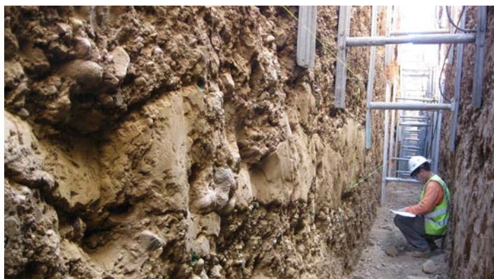
Santiago Creek Dam
