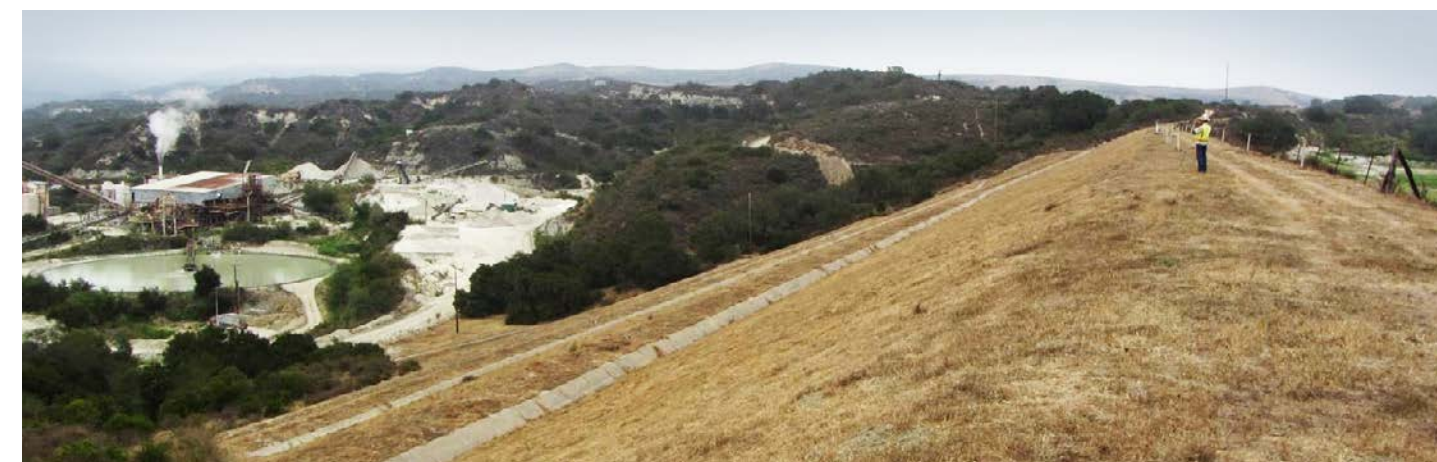
Trampas Canyon Dam
