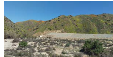
Lee Lake Dam Upgrade Project Corona, CA
