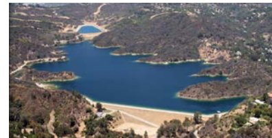
Stone Canyon Dam Seismic Stability Evaluation Los Angeles, CA
