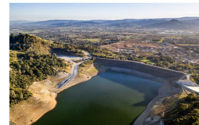
Anderson Dam Seismic Retrofit
