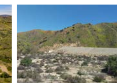
Lee Lake Dam Upgrade Project Corona, CA
