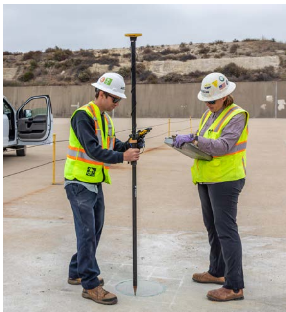
Prado Dam Spillway Raise Project
