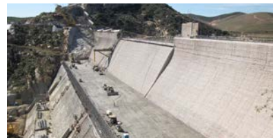
San Vicente Dam Raise San Diego, CA
