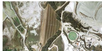
Trampas Canyon Dam and Recycled Water Reservoir Orange County, CA
