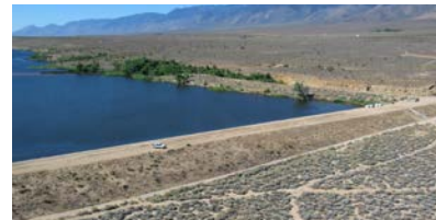
North Haiwee Dam No. 2 Inyo County, CA
