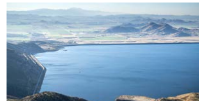
Diamond Valley Lake Engineering Design Winchester, CA
