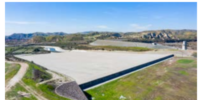
Prado Dam Spillway Raise Project Riverside County, CA
