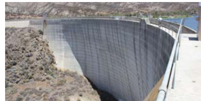
Vail Dam Seismic and Hydrologic Deficiency Evaluation Riverside, CA
