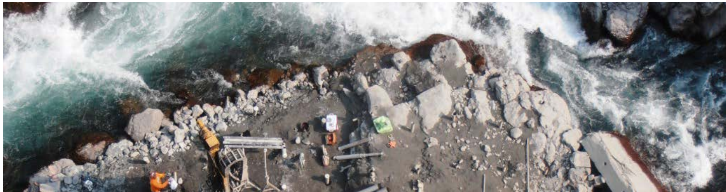
Elwha and Glines Canyon Dam Removal, Port Angeles, WA
