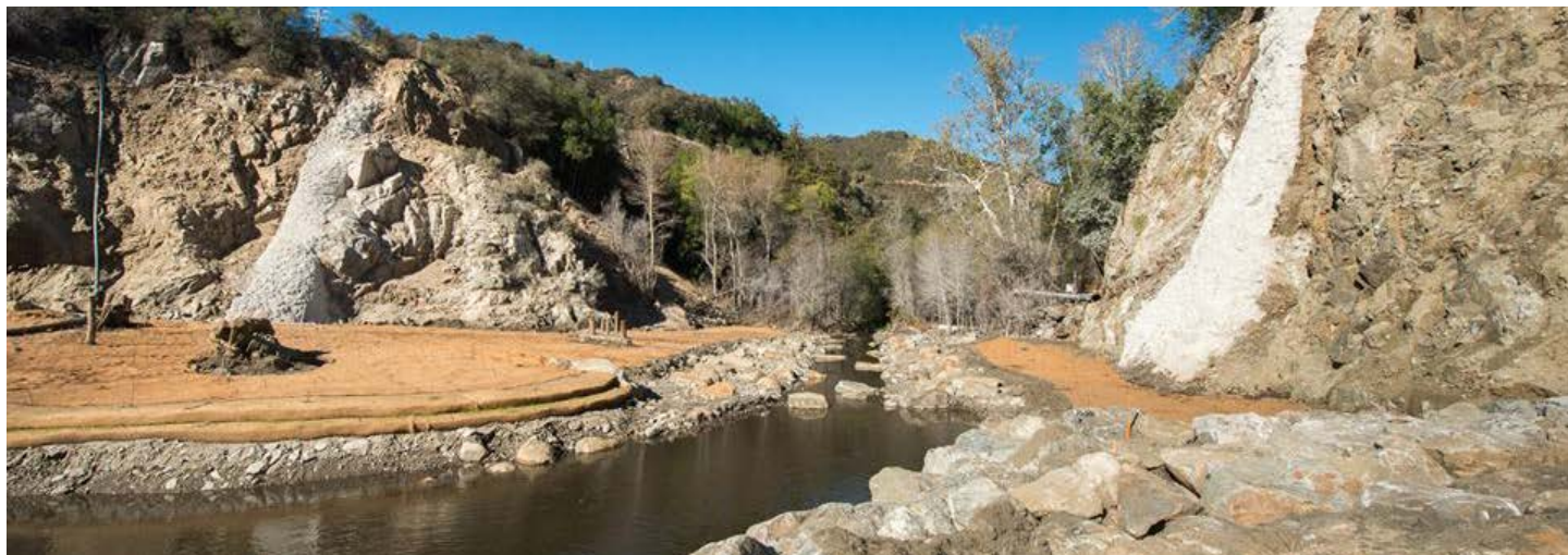
Carmel River Reroute and San Clemente Dam Removal, Monterey County, CA
