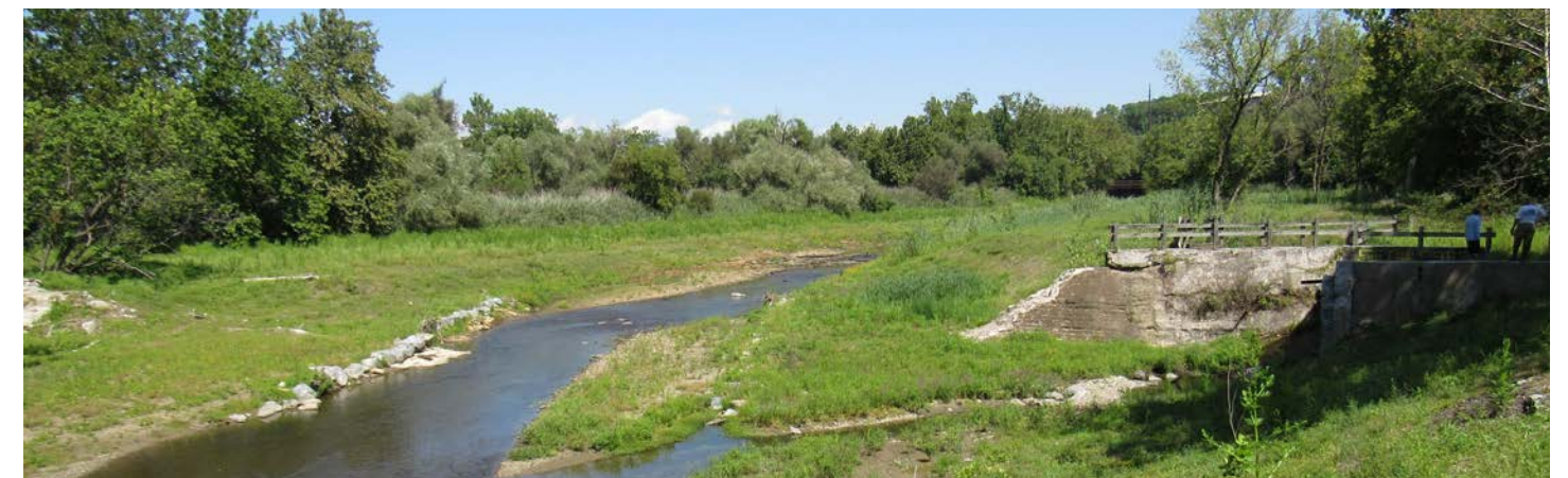
Elwha and Glines Canyon Dam Removal, Port Angeles, WA (After)
