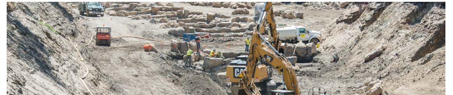
Carmel River Reroute and San Clemente Dam Removal, Monterey County, CA
