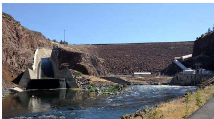
Iron Gate Dam and Spillway
