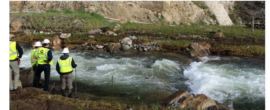
Carmel River Reroute and San Clemente Dam Removal – Channel Inspections, Monterey County, CA
