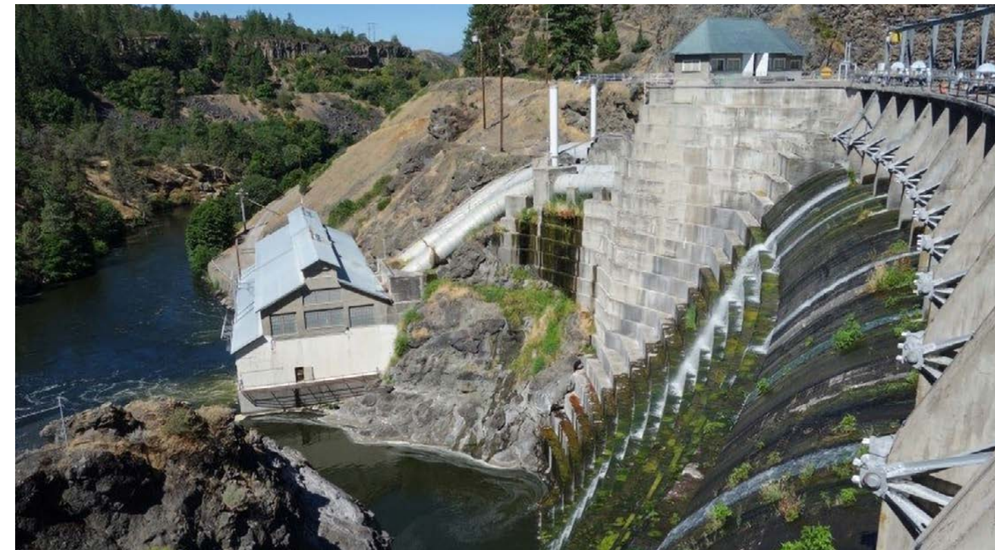
Copco No. 1 Dam
