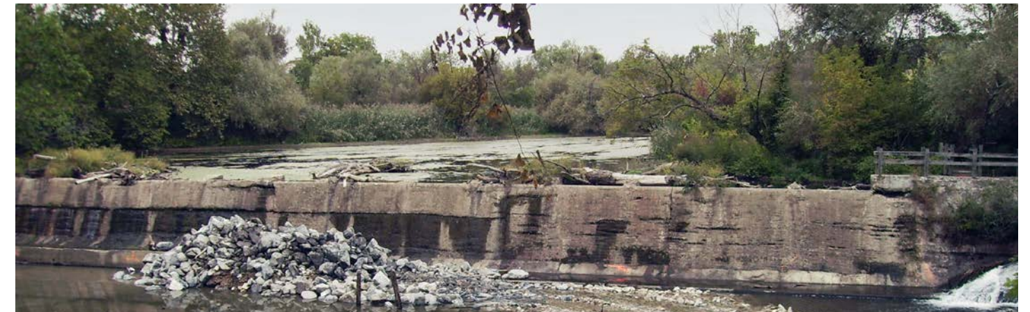
Elwha and Glines Canyon Dam Removal, Port Angeles, WA (Before)
