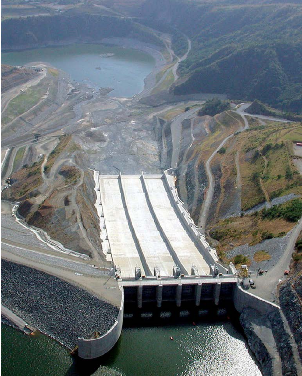
Left and above: San Roque Dam Luzon, Philippines Under an Engineering, Procurement, Construction (EPC) contract AECOM designed and built one of the largest hydroelectric, flood-control and irrigation projects in Asian history. Its major feature is a 650-foot-high rock-fill dam with a concrete chute spillway. The project reduces flooding, provides irrigation to more than 200,000 acres of land, and supplies clean hydroelectric power for commercial and industrial use to a region that desperately needs it. The spillway design required accommodating the Probable Maximum Flood (PMF) of 452,000 cfs.
