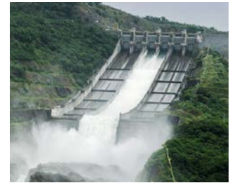
Left and above: San Roque Dam Luzon, Philippines Under an Engineering, Procurement, Construction (EPC) contract AECOM designed and built one of the largest hydroelectric, flood-control and irrigation projects in Asian history. Its major feature is a 650-foot-high rock-fill dam with a concrete chute spillway. The project reduces flooding, provides irrigation to more than 200,000 acres of land, and supplies clean hydroelectric power for commercial and industrial use to a region that desperately needs it. The spillway design required accommodating the Probable Maximum Flood (PMF) of 452,000 cfs.
