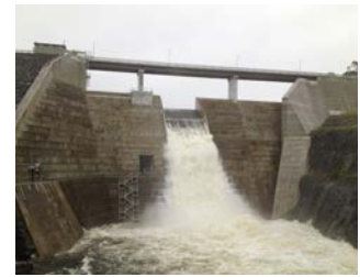
Left and above: Hinze Dam Queensland, Australia Raising the Hinze Dam for additional water storage was a key component of the Gold Coast Waterfuture Strategy. The risk-informed upgrade design raised the dam embankment 50 feet, from 310 feet above sea level, to 360 feet and extended the saddle of the dam by 2,600 feet. The complex foundation conditions at the right abutment required treatment that included the construction of a plastic concrete barrier wall to depths of up to 165 feet.
