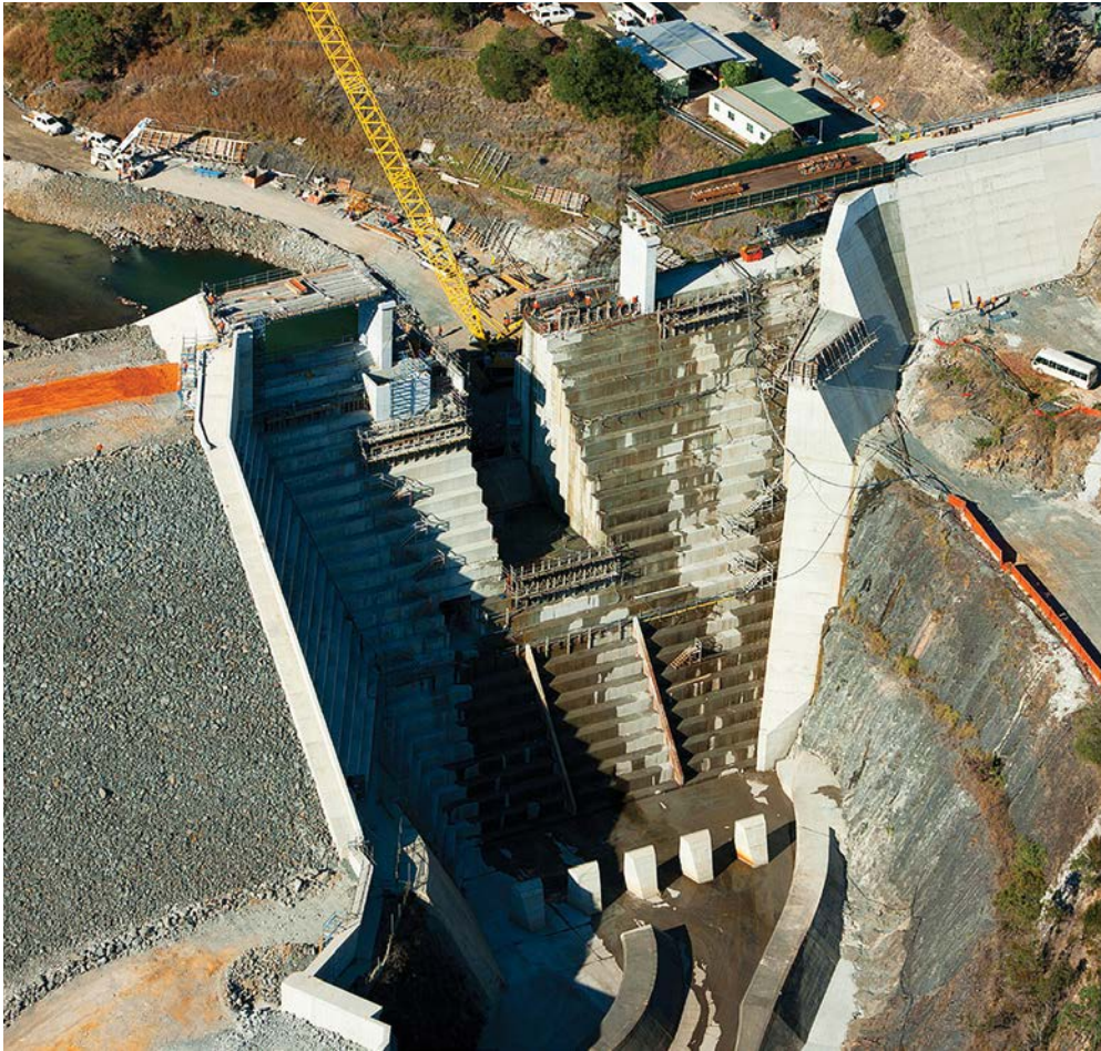
Left and above: Hinze Dam Queensland, Australia Raising the Hinze Dam for additional water storage was a key component of the Gold Coast Waterfuture Strategy. The risk-informed upgrade design raised the dam embankment 50 feet, from 310 feet above sea level, to 360 feet and extended the saddle of the dam by 2,600 feet. The complex foundation conditions at the right abutment required treatment that included the construction of a plastic concrete barrier wall to depths of up to 165 feet.
