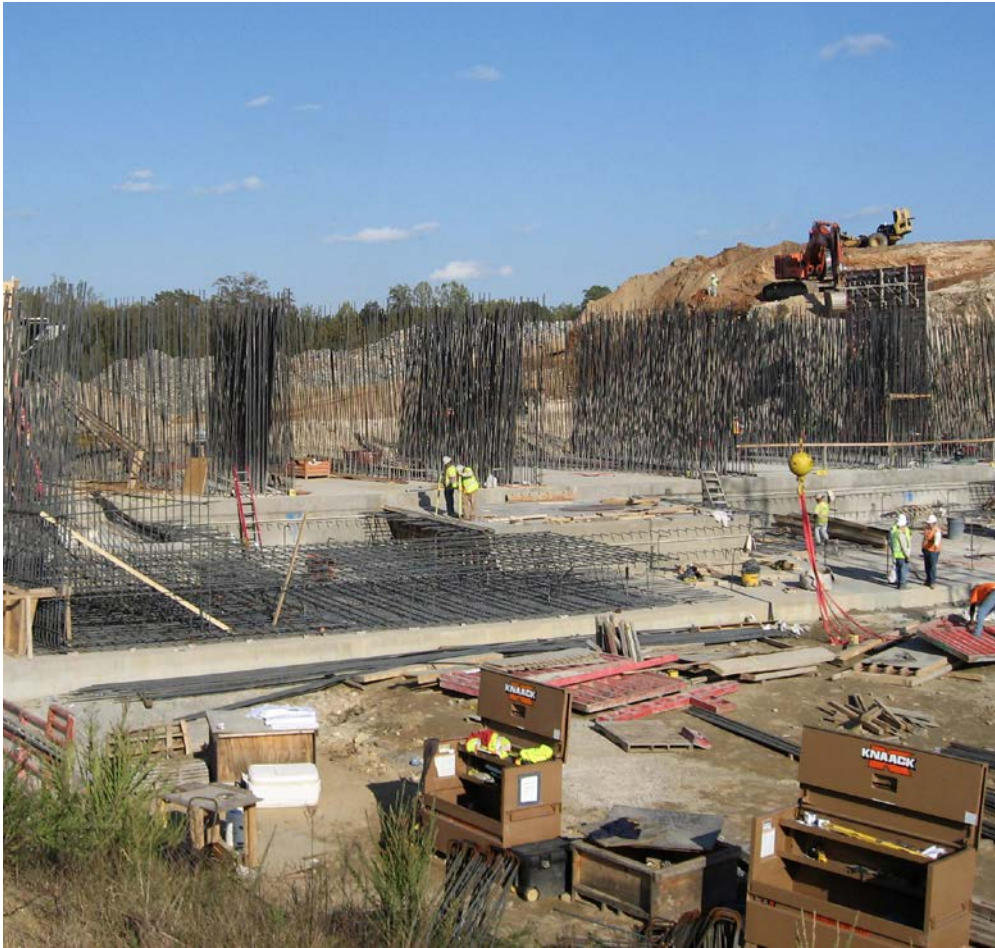
Left and above: Rocky Pen Run Reservoir Stafford County, Virginia, USA We provided engineering and construction services for the design of the Rocky Pen Run Reservoir project. The project consists of a 5.3-billion-gallon, pumped-storage, raw water supply reservoir and pump station adjacent to the Rappahannock River. Components include the main dam, spillway, outlet works, saddle dike, pump station, pipeline and access roads.
