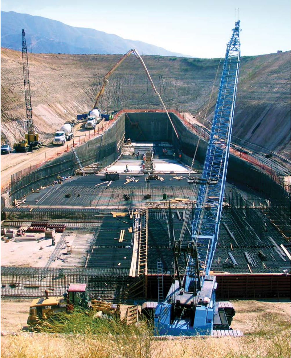
From left: Prado Dam, Gates and Control Tower Replacement Corona, California, U.S.A. AECOM provided services to the US Army Corps of Engineers to raise the dam by 65 feet, and to replace the gates and control tower at the Prado Dam. The improved storage and release capacities of the dam that were achieved through this project enable the dam to take full advantage of the improved channel capacity downstream. They also greatly increased the level of flood protection to the communities of Orange County in the Santa Ana River floodplain.
