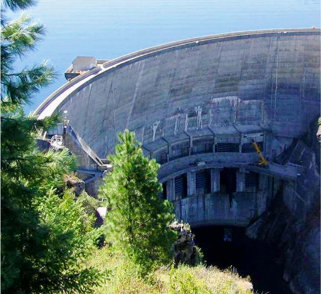
Boundary Hydroelectric Relicensing Project Washington, U.S.A. Boundary Dam, located on the Pend Orielle River in Washington is Seattle City Light's (SCL) major hydroelectric power generating resource. The scheme includes a 104-meter high variable radius concrete arch dam, with two service spillways, seven low-level sluices through the dam, and a power house with six turbines, with a total installed generating capacity of 1,070 MW.
