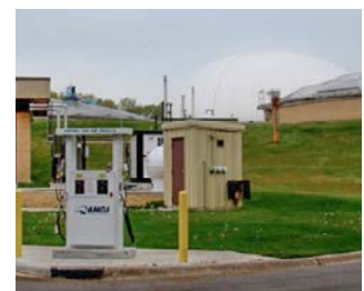
Digester Gas Utilization Janesville, Wisconsin, USA
