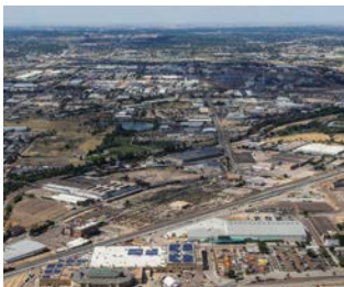
National Western Center Integrated Campus Energy Systems Denver, Colorado, USA
