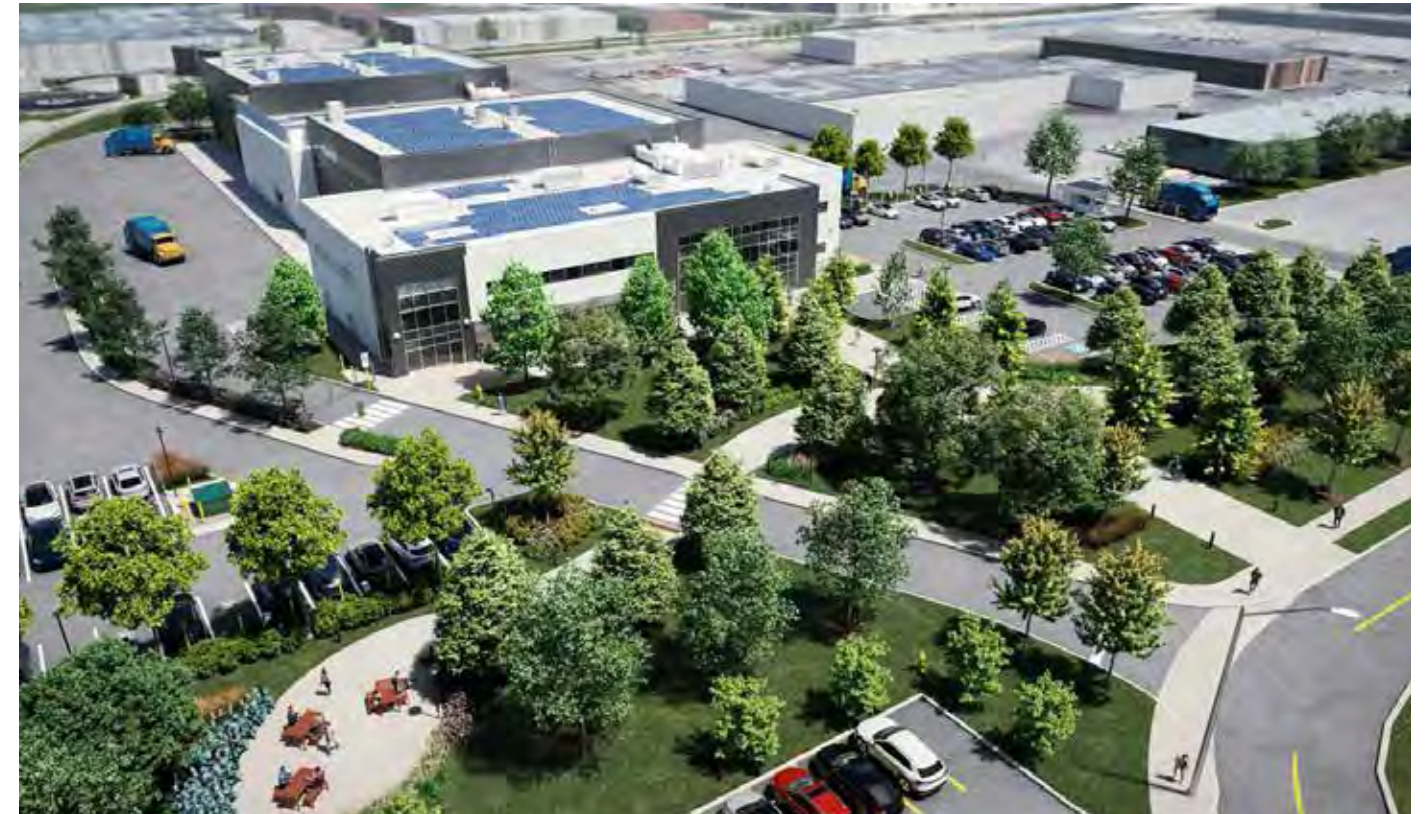
The design of the Ellesmere FMF building and its exterior environments incorporates several measures to improve sustainability and mitigate environmental impacts. To achieve net zero status, insulation, air tightness and triple glazing were used in the architectural design.
