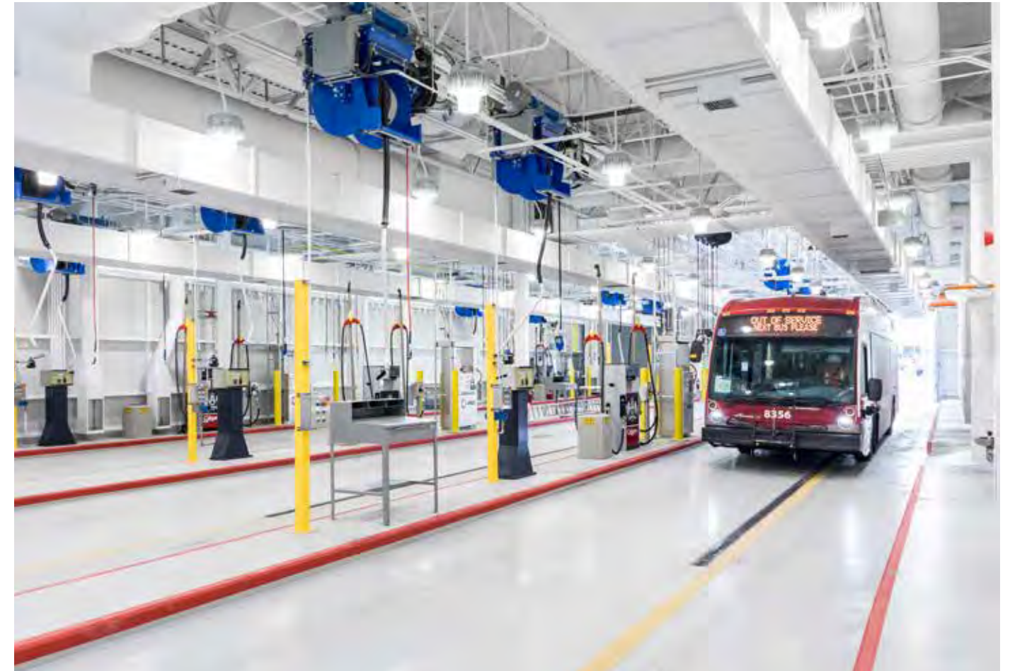
6 service lanes designed to complete fuel and daily service
