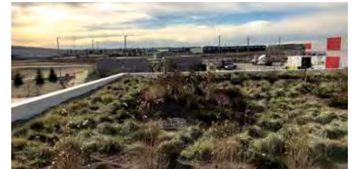
Green Roof Area
