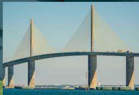
Sunshine Skyway Bridge Tampa, FL
