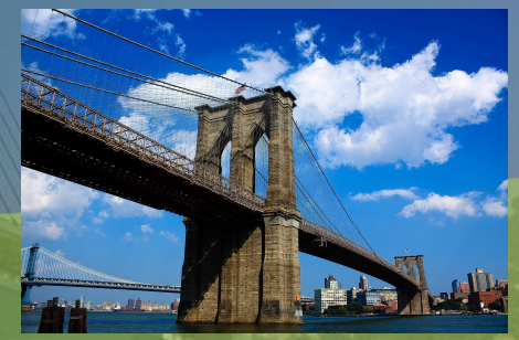
Brooklyn Bridge New York City, NY
