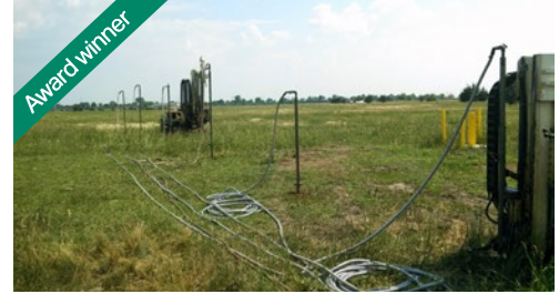
Cornhusker Army Ammunition Plant (Sub) Designed large system to pump and treat explosives-contaminated groundwater at EPA Superfund site; performed long-term monitoring
