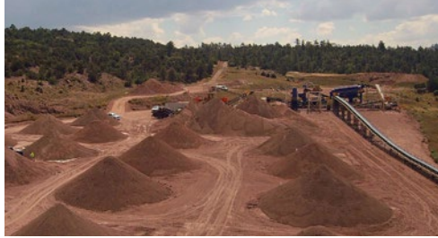
Fort Wingate Military Munitions Response Program (MMRP) Removal Action Removed and disposed of up to 500,000 cubic yards (cy) of UXO-contaminated soil
