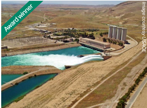
Mosul Dam Rehabilitation (Iraq) A/E services in support of USACE Engineer of Record during rehab focused on foundation grouting and repair of bottom outlets
