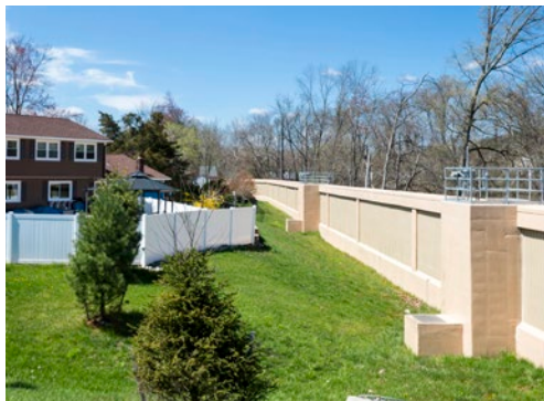
Green Brook Flood Risk Management - JV (NJ) Fast-track design of more than $20M in construction to meet ARRA funding requirements
