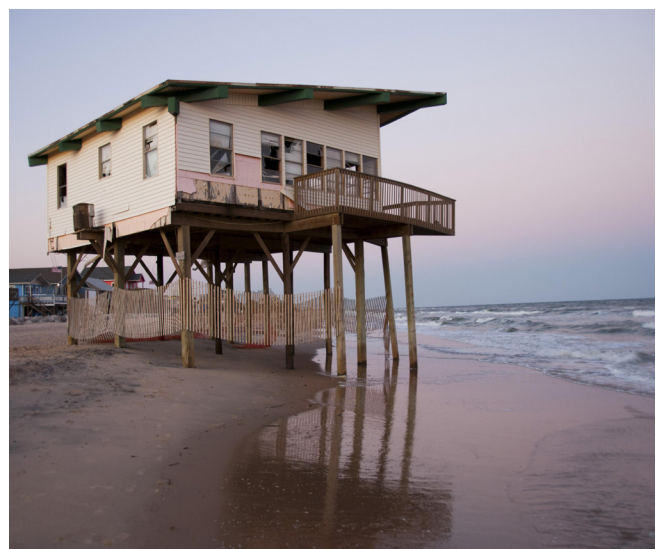
An endangered house in wait of advancing sea level and coastal storms along the Gulf Coast near Freeport, TX.
