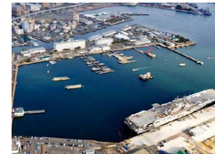
Juliet Pier Shore Power Upgrades for US Navy CFA Japan
