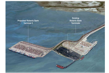
Roberts Bank Terminal 2 Vancouver, Canada
