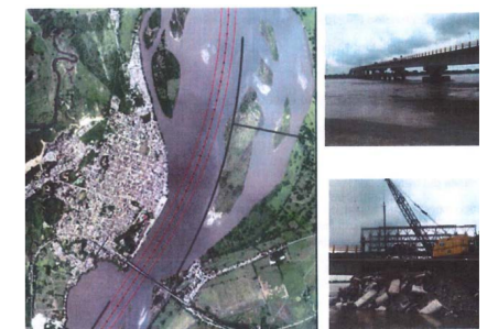
Detailed designs of the infrastructure/works for the recovery of the Navigability of the Magdalena River Colombia
