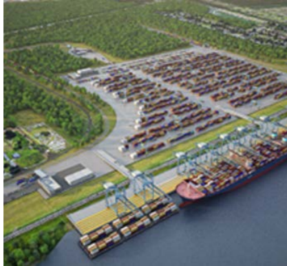
Louisiana International Container Terminal, USA
