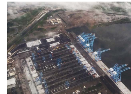
APMT Container Terminal – TEC II using an EPC FIDIC Yellow Book Contract Mexico
