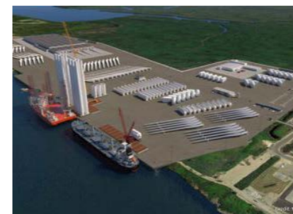
New Jersey Wind Terminal New Jersey, NJ
