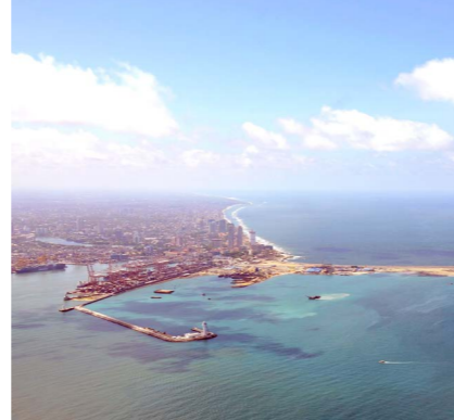
Colombo South Container Terminal, Colombo, Sri Lanka
