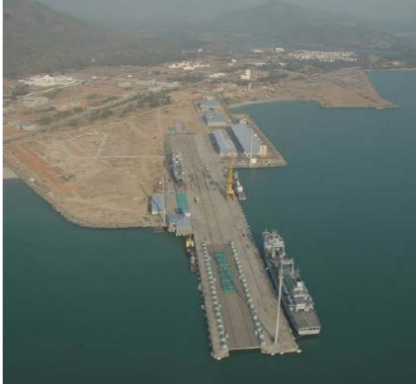
Project Seabird Marine Works and PMC Services for Indian Navy, Karwar, India
