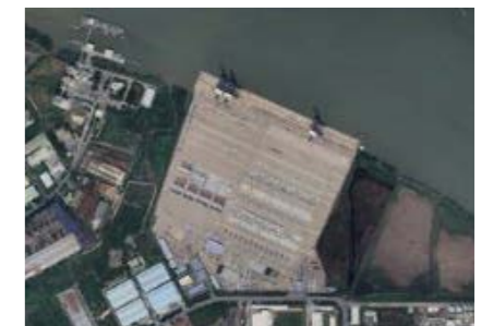
Saigon Premier Container Terminal – DP World Vietnam
