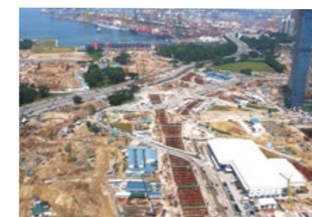
Singapore Downtown Line Cut-and-cover stations, Singapore
