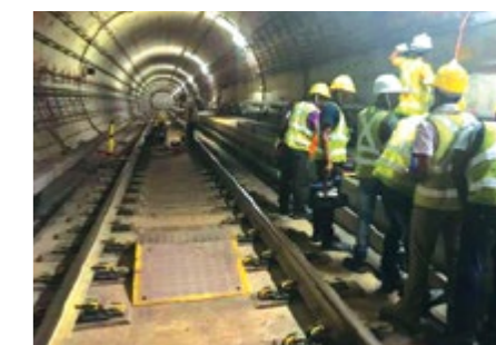
Singapore MRT Thomson Line C2104 Tunnels and station, Singapore
