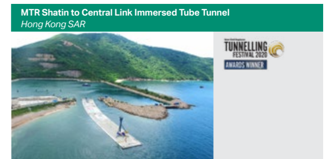
MTR Shatin to Central Link Immersed Tube Tunnel Hong Kong SAR 1.7-km-long railway immersed tube tunnel
