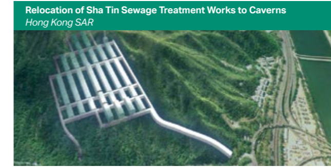
Relocation of Sha Tin Sewage Treatment Works to Caverns Hong Kong SAR Sustainable use of underground space – New Civil Engineer Award 2015
