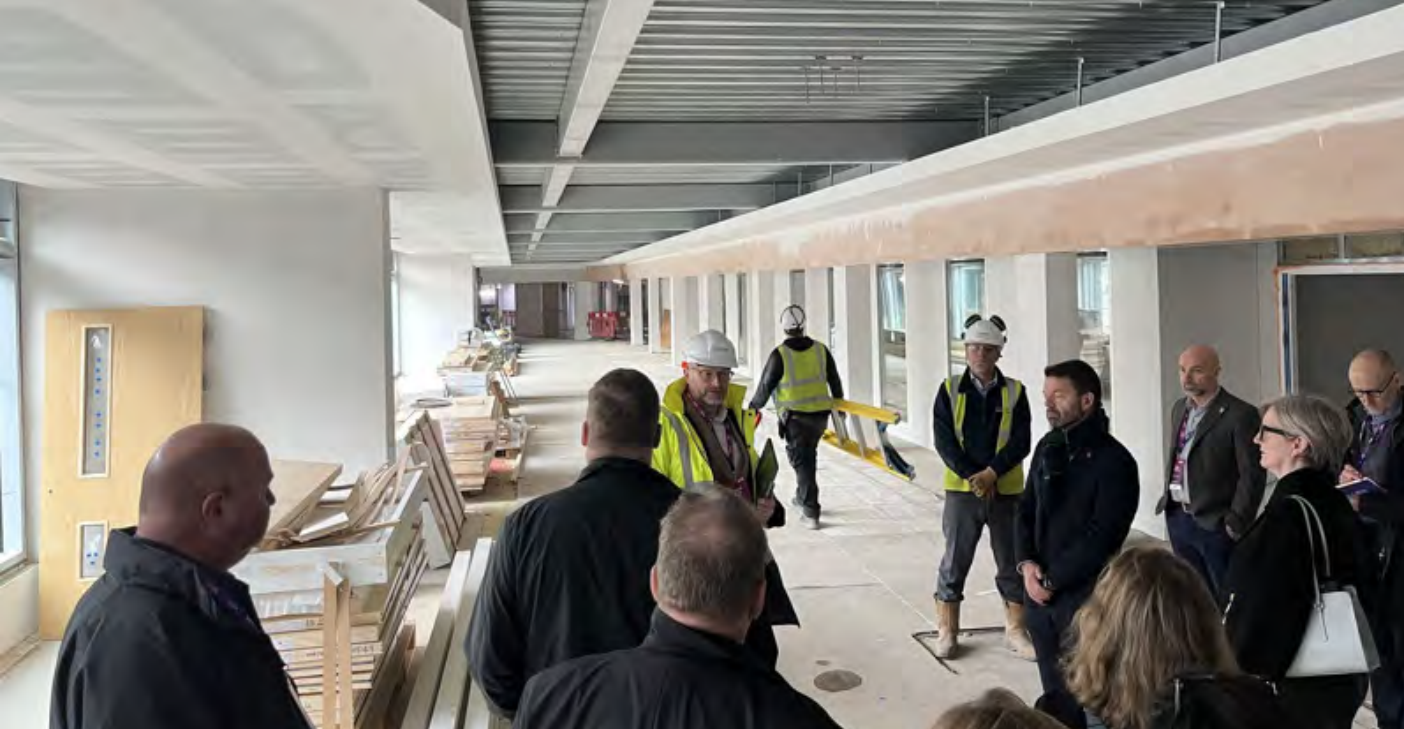
Lancaster University Management School - East Pavilion
