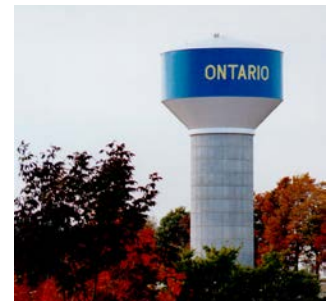
Mabee Road 1 MG/3.8ML Elevated Storage Tank
