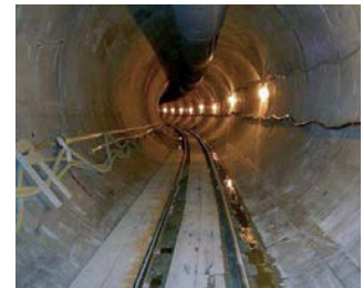
From top: Deep Rock Tunnel Connector and Dewatering Pump Station Indianapolis, Indiana, USA To reduce sewage overflows, design and construction management services were performed for this 7.6-mile/12.2-km-long, 18-foot/5.5-meter-diameter tunnel. North Dorchester Bay CSO Tunnel Boston, Massachusetts, USA The 17-foot/5.2-meter-diameter tunnel was constructed between 40 and 60 feet/12.2 and 18.3 meters deep in soft earth.
