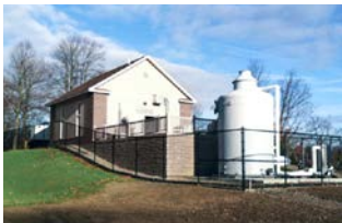
Watchemoket Pump Station from 3D Design to Operation East Providence, Rhode Island, USA We provided 3D modeling and design services for the 10-MGD/3.8-ML/d pump station.
