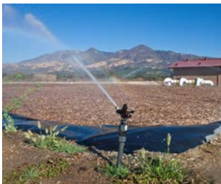
Fillmore Water Recycling Plant Fillmore, California, USA AECOM provided construction and program management services and was the owner's representative for the state-of-the-art water recycling plant (WRP) under a design-build-operate approach. The $43 million WRP used membrane bioreactor wastewater treatment technology to meet the City of Fillmore's water quality and environmental improvement goals.
