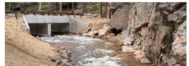
James Creek Flood Reduction, Boulder County, CO
