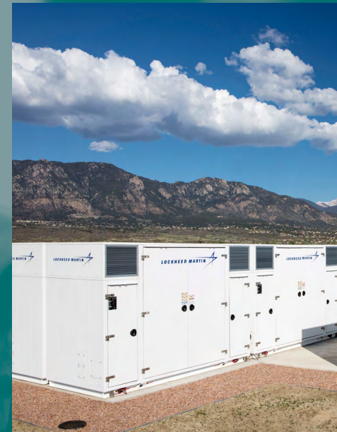
Fort Carson, U.S. Army Training Facility, ESPC
