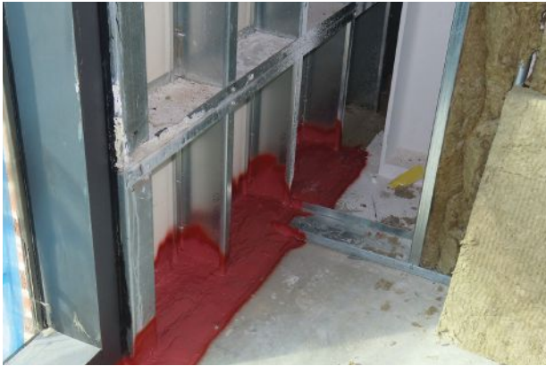
Example of CFMF slab edge detailing and sequencing and coordination of installation. Zussman Photo.
