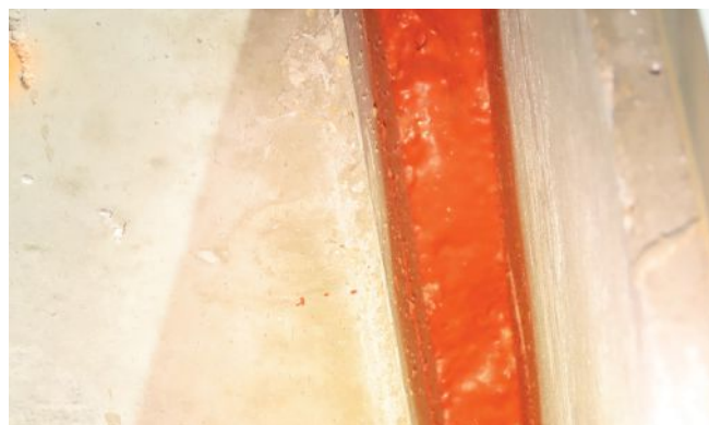
Example of underside edge of slab fire stopping installation due to sequencing and coordination. Zussman Photo.
