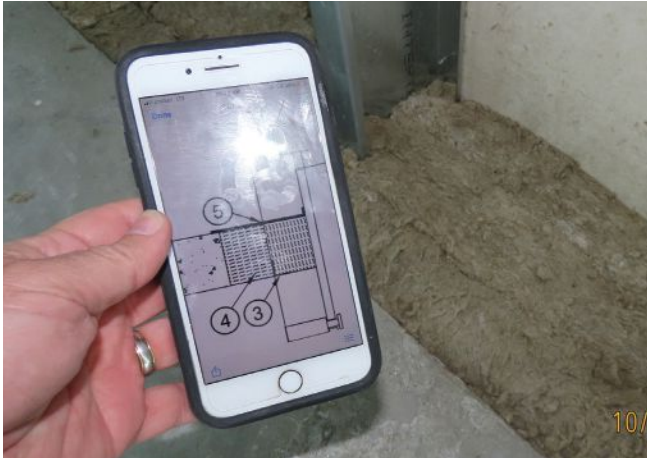
Example of a first work-in-place inspection of the mineral wool. Zussman Photo.
