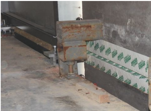
Coordination of attachment of dead load clip at precast and curtainwall to raise the support for better access of the slab edge fire joint. Zussman Photo.
