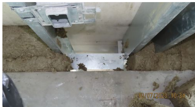
Example of mineral wool support at CFMF due to slab edge gap size. Zussman Photo.
