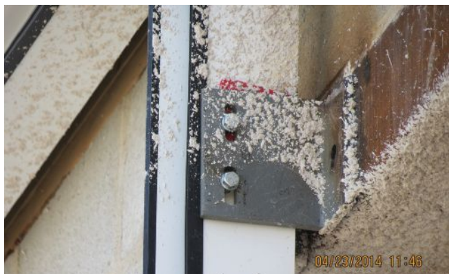
Example of a wind connection of the curtainwall system. Zussman Photo.
