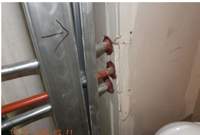
Fire-rated penetration at a fire-rated room perimeter wall. Corey Zussman photo
