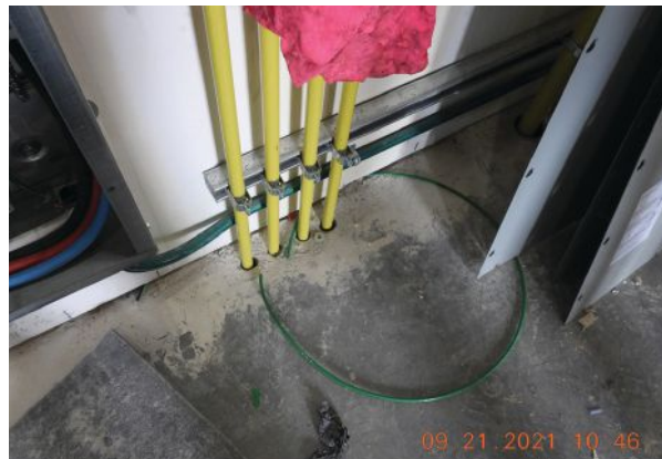
T-rated firestopping needed, which will need a large core through the floor. Corey Zussman Photo
