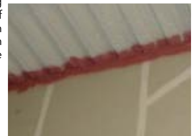
Spray fireproofing (SFRM) on deck. Fire Stop Technologies Photo
