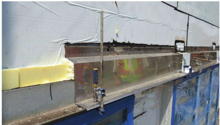
Creating a continuous air barrier from the wall to the shelf angle with a stainless steel flashing. The author also installed a spray polyurethane foam (SPF) solid under the stainless steel flashing to reduce the condensation potential under the flashing.
