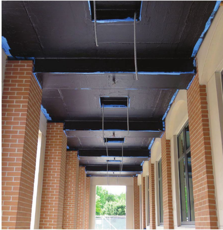
Upper soffit for the air barrier, including the electrical lightbox. A finish soffit will be installed under this soffit.
