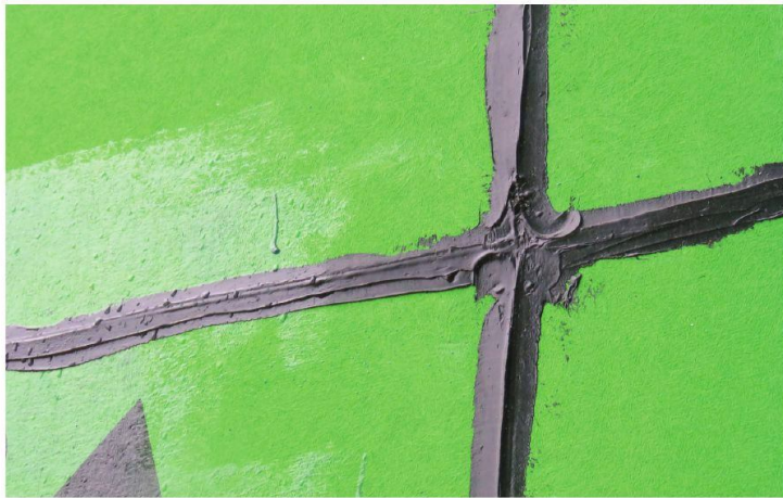
Proper sheathing joint detailing (approximately 3.2 mm [0.125 in.] thick by 25 mm [1 in.] wide approved joint material with proper water shedding slopes.
