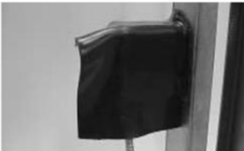
Step 3: Starting at top, align to front edge of box and overlap onto the stud 1/2 inch (13 mm).
