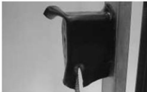
Step 4: Adhere remaining pad to box and cut to provide a snug fit around conduits or cables.
