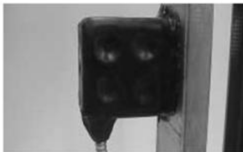
Step 6: Trim excess putty from corners and apply it to conduit fittings or cables connected to the box. Ensure pad is pressed firmly to surface of top, back, bottom, and side of box.
