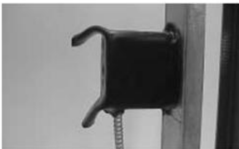
Step 5: Extra putty will pleat at corners after pad has been applied to surface of box.
