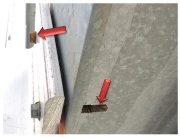
Fasteners rated for exterior exposure will be "CORROSION RESISTANT". The fastener should have a salt spray test of over 500 hours per ASTM B117 or have less than 15% surface rust after 15 cycles of salt exposure via the Kesternich Test per FM Global.
