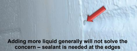
Installing the manufacturer's sealant over the joint between the peel and stick membrane and the liquid AVB will close off the openings that will likely exist at the CMU joints.
