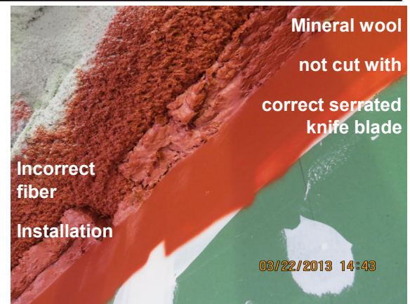
Good example of a fire stopping and head-of-wall mock-up
