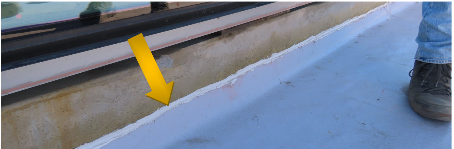
Proper end-of-day seal installed on the roofing membrane.
